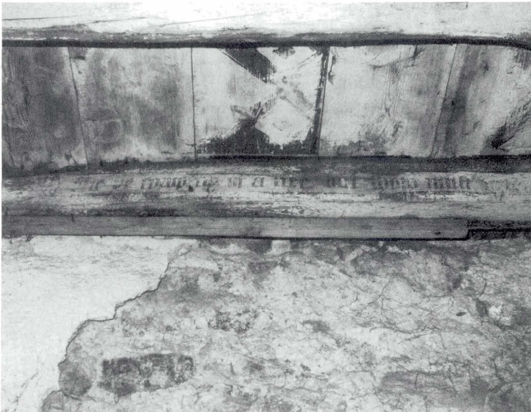
1. Lime plaster on the hard at Collairnie Castle Fife, probably late sixteenth century
