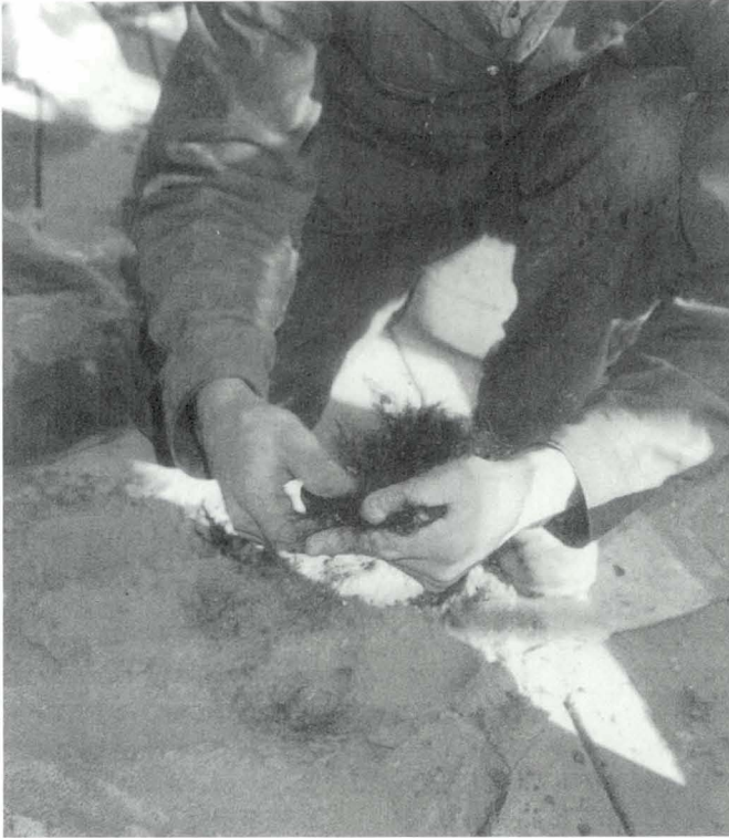
12. Teasing out hair, before mixing with coarse stuff
