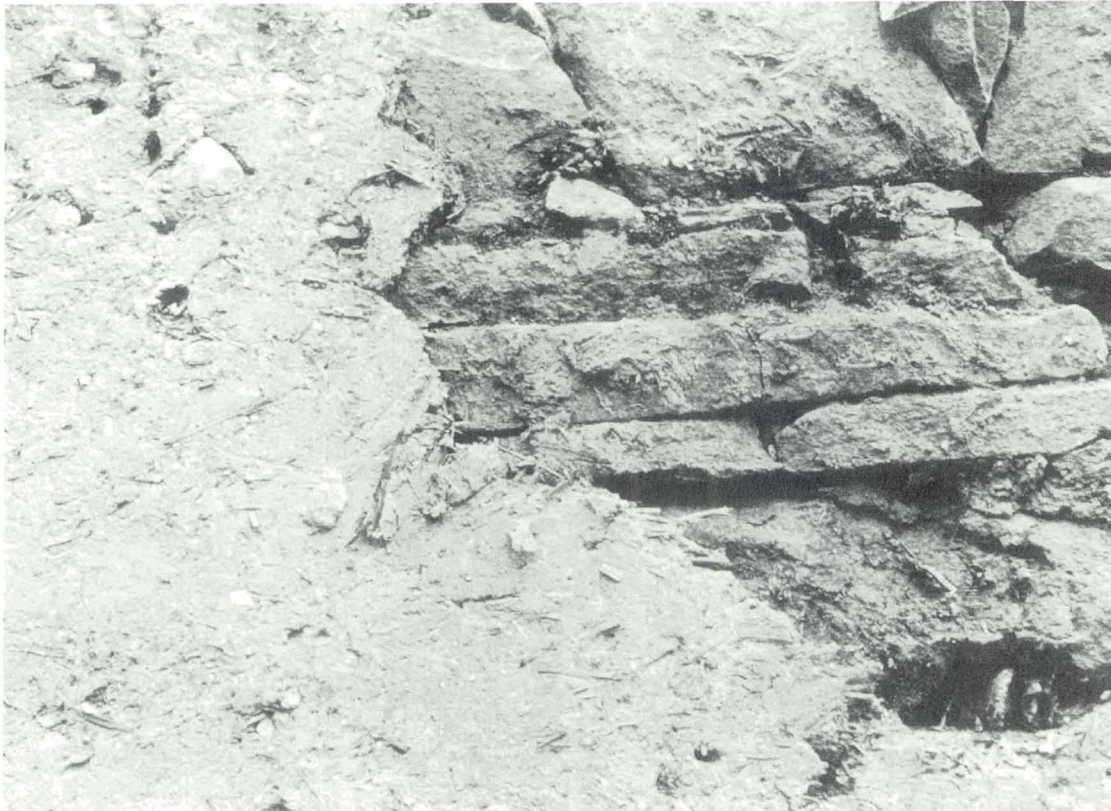
2. Clay plaster on the hard, from a group of four weavers' cottages known as Jericho, on the Angus and Glamis Estates, built by Firpark of Brigton, 1771-76
