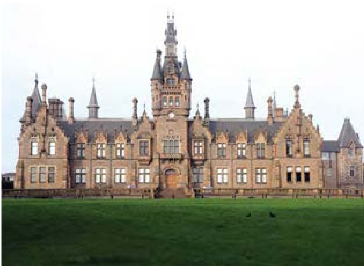
Illus 53 The category A listed Morgan Academy in Dundee was devastated by fire in 2001. The facade was subsequently reinstated with costs running into millions of pounds Top: © Crown Copyright: RCAHMS. Licensor www.rcahms.gov.uk and bottom: © Historic Scotland
