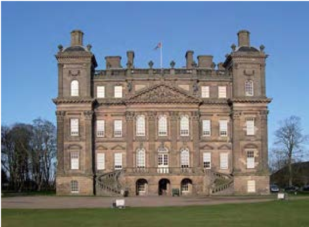
Illus 66 Duff House, Banff. To address the fire safety needs of this property during a conversion to an art gallery, sprinklers were sympathetically installed
