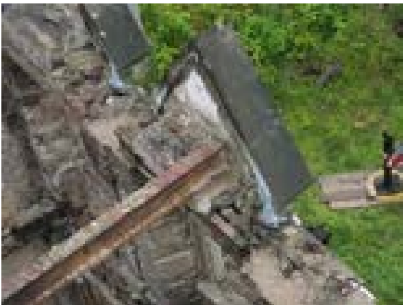
Illus 91 Broadstone House, wall head dormer detail
