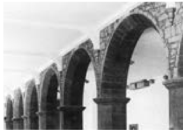
Illus 95 Sidewall sprinklers and exposed pipework in the Laigh Hall, High Courts, Edinburgh
