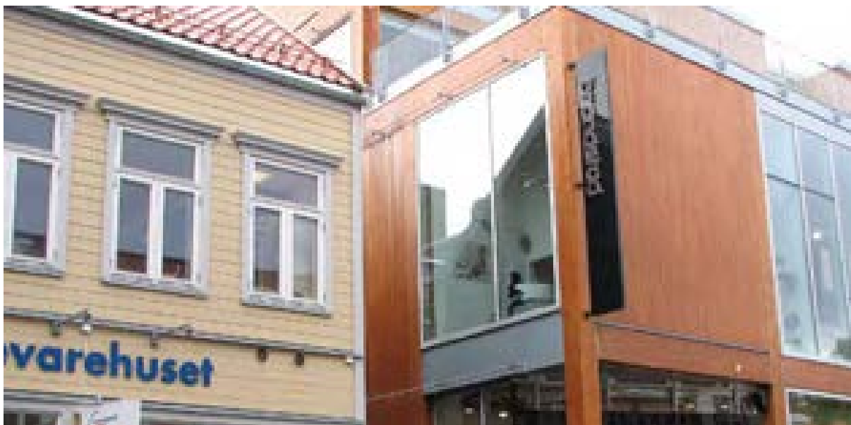
Illus 24 A Norwegian example where a drencher system has been installed to the exterior of the building on the right to prevent fire spread from or to the neighbouring timber building
