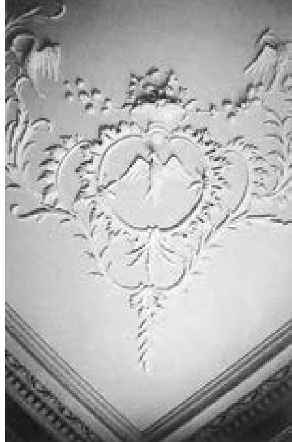
Illus 112 Installed concealed sprinkler head, the vestibule, Duff House
