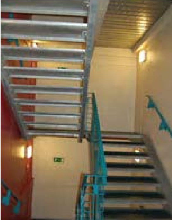
Illus 70 The new north staircase that was constructed to allow a direct fire exit route from the Reading Room and to provide a second stairway
