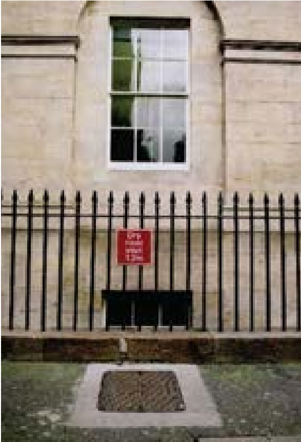
Illus 23 Historic fabric impact minimised by locating dry riser inlet valves beneath cast iron cover in footpath © Paul Beaton
