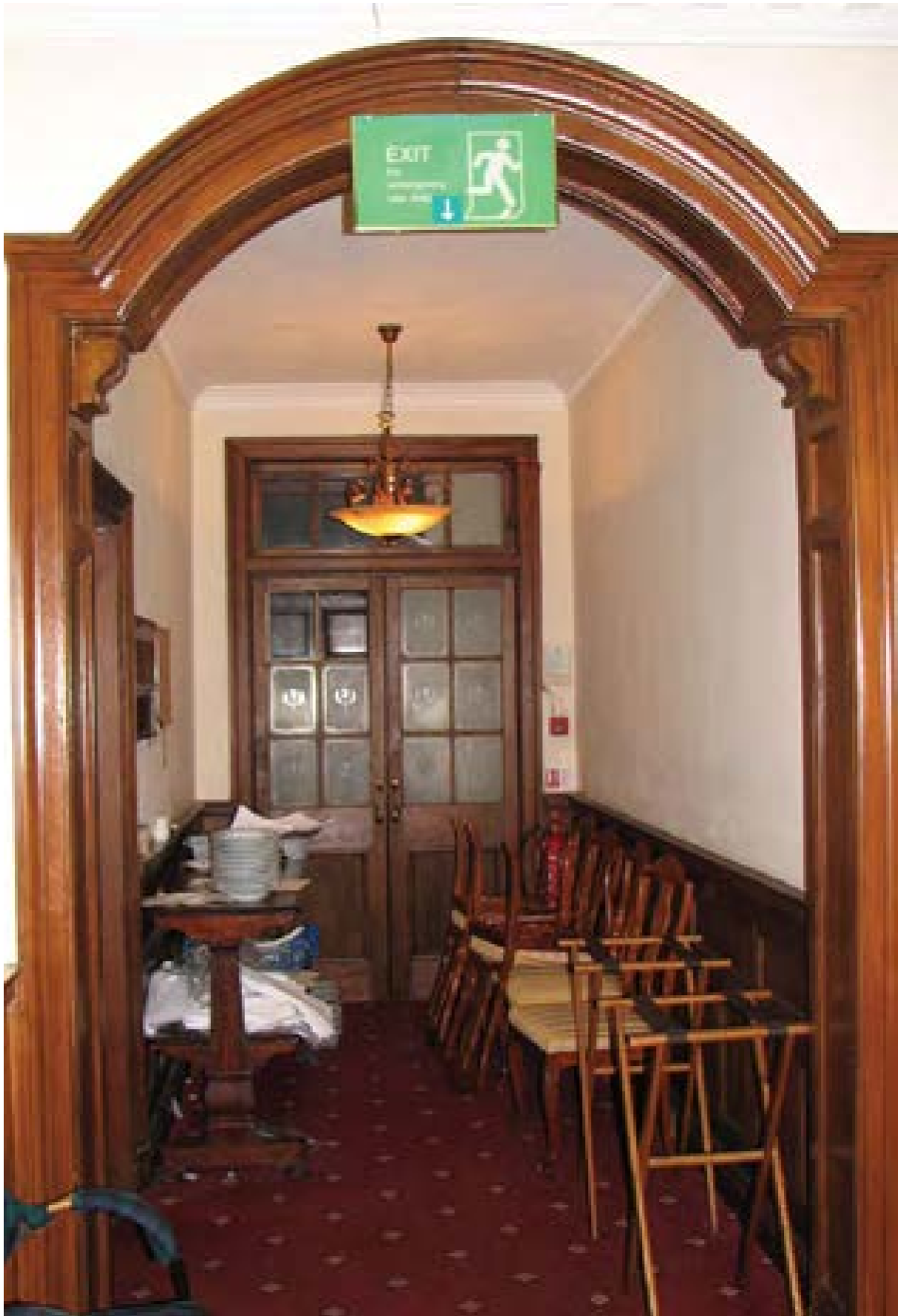
Illus 3 Sound management should ensure that hazards and risks are eliminated or reduced, so situations like blocked fire escapes are avoided
