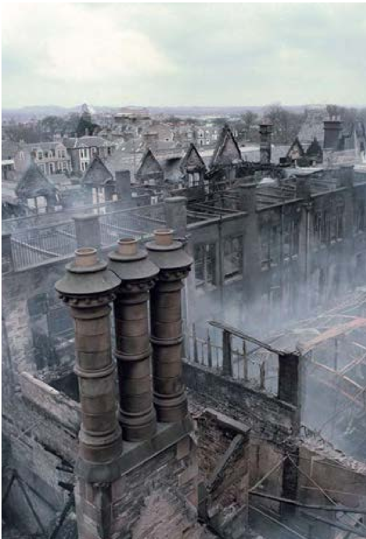
Illus 1 Morgan Academy, a category A listed school was gutted by fire in 2001 © Crown Copyright: RCAHMS. Licensor www.rcahms.gov.uk
