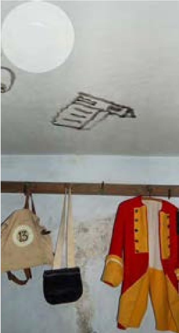
Illus 77 Concealed sprinklers do not distract from the original Jacobite graffiti on the ceiling of the former barracks room
