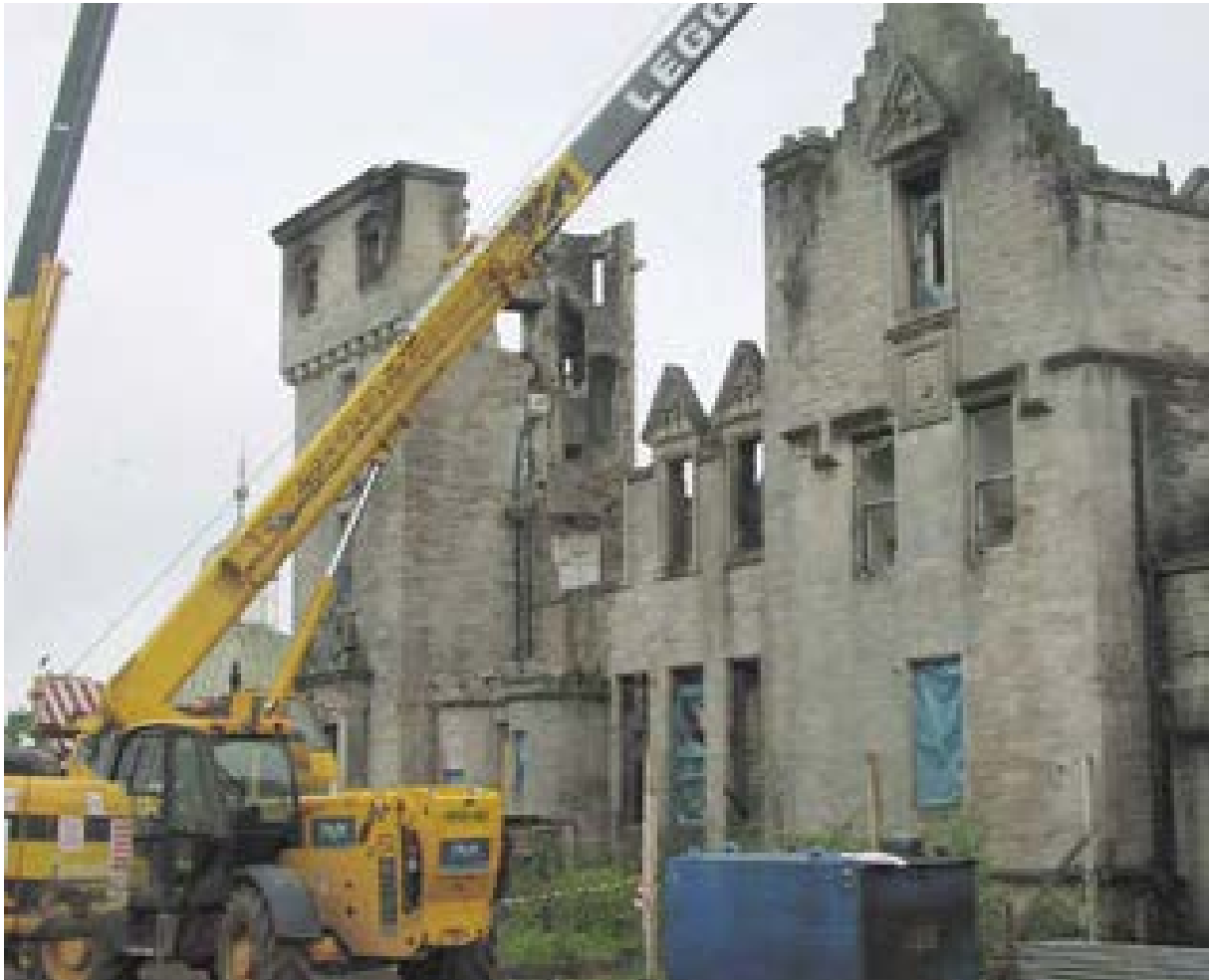
Illus 89 Broadstone House, Renfrewshire. Post-fire stabilisation works underway
