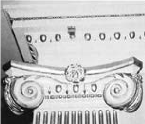
Illus 117 Sidewall sprinkler head installed within cornice
