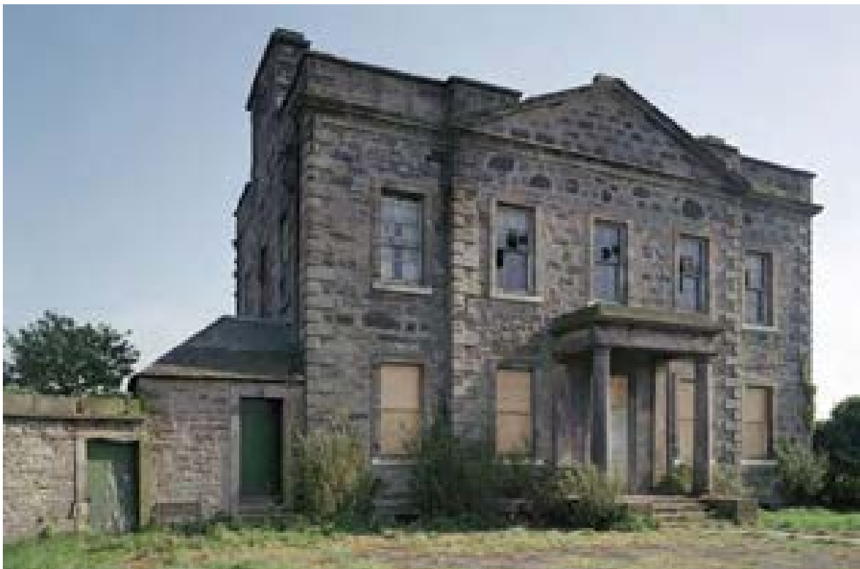
Illus 81 This A listed property lay derelict for many years, vulnerable to fire amongst other things
