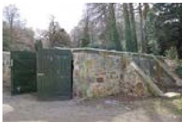
Illus 28 Sprinkler components such as water tanks, pumps and valve sets can sometimes be discreetly housed in outbuildings as here at Newhailes house (reproduced with kind permission of the National Trust for Scotland)
