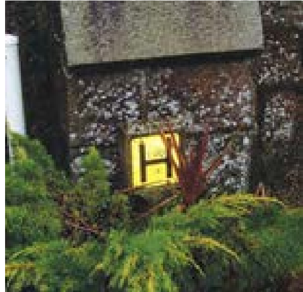
Illus 50 A hydrant marker that has become obscured by overgrown vegetation, a situation good management would address © Stewart Kidd
