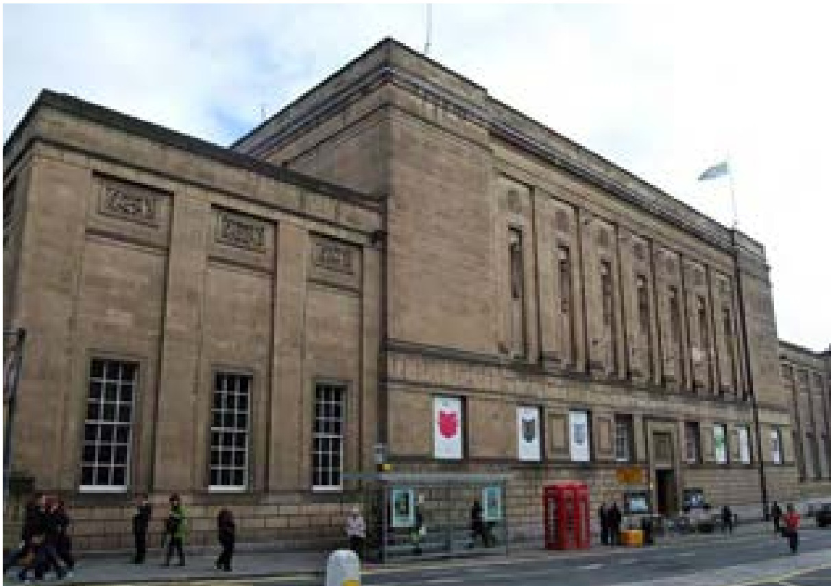
Illus 68 The National Library of Scotland installed a sprinkler system to compensate for deficiencies in the fire safety provisions in the property
