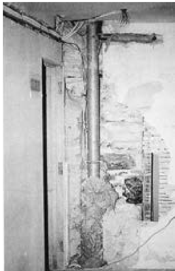
Illus 108 Vertical pipe installation
