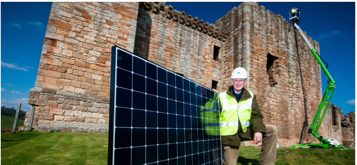
Replacement of solar panels at Crichton Castle, Midlothian
