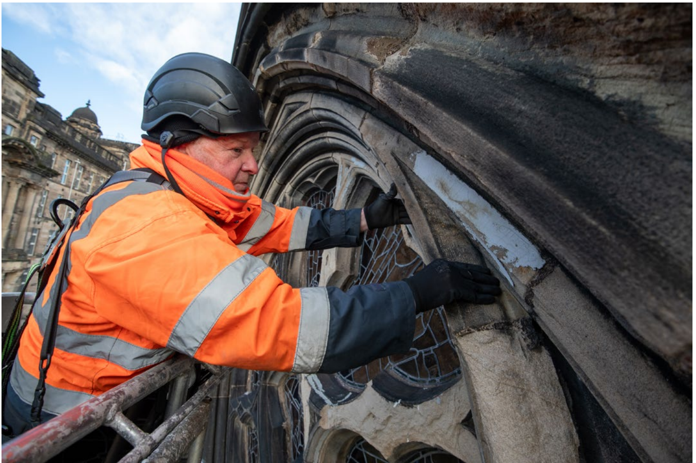
High-level masonry inspection survey at Glasgow Cathedral
