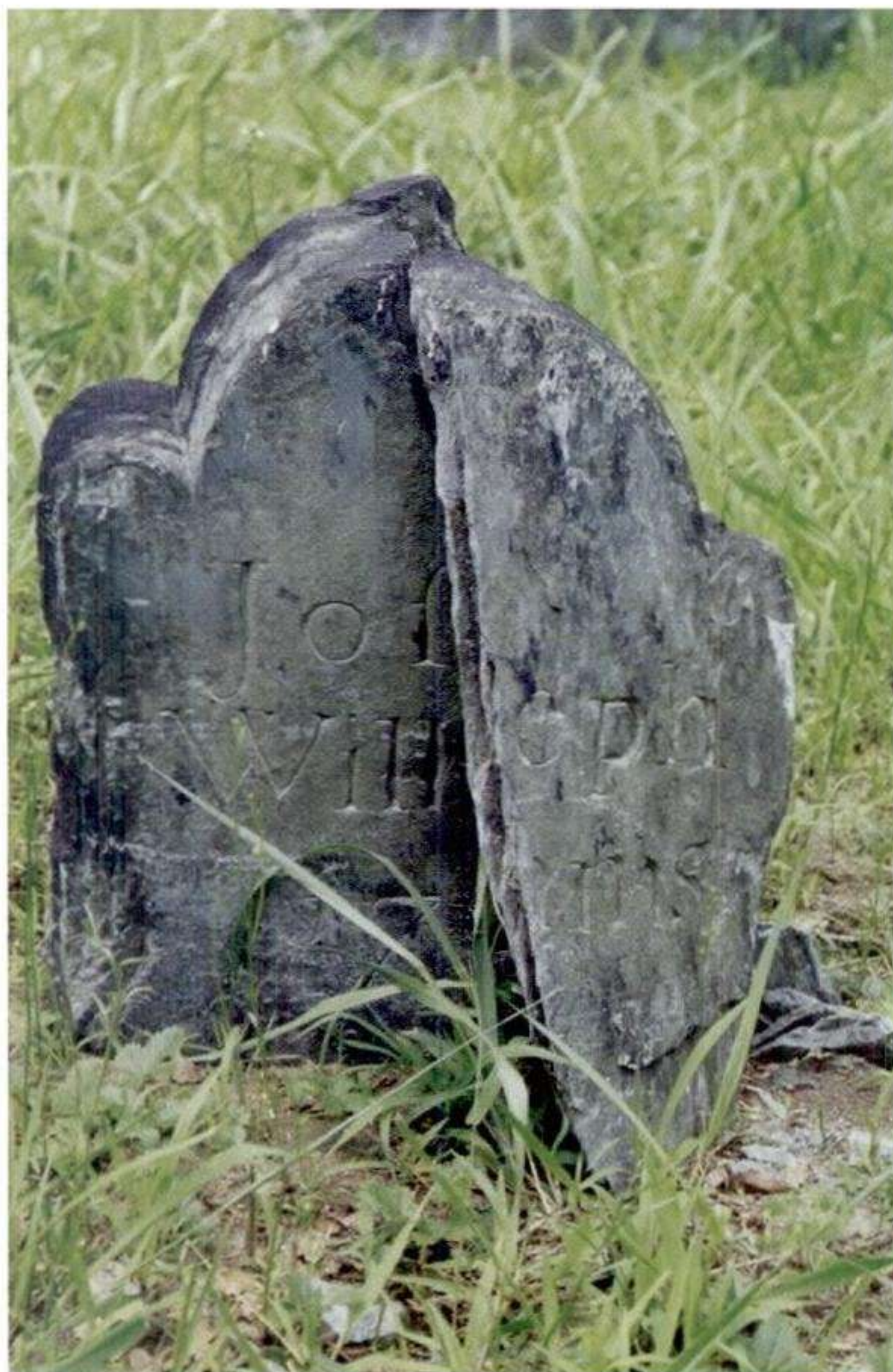
Illus 4 Case study: repair of a sunken and fractured direct-burial slate marker
