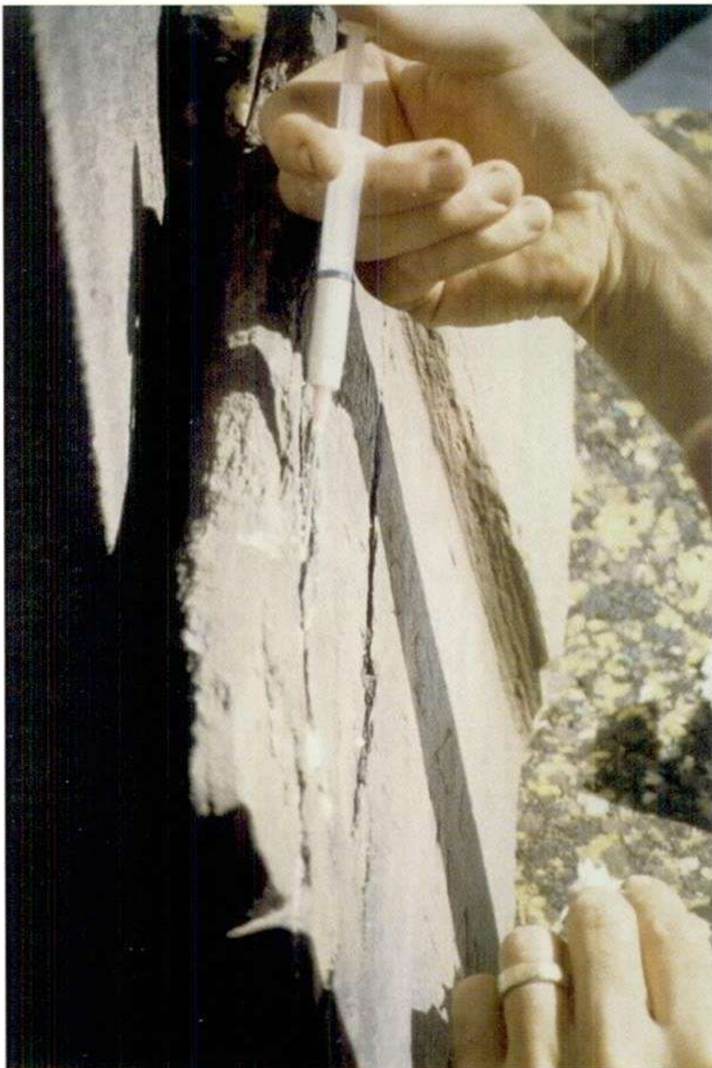
Illus 6 Injecting cracks in stone
