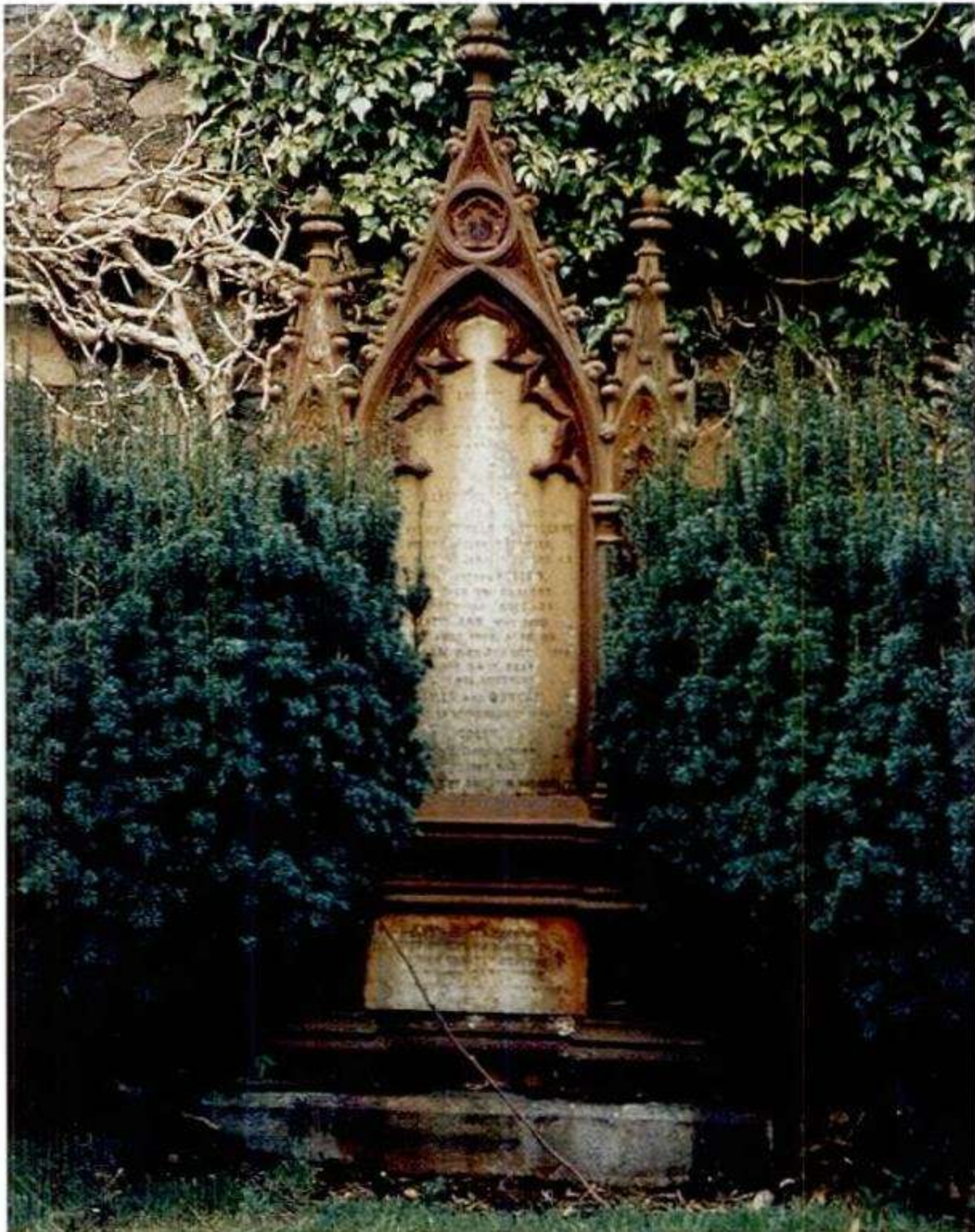
Illus 12 A cast-iron gravestone at Kilkerran Churchyard, Campbeltown, showing corrosion from exposure to the salty coastal air
