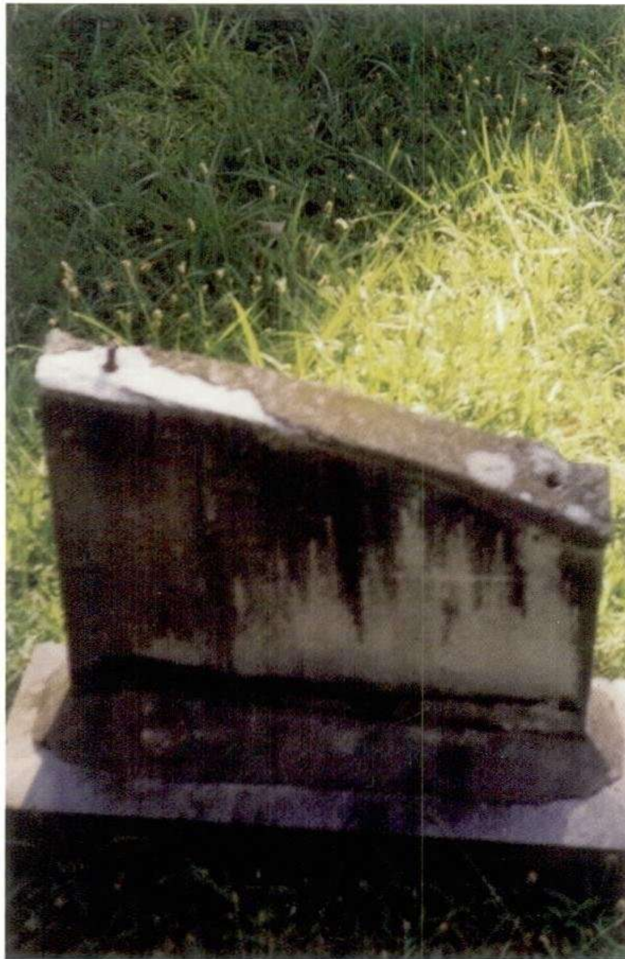
Illus 5 Case study: repair of a fractured marble stone on tilted granite base
