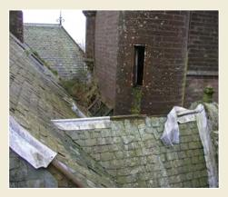
Fig. 6: Wind uplift on exposed leadwork can result in the lead coming off.
