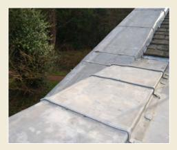
Fig. 5: Milled lead sheet used to cover a flat roof.
