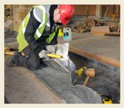
Fig. 10: Dressing in new lead sheet using traditional techniques and tools.
