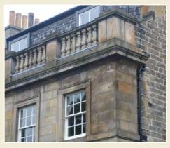
Fig. 7: A blocked lead parapet gutter is causing saturation of the masonry below.
