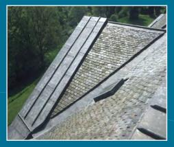
Fig. 1: Lead is used for both roof coverings, and to cover pediments, ridges and roof valleys.
