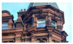
Fig 6 Different surface finishes on stone masonry attract differing degrees of soiling which adds depth and richness to the building.
