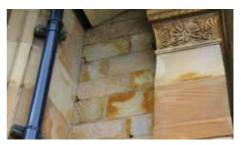
Fig 12 Surface damage, bleaching and iron staining to stone masonry caused by inappropriate and aggressive stone cleaning.
