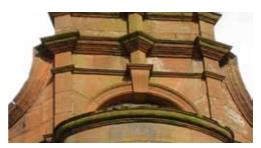
**Fig 20** Recently cleaned sandstone building showing relatively rapid recolonisation and biological soiling.
