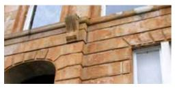
**Fig 17** Severely damaged stone façade following inappropriate cleaning, resulting in a loss of the external patination layer, discolouration from oxidation and increased deterioration.
