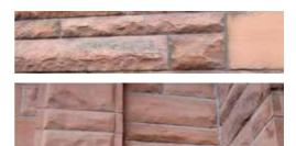
**Fig 19** Original soiled (top) and mechanically cleaned (disked) (bottom) rock-faced masonry showing destruction of the original sharp masonry finish to the cleaned stone.
