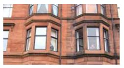
**Fig 13** The cleaning of a facade (left side of image) is often considered desirable yet does not necessarily dramatically improve the aesthetics of a building.
