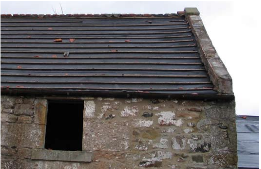
An exposed roof showing battens onto which pantiles are hung by their nibs
