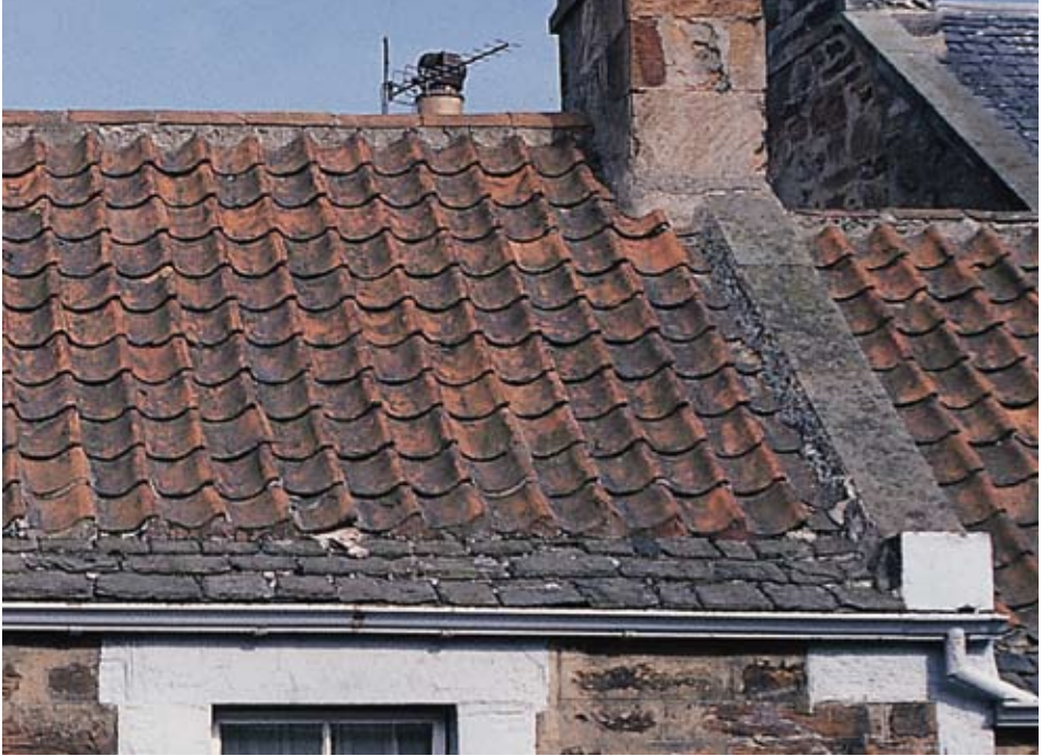
Pantiled roof showing slated easing course
