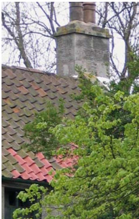
Replacement pantiles located in an unobtrusive area of the roof
