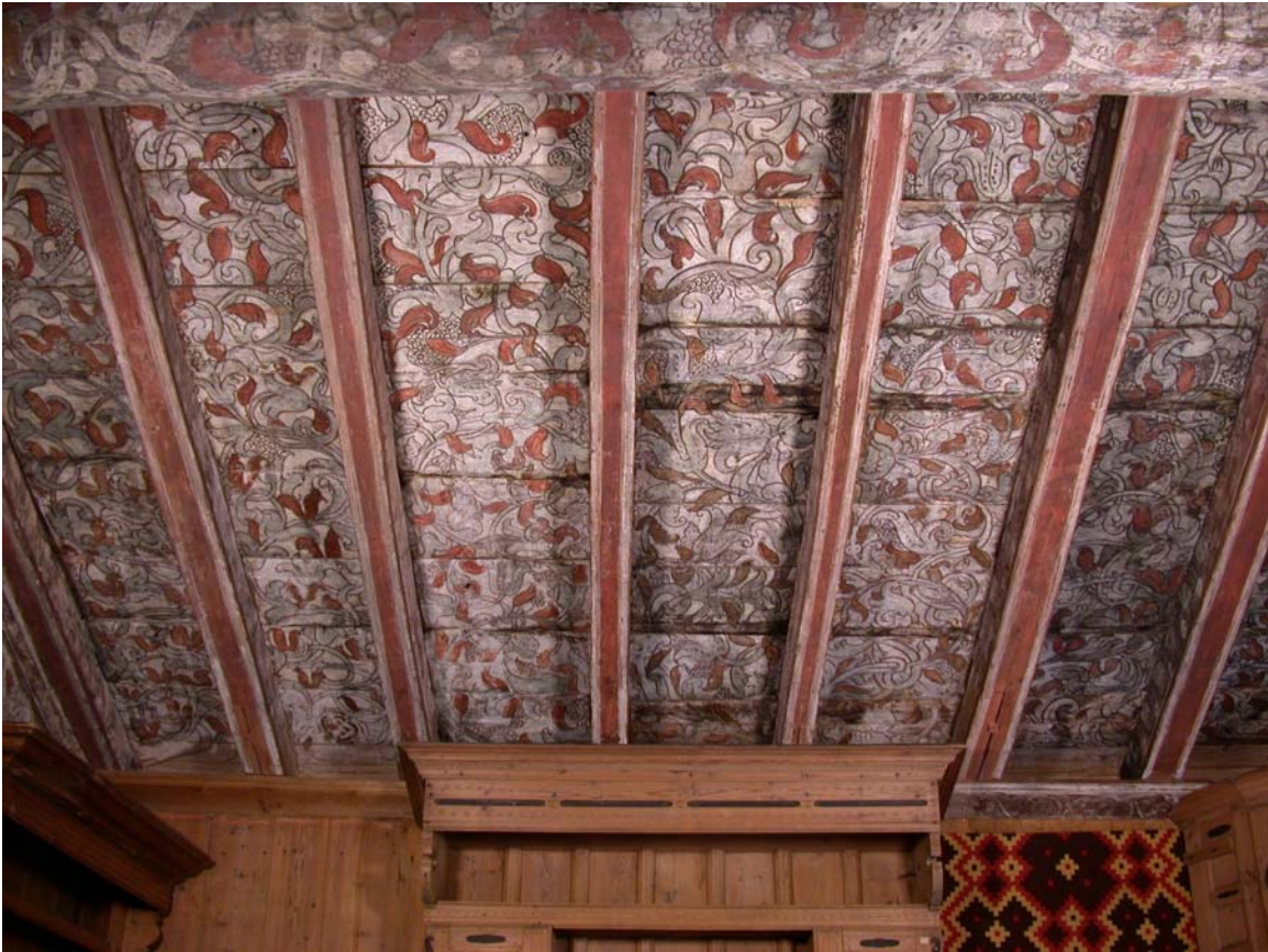
Illus. 5 Painted underside of a beam-and-board roof in a wooden Norwegian house © Norwegian Institute for Heritage Research, Oslo
