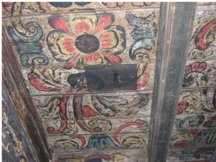
Illus. 2 Remaining show square of a discoloured creosote layer on the ceiling of a 19 th century guest house at the Norsk Folkemuseum, Oslo © Norsk Folkemuseum, Oslo
