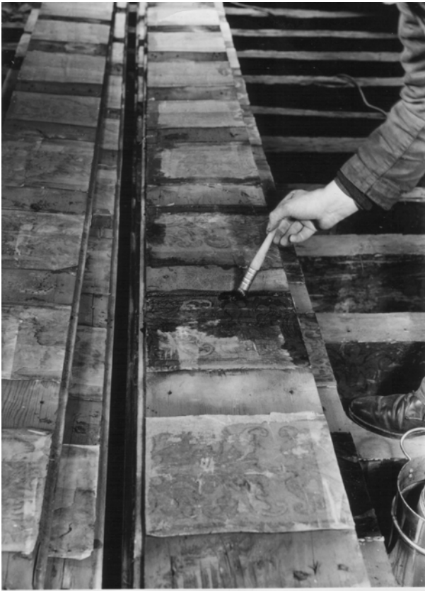
Illus. 1 Application of a gelatine facing to panels from the Riddle's Court ceiling on Lawnmarket, Edinburgh 1964
