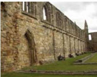
Cloister wall, clearly showing greater weathering at top half
