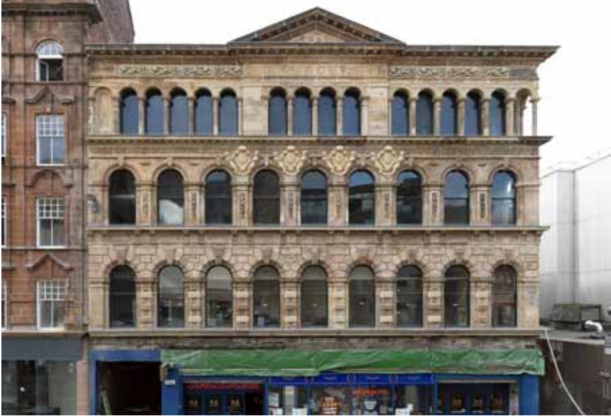
The newly restored façade of the Britannia Panopticon Music Hall in Glasgow's Trongate.
