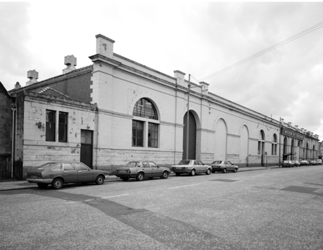
The former Tramway Works and Depot in Albert Drive, Glasgow in 1987 before its conversion to the Tramway Theatre. © Crown Copyright: RCAHMS. Licensor www.rcahms.gov.uk
