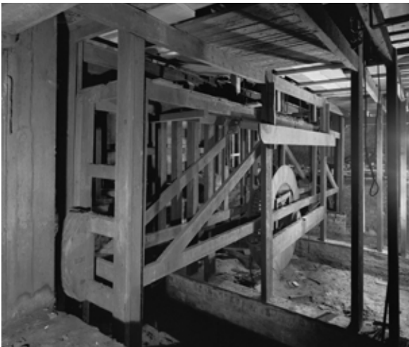
The basement of the Citizens Theatre in Glasgow in 1977, showing machinery for raising the scenery.
