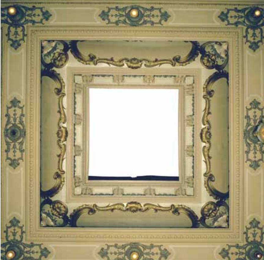
The sliding roof panel above the auditorium in the Pavilion Theatre, Glasgow.
