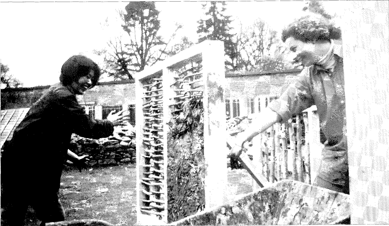
4a. Preparing test panels of clay walling
