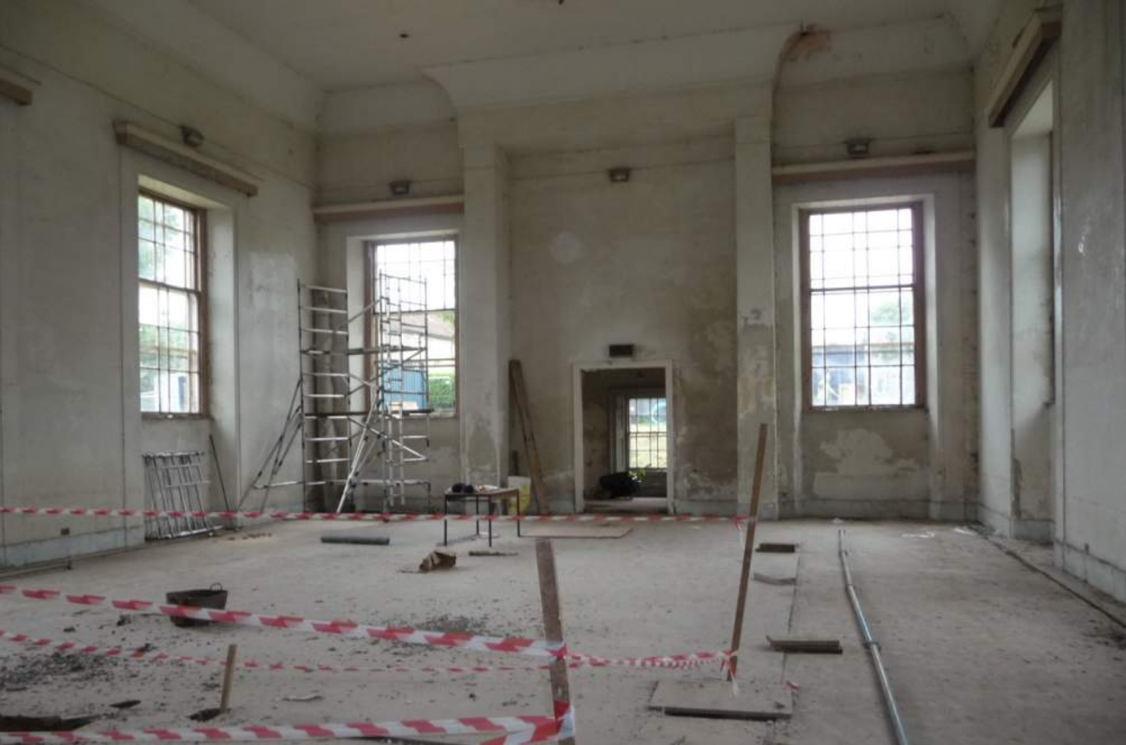
Above: The multi purpose hall in renovation ©SHBT
