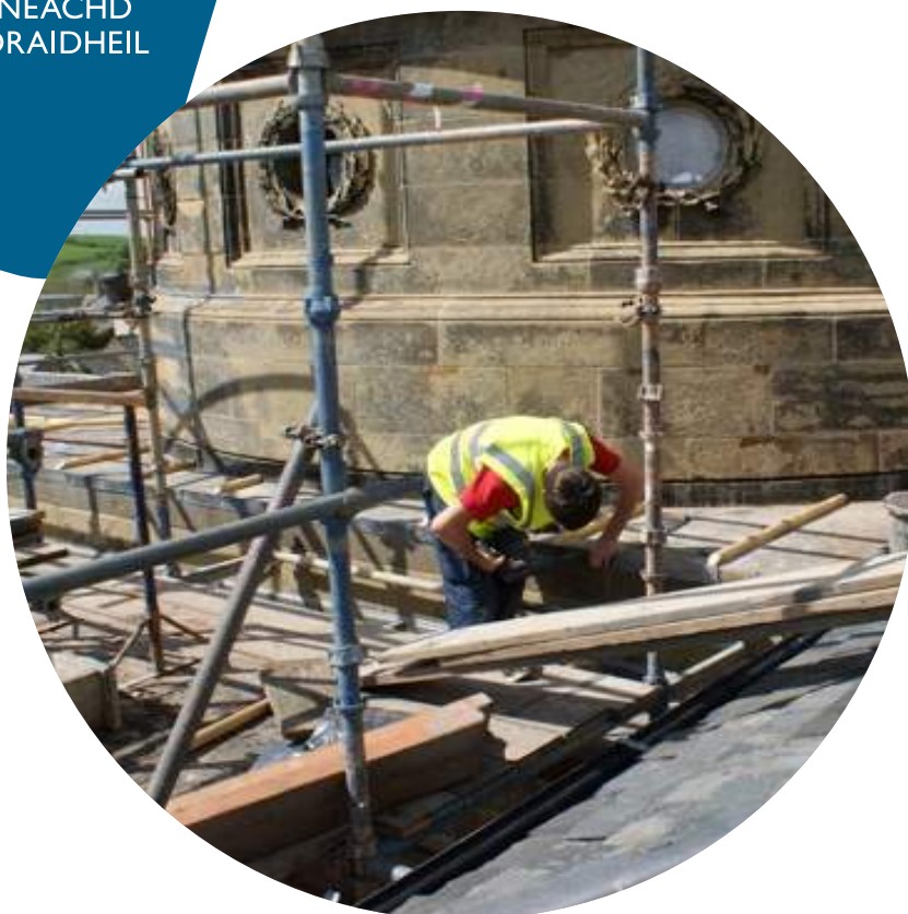
Roof and cupola restoration ©SHBT
