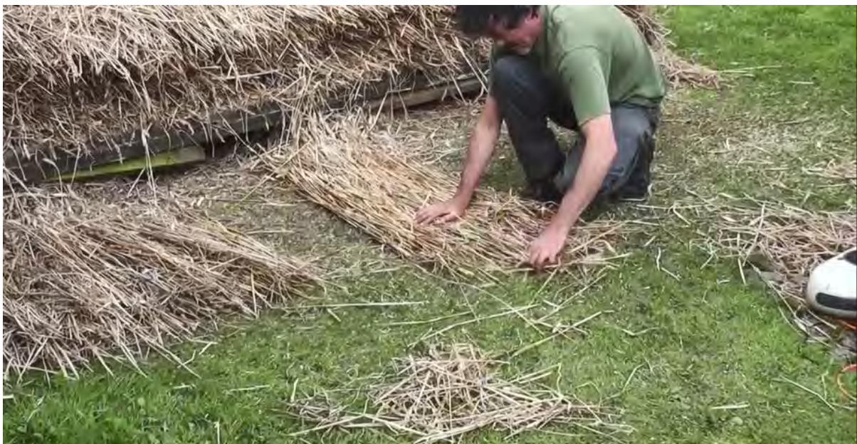
Figure 6. Yealming the straw - arranging it into bundles on the ground before combing it by hand. Image courtesy Cruck Cottage Heritage Association.
