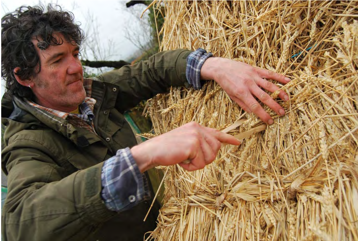
Figure 7. Fixing hazel scobs over sways formed from the thatching straw.
