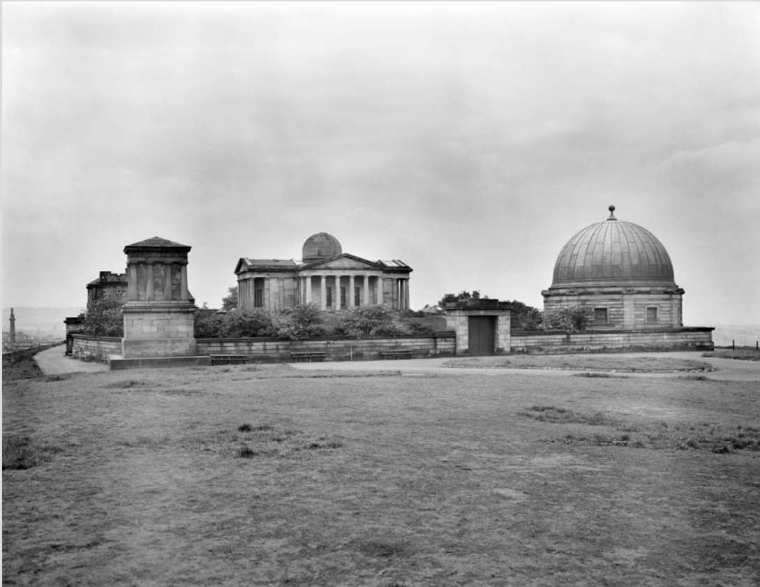
SC 1112808 © Crown Copyright: Historic Environment Scotland.
