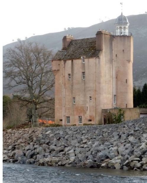
Flood Damage at Abergeldie Castle
