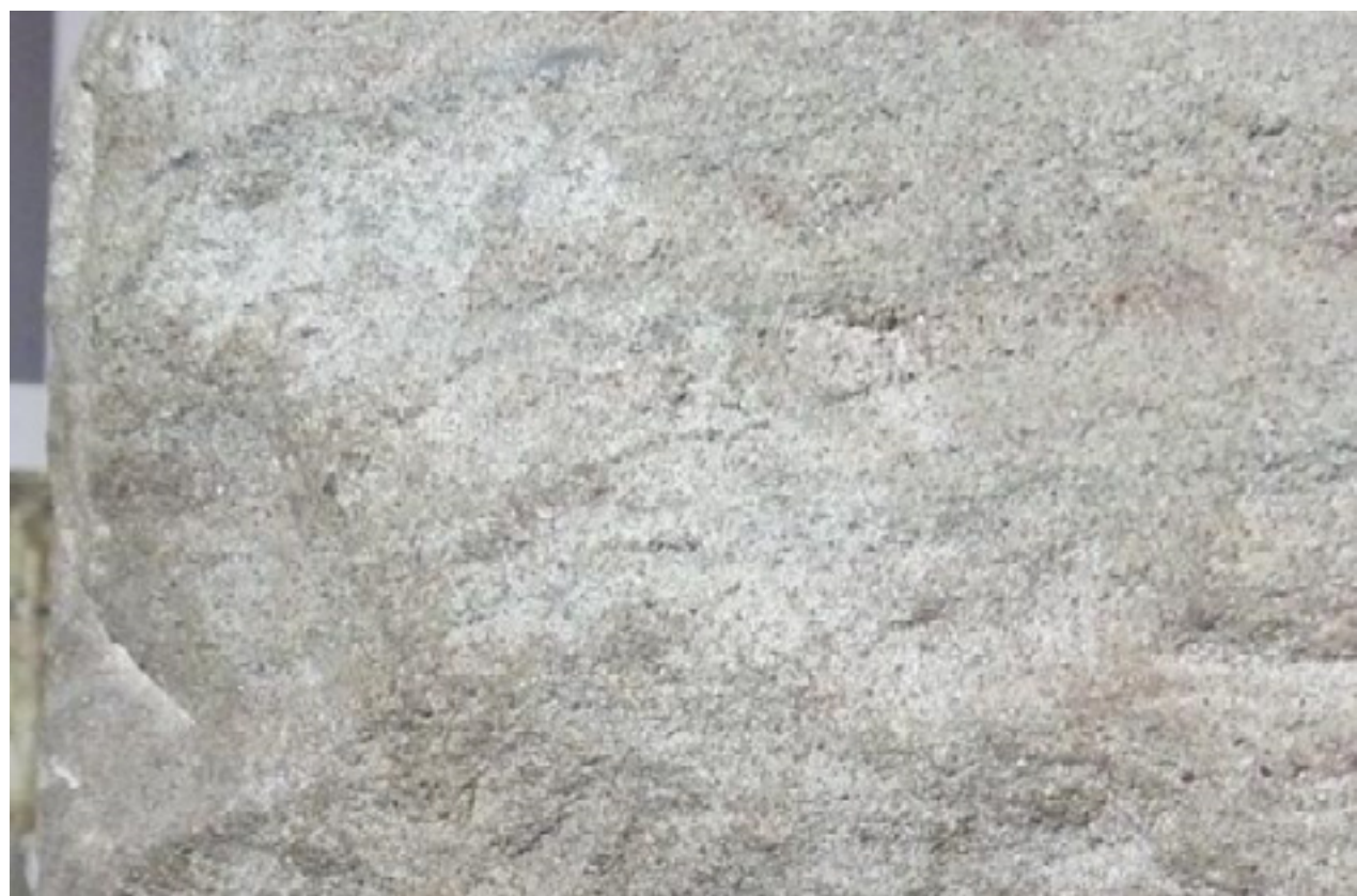
Fig 25. Photo record of the mineral mortar residue (2016).
