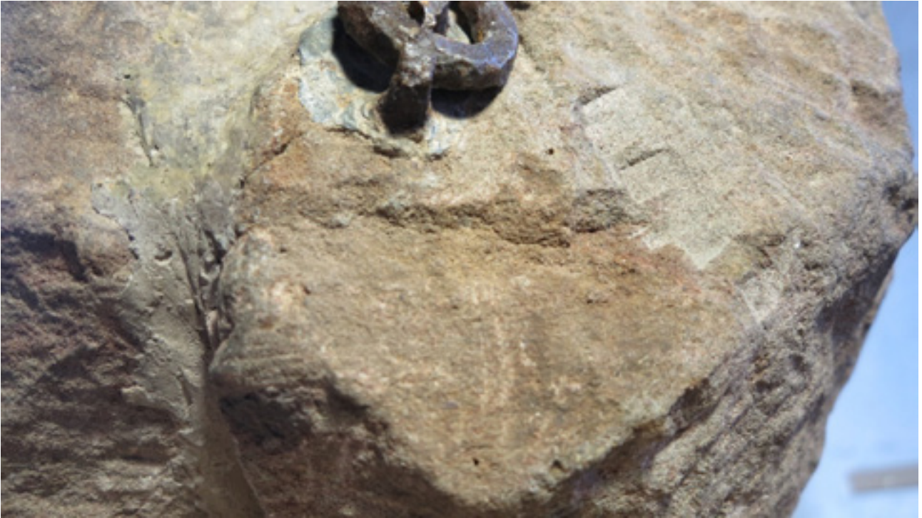
Fig 36. The sinister end face showing a visible fine crack and the area prone to flaking (2023).
