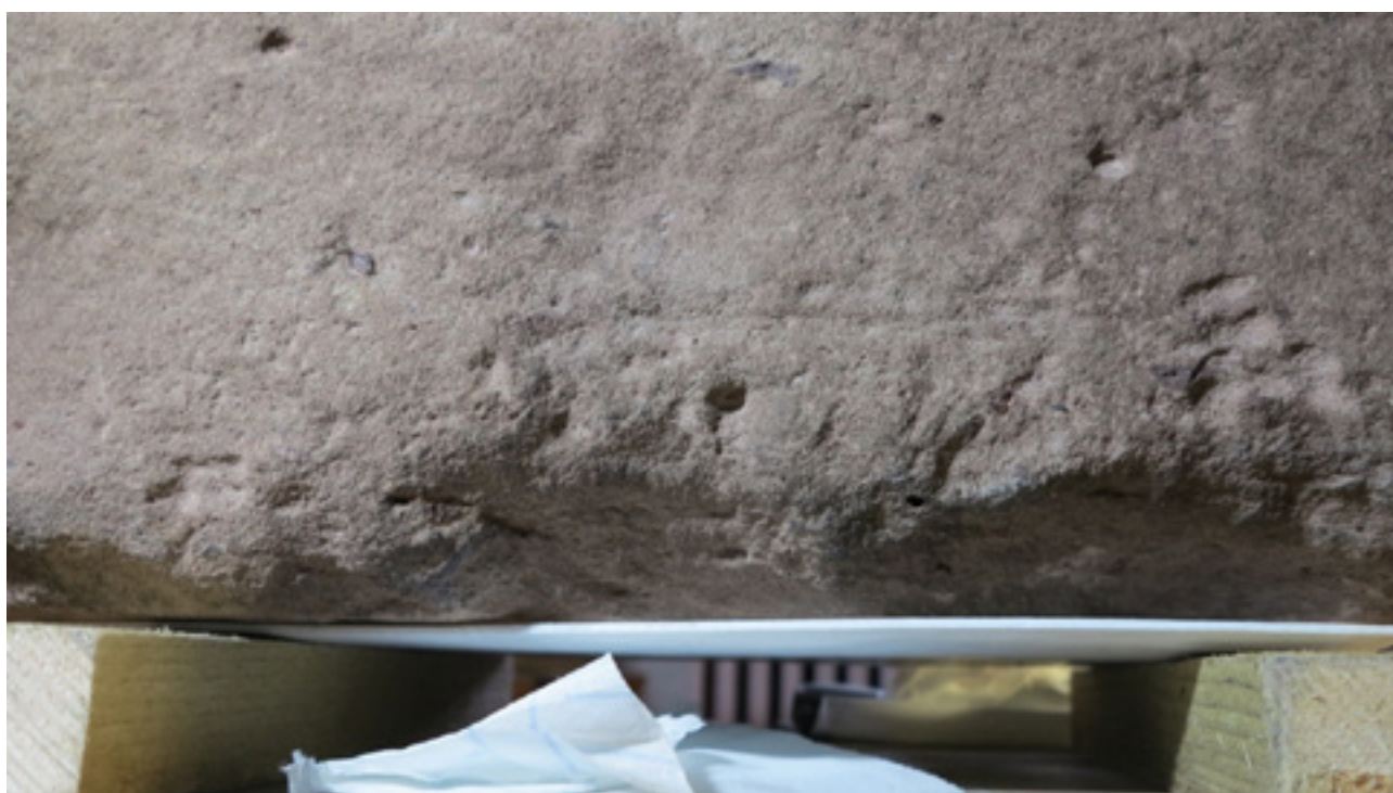
Fig 21. Lower edge of the front face. Visible fine fissure and a stone flake (2023).
