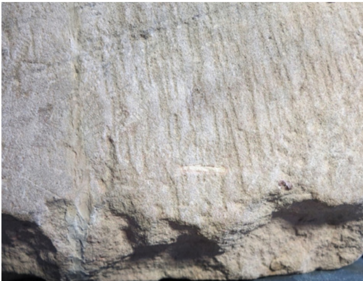
Fig 28. The same area as Fig. 27 after the replacement of the fill in 2023.
