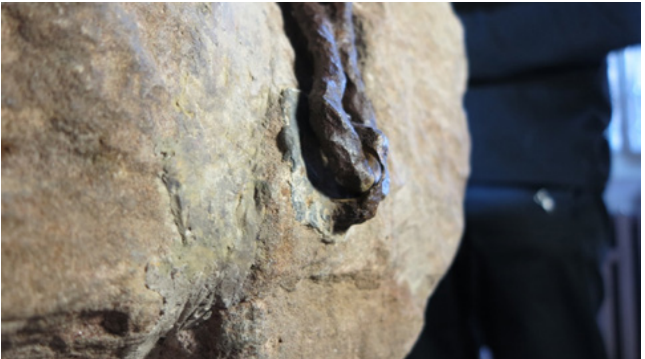
Fig 49. Close-up of the sinister face showing the thinness of the staple and its fragility and vulnerability to mechanical damage (2023).
