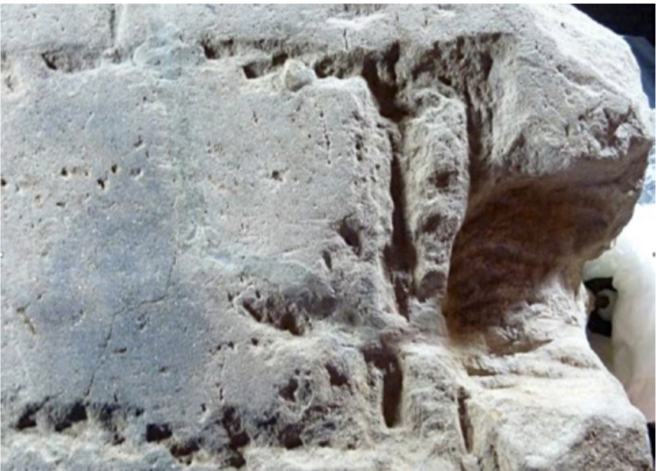
Fig 5. The top surface with a noticeable fine crack and dark staining in the middle of the Stone, photographed in 2016.
