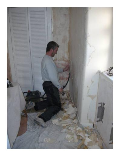
Fig. 3. Stripping of wallpaper and paint prior to application of calcium silicate board
