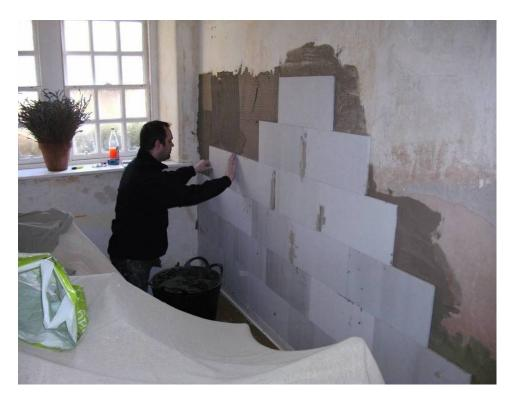
Fig. 4. Calcium silicate board being applied to a masonry wall at Wee Causeway
