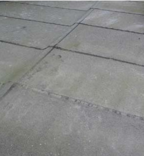
Flat roof covered in sheets of bituminous felt
