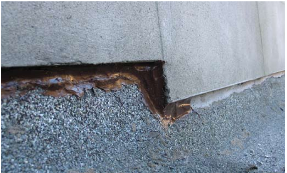
Repair to detailing where flat roof meets parapet wall
