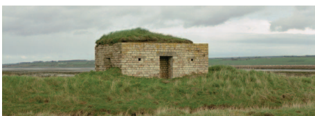
This brick -built pillbox was one of a series guarding the perimeter of an airfield from threat of invasion from the sea. © Crown Copyright: RCAHMS
