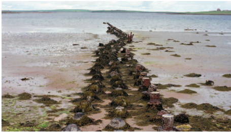
Anti-tank concrete blocks were set in single or multiple rows to obstruct the progress of enemy tanks. The most common were cubes, but square pyramids with flat tops (known as dragons' teeth) were often used. Today, small groups of such blocks represent all that remains of the original long defence lines. © Crown Copyright: Historic Scotland; RCAHMS
