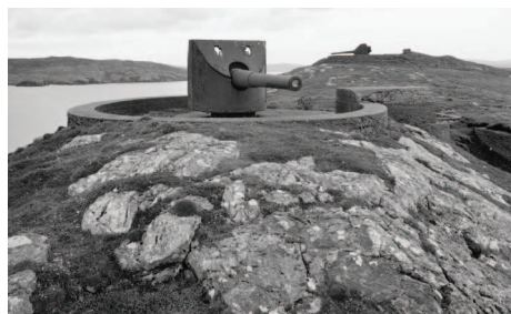
These two guns are part of the remains of a coastal battery on the remote hilltop at Swarbacks Head, Vementry, in Shetland. The site consists of two guns, ammunition magazines and an observation tower – typical features of coastal defence in Scotland.
