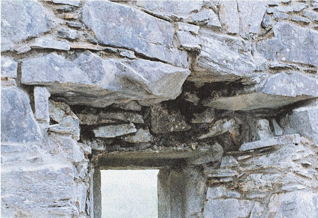
**12. The loss of lintels over wall openings can leave the masonry above in an apparently precarious state. However, where the individual stones are of relatively large size, and are deeply bedded in the wall core, the masonry may be less unstable than first seems. Each case has to be individually assessed, but the aim should be to do as little as is consistent with achieving stability.**
