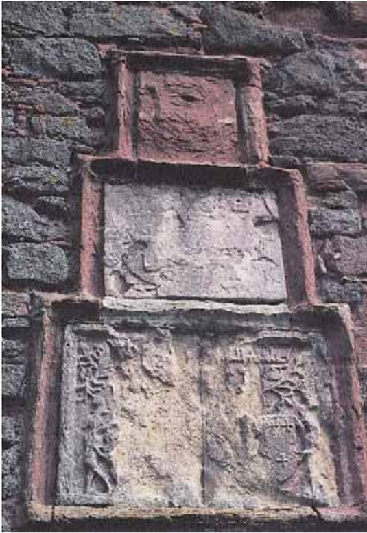
17. Carved panels are particularly prone to decay because the stones from which they are cut are usually set against their natural geological bedding, and long-term erosion takes place along the bedding planes. The process of decay may be accelerated when the protective framing mouldings have themselves failed.
