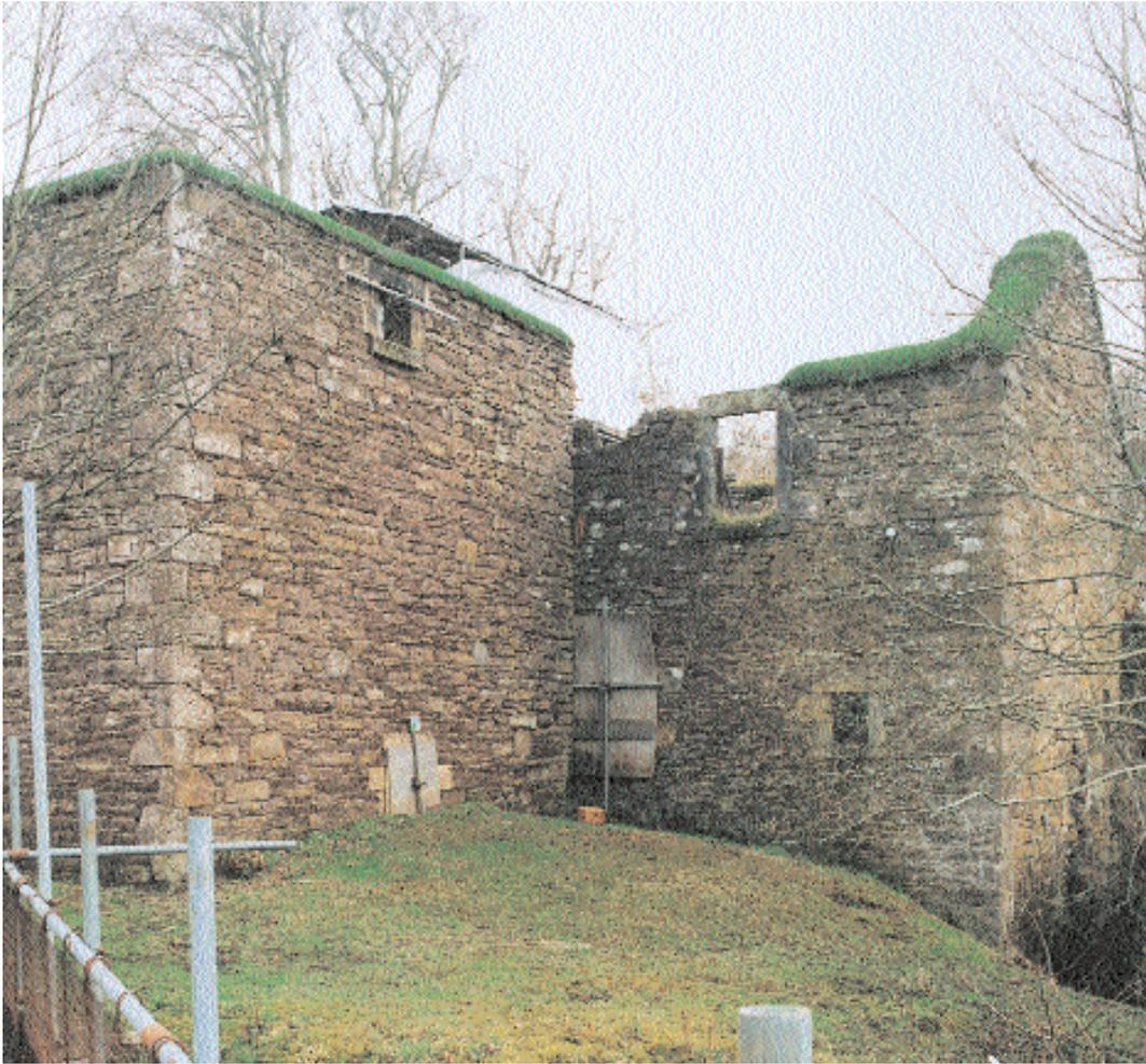
**11. In this view the wall-heads of a nineteenth-century mill building have been experimentally protected with turf strips, although this is a technique that is probably more generally appropriate for less complete structures.**
