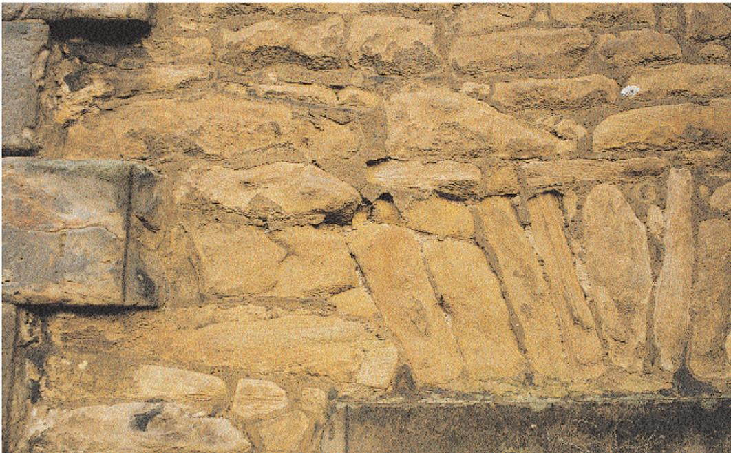
**22. Hard cement pointing can exacerbate masonry decay. Here some of the relatively modern cement pointing has been left proud of the adjacent stones as they have eroded. In other areas it can be seen that the original lime mortar survives within the narrow underlying joints where the cement has fallen away.**
