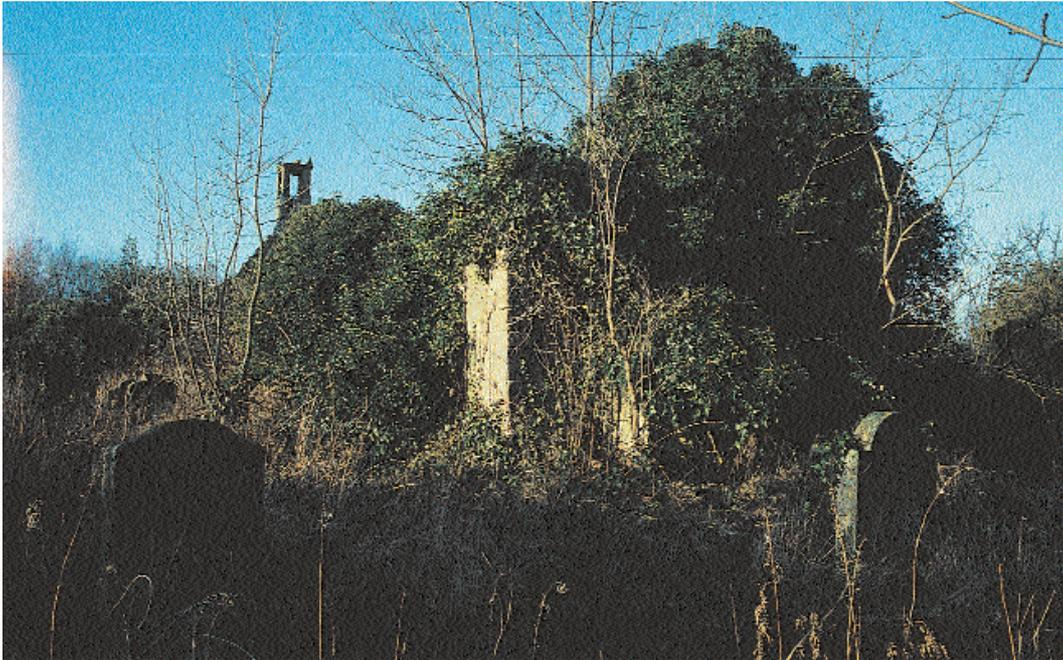
**43. In many cases, ivy has taken such a complete hold of a monument that the masonry is almost completely lost to sight. More importantly, however, the ivy will be certainly forcing its way into the joints and core of the stonework, while the constantly increasing weight of the growth may be a major threat to stability.**
