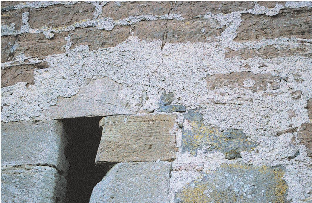
**23. Harling tends to survive only in a very fragmentary condition. It is found more often still attached to the rough surfaces of rubble than to smoothly finished ashlar, though in this view it clearly extended across both rubble and ashlar. The coating was sometimes thinner on smoothly dressed stone.**
