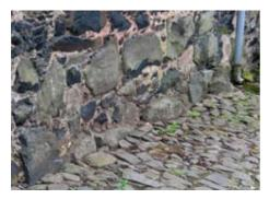
the gutter, running the risk of surface water flowing back towards the building's wall footing and foundations, especially if the surface slope away from the wall is slight, or non-existent. In addition, the impermeability of modern paving materials can trap underlying moisture adjacent to the wall footing.
