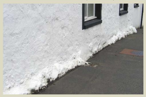
By Victorian times this protrusion had been regularised, and reduced in dimension, until only a minor thickening of the wall occurred at the footing. At the same time a more scientific approach emerged in designing foundations, resulting in the laying of proper load bearing strips upon which the building's walls were constructed.
