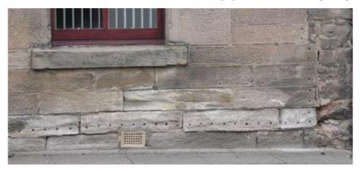
into the wall might include active and passive electro-osmotic techniques where electric currents are passed through the installed system in an attempt to control dampness.
