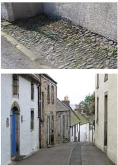
the build up of pavements leads to creating a small well at the foot of the building into which rainwater is discharged. This arrangement can also encroach onto the external face of wall foot ventilators, allowing water access directly into the sub-surface of the building through the vent slots. Unfortunately, increases in modern road level surfacing sometimes also eliminates
