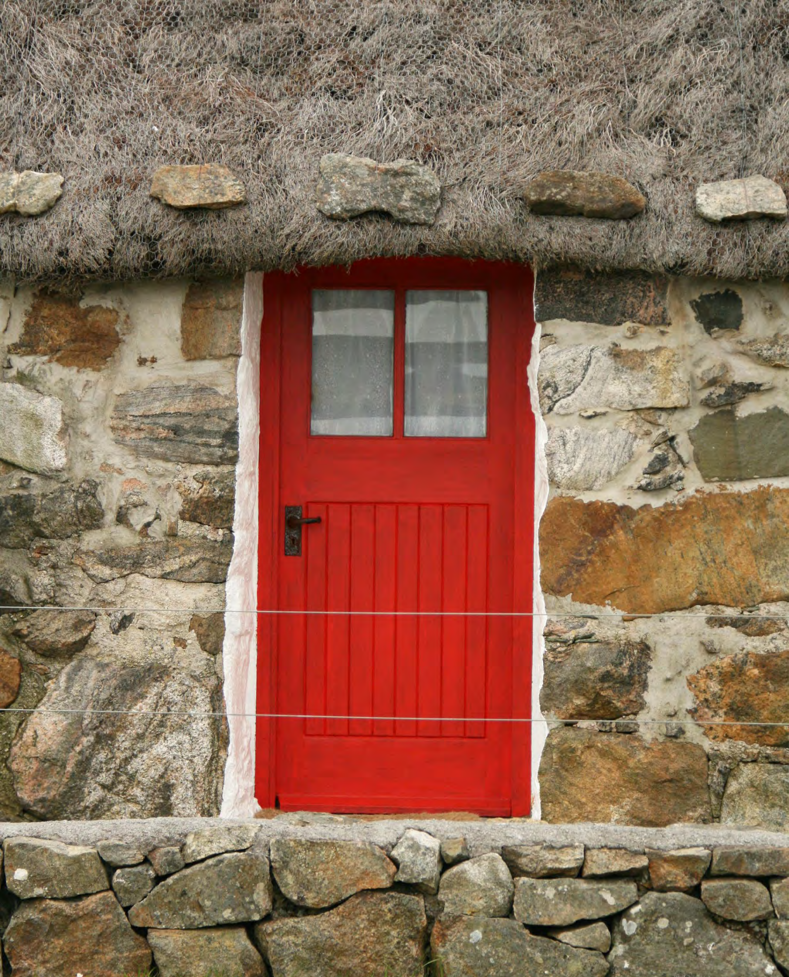
Full-page image 3: Detail of a netted heather-thatched roof above a doorway at Loch Baghasdail a Deas, Uibhist a Deas ~ South Lochboisdale, South Uist. © Courtesy of HES (Society for the Protection of Ancient Buildings Collection).
