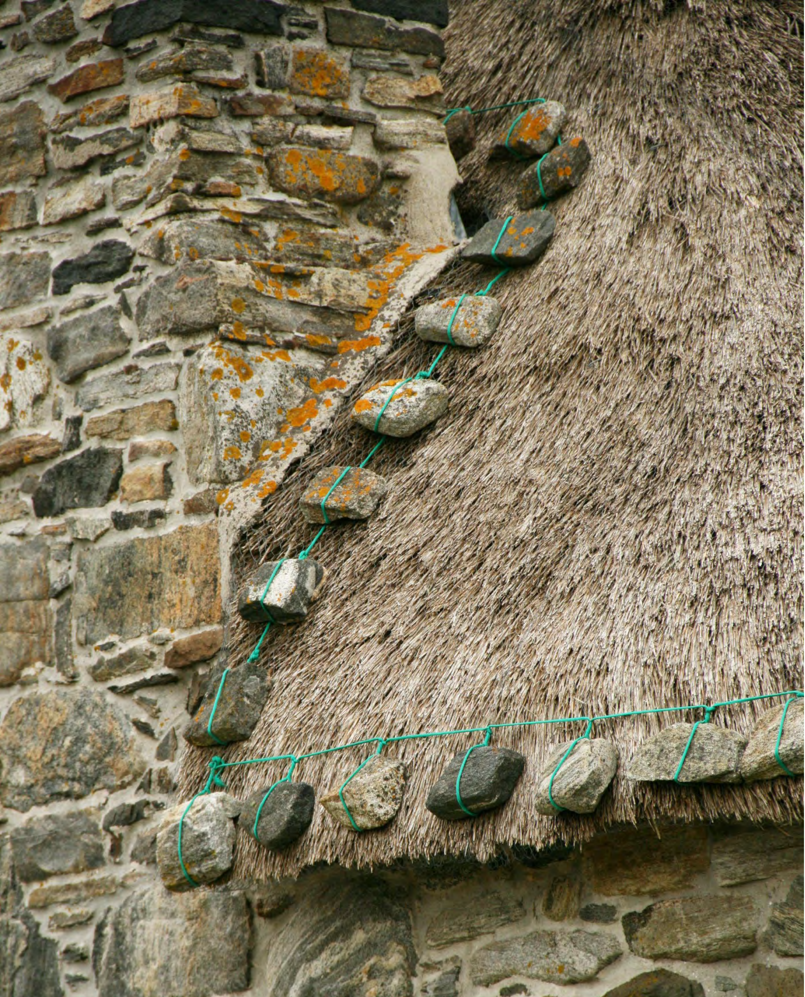
Full-page image 1: Detail of weighted marram thatch on a renovated cottage at Rubha Ghaisinis, Uibhist a Tuath ~ Rughasinish, South Uist. © Courtesy of HES (Society for the Protection of Ancient Buildings Collection).
