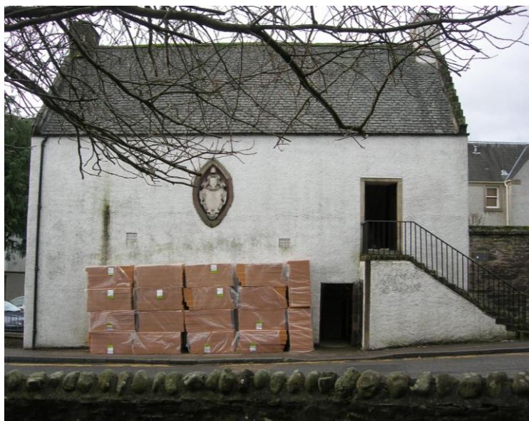
Fig. 3. Insulation arrives on site during the improvement works
