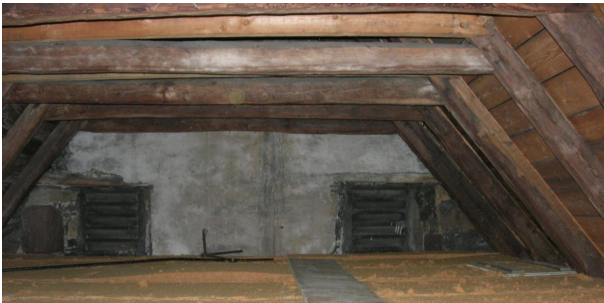
Fig. 6. Existing vents retained for ventilation
