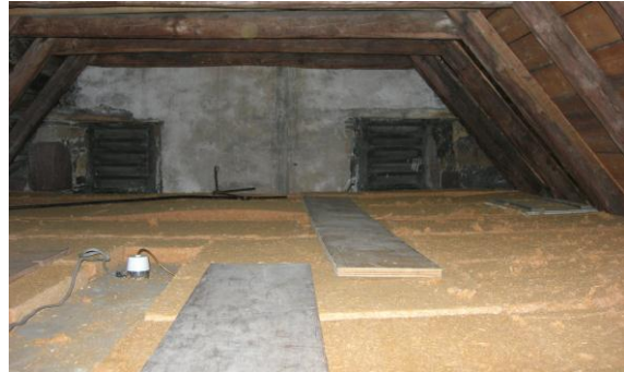
Fig 5. Wood fibre boards fitted with no gaps
