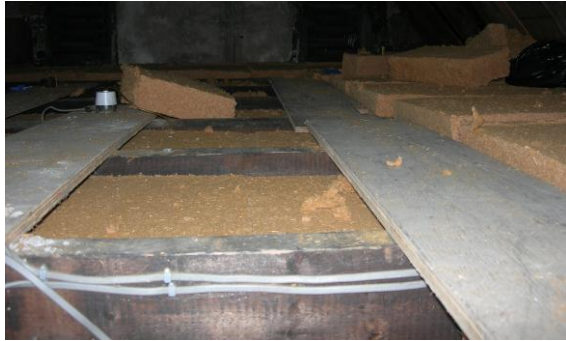
Fig 4. The wood fibre board fitted between the ceiling joists
