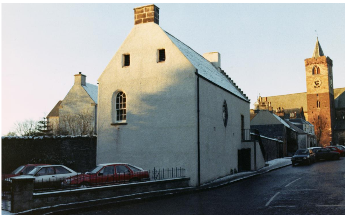
Fig. 7. South-east gable of library showing the two loft vents at upper level. © Newsquest (Herald & Times). Licensor www.scran.ac.uk
