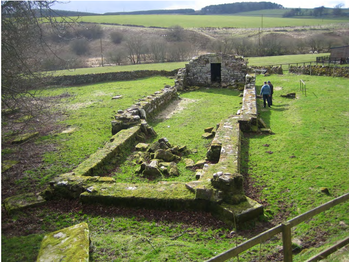
Figure 3. Souden Kirk viewed from the north east; the choir in the middle foreground, with the nave and the rebuilt tower in the middle right.
