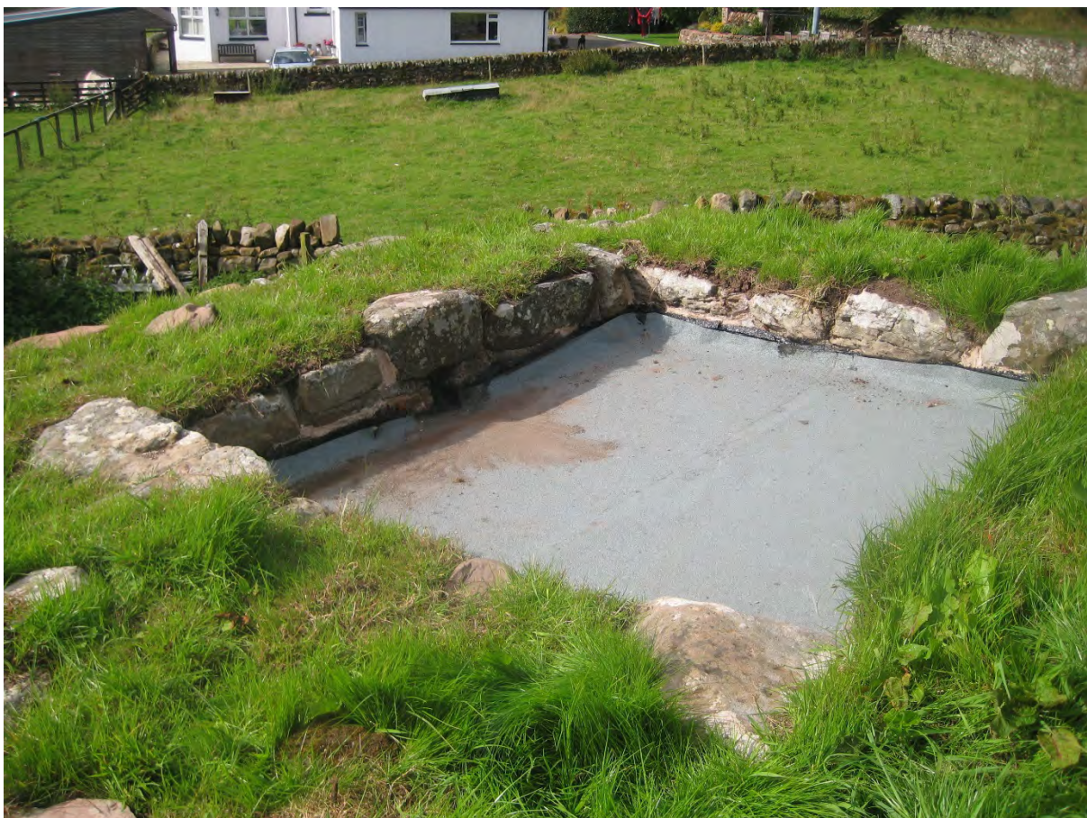
Figure 10. The roof and soft capping photographed in 2016.
