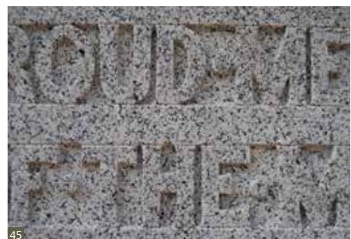
Fig 45 Loss of definition to granite lettering following cleaning.
