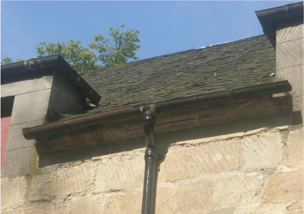
Fig. 3. Existing rhones were repaired and downpipes made good
