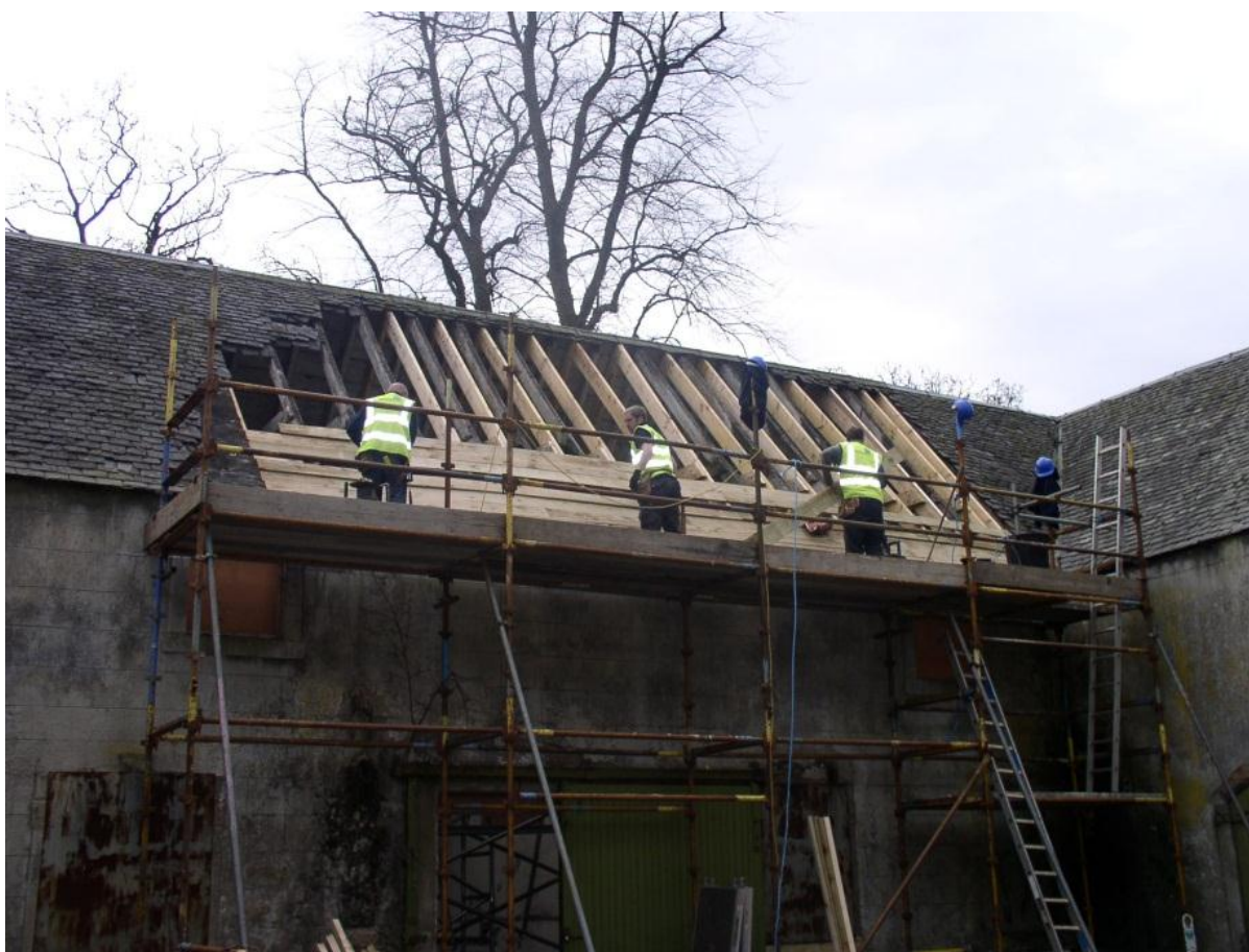
Fig. 6. Fixing the sarking boards onto the new trusses
