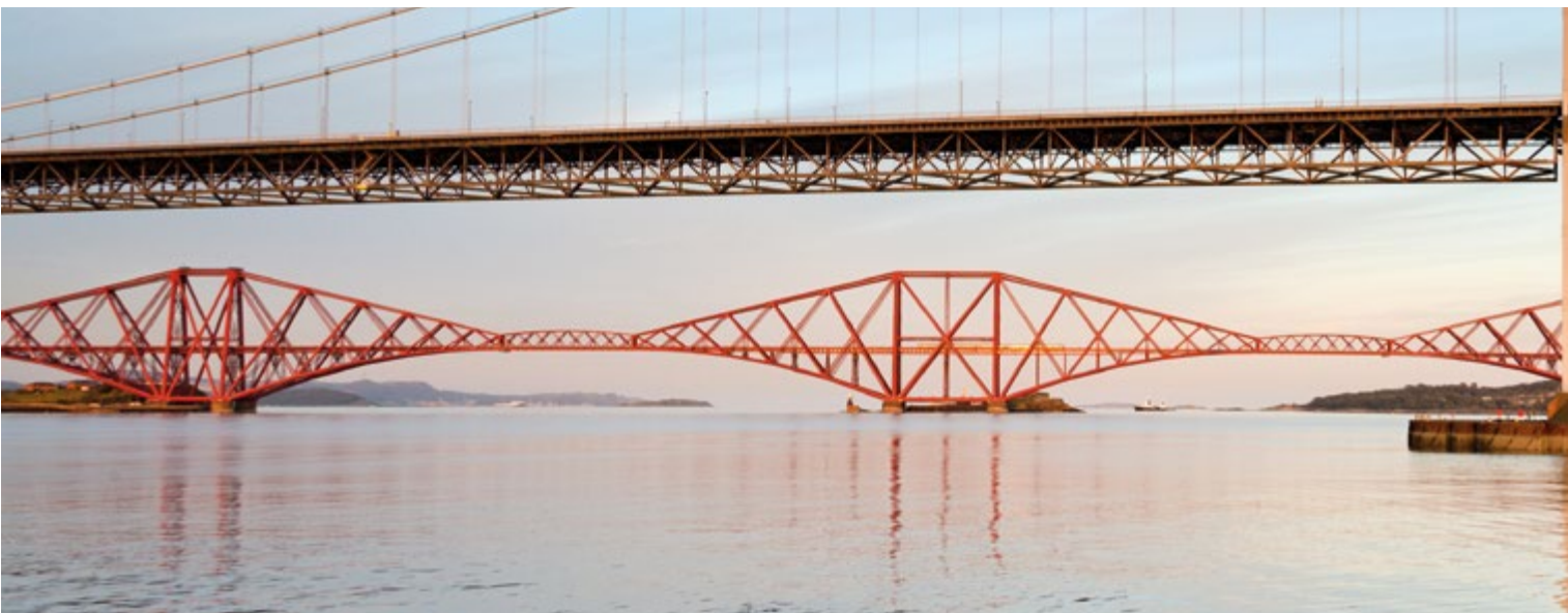
The Forth Bridge and Forth Road Bridge.
