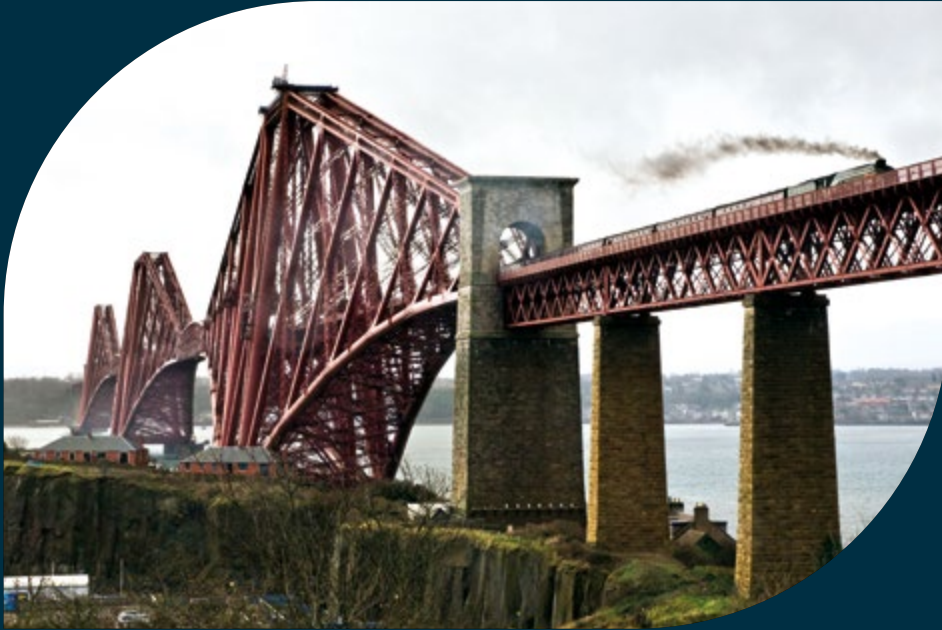
The Forth Bridge from the Fife Coastal Path.
