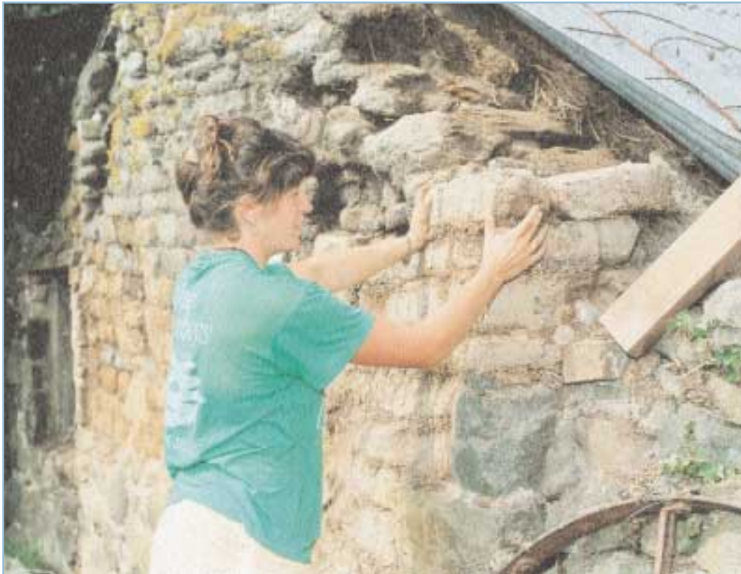
Vernacular building repair, near Huntly, Aberdeenshire.
