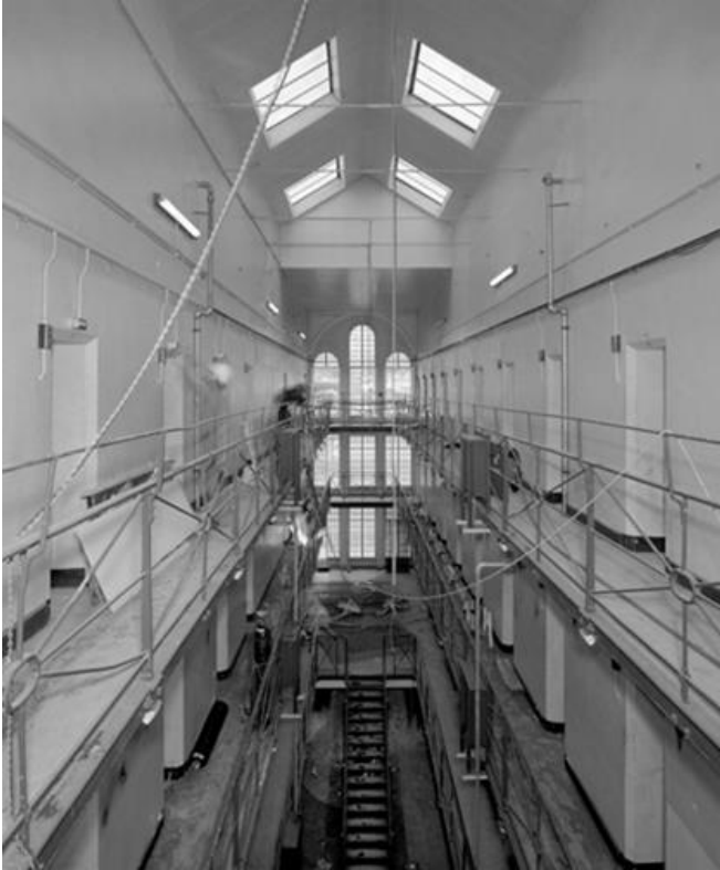
Fig 19. Perth prison, former D Hall, Robert Matheson, 1857 © Crown Copyright: Historic Environment Scotland
