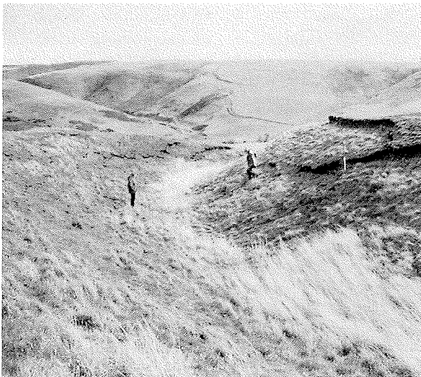
Figs 13 & 14. Addinston hillfort, Lauder, Scottish Borders: before and after the beneficial effects of rabbit and stock control. Crown copyright: Historic Scotland.
