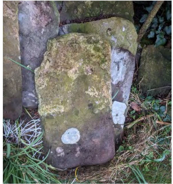
Figure 58: A flagstone slate from the roof, showing the remains of a peg in the single head hole and traces of mortar bedding. © Sara Carruthers.
