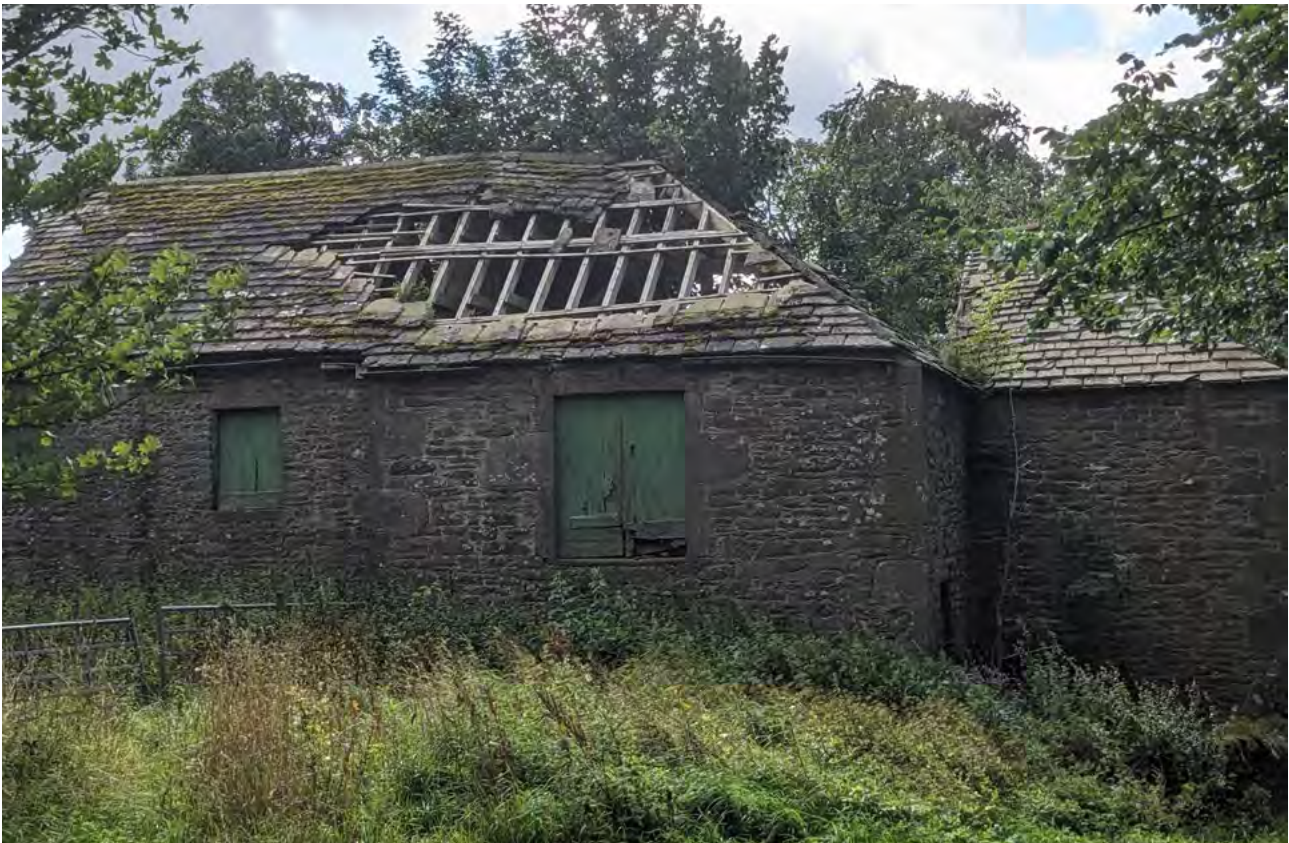
Figure 23: South Balluderon Mill and Steading, Tealing, with the formation of battens and slates visible. © Sara Carruthers.
