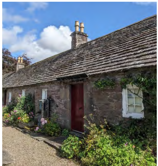
Figure 32: Eaves with an overstop in Kirkwynd, Glamis. © Sara Carruthers.
