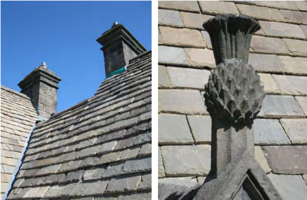
Figure 42a and b: Acheson House roof after new stone was laid. © Denfind Stone Ltd.
