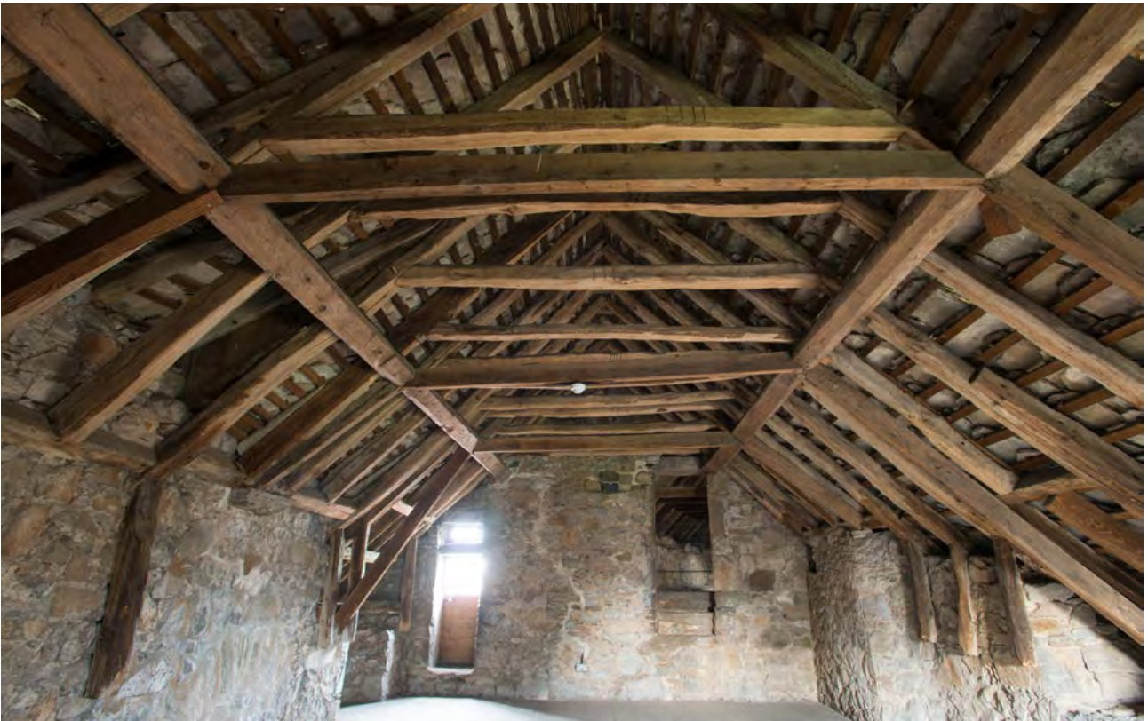
Figure 14: The interior roof structure of Claypotts Castle, Dundee.
