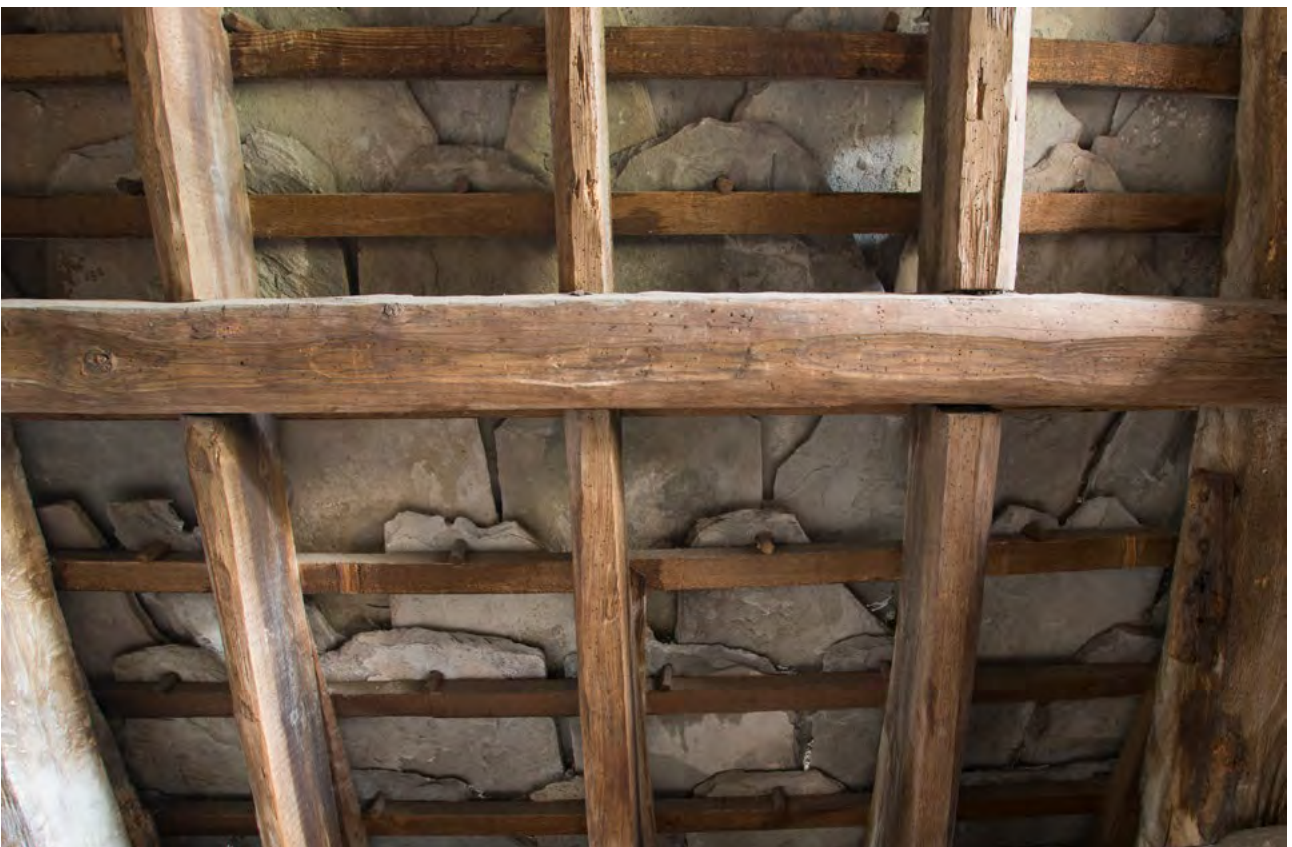
Figure 15: Batten and peg method of laying flagstone, Claypotts Castle, Dundee.
