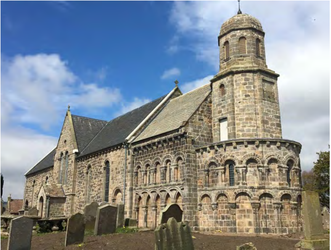
Figure 50: The completed repairs at St Athernase, showing the flagstone roof on the chancel. © Denfind Stone Ltd.
