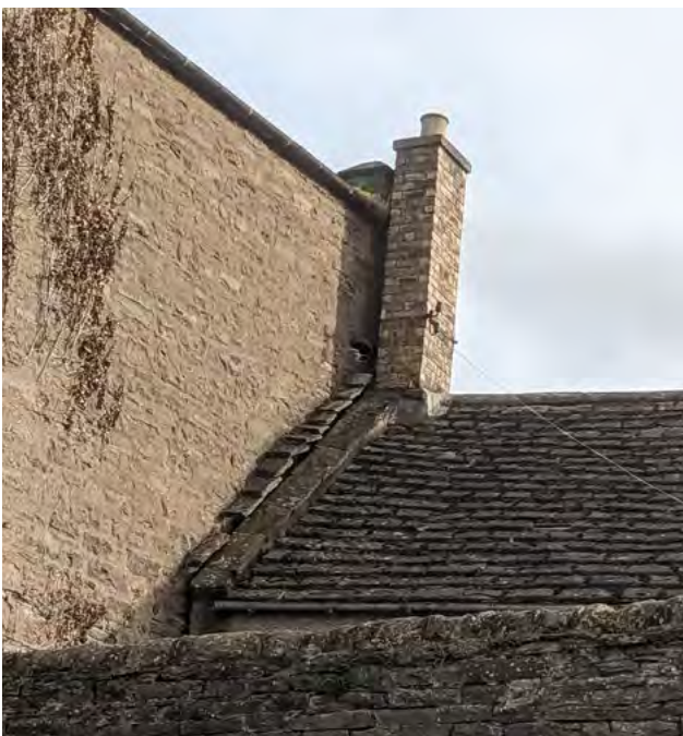
Figure 31: Stone flashings in St James Road, Forfar. © Sara Carruthers.
