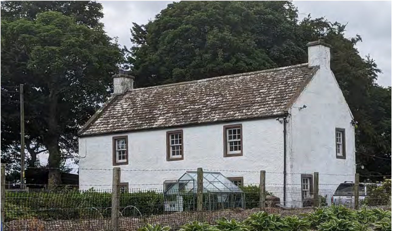
Figure 28: A roof detailed with skewes and a stone ridge. Priory House, Restenneth near Forfar, Angus. © Sara Carruthers.
