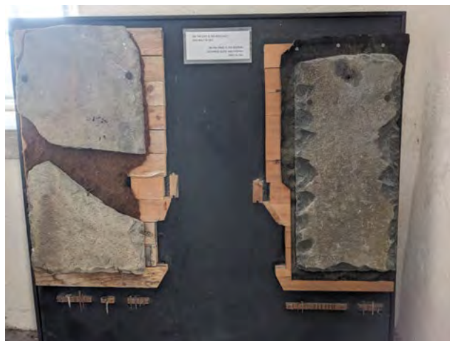
Figure 7: A wall display from Duart Castle, contrasting flagstone slates from 1911 (left) and 1990 (right). © Sara Carruthers.
