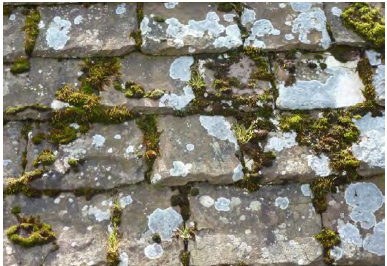
Figure 47: Part of St Athernase north roof, prior to repair. © Douglas Binnie.
