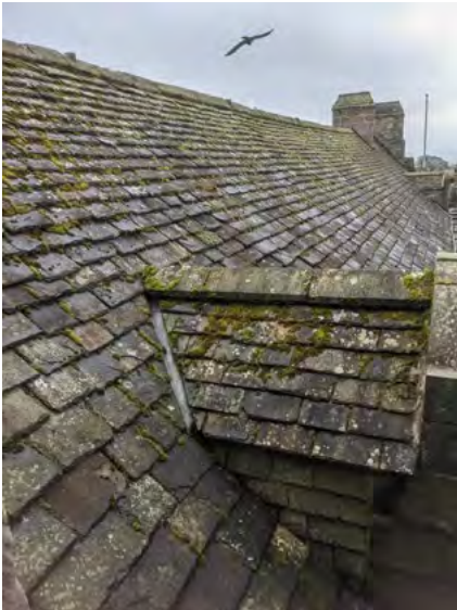
Figure 53: The flagstone-roofed south elevation of the South Range, Falkland Palace. © Sara Carruthers.
