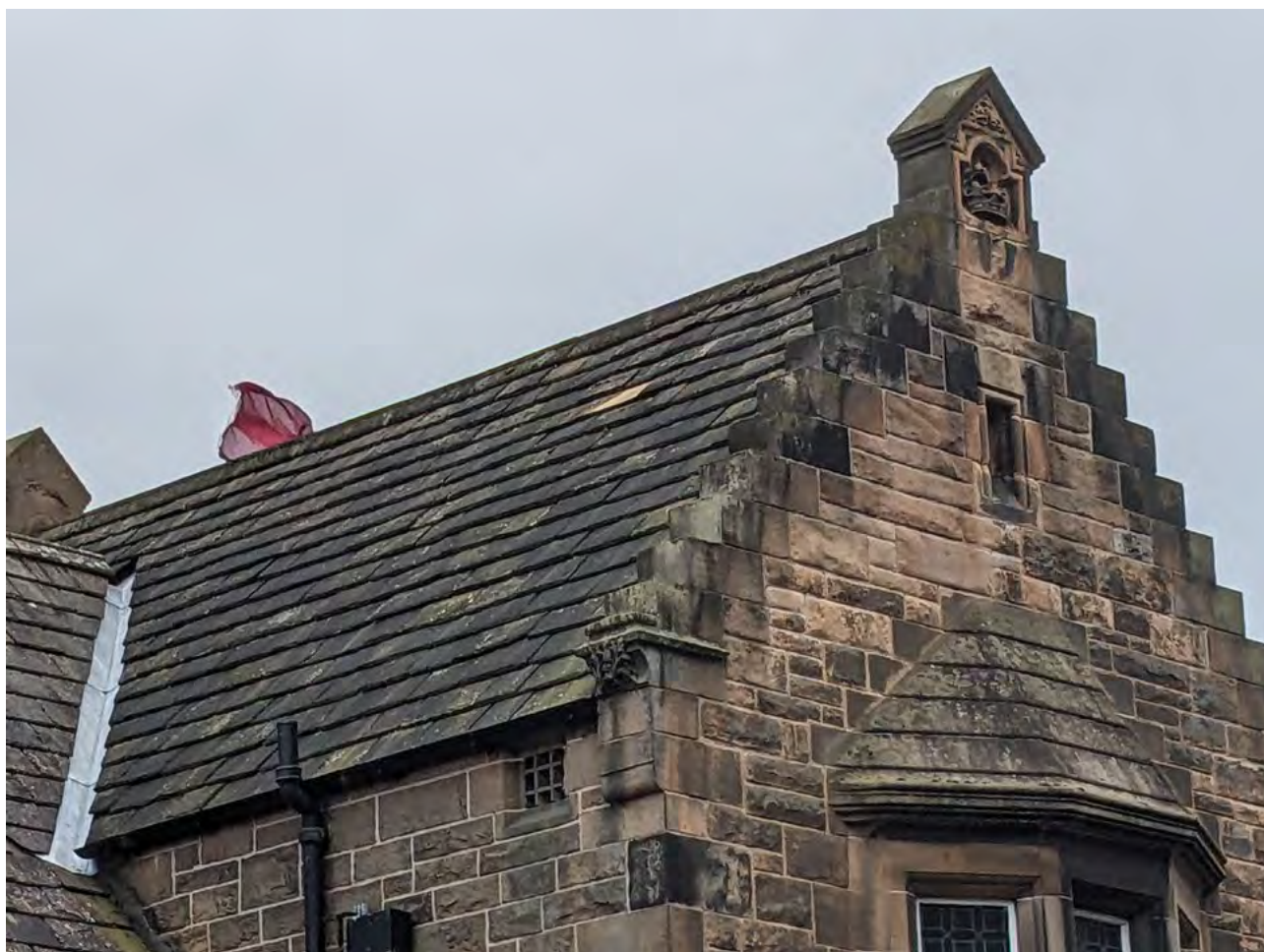
Figure 1: Angus flagstone roof on the Gatehouse at Edinburgh Castle. © Sara Carruthers.
