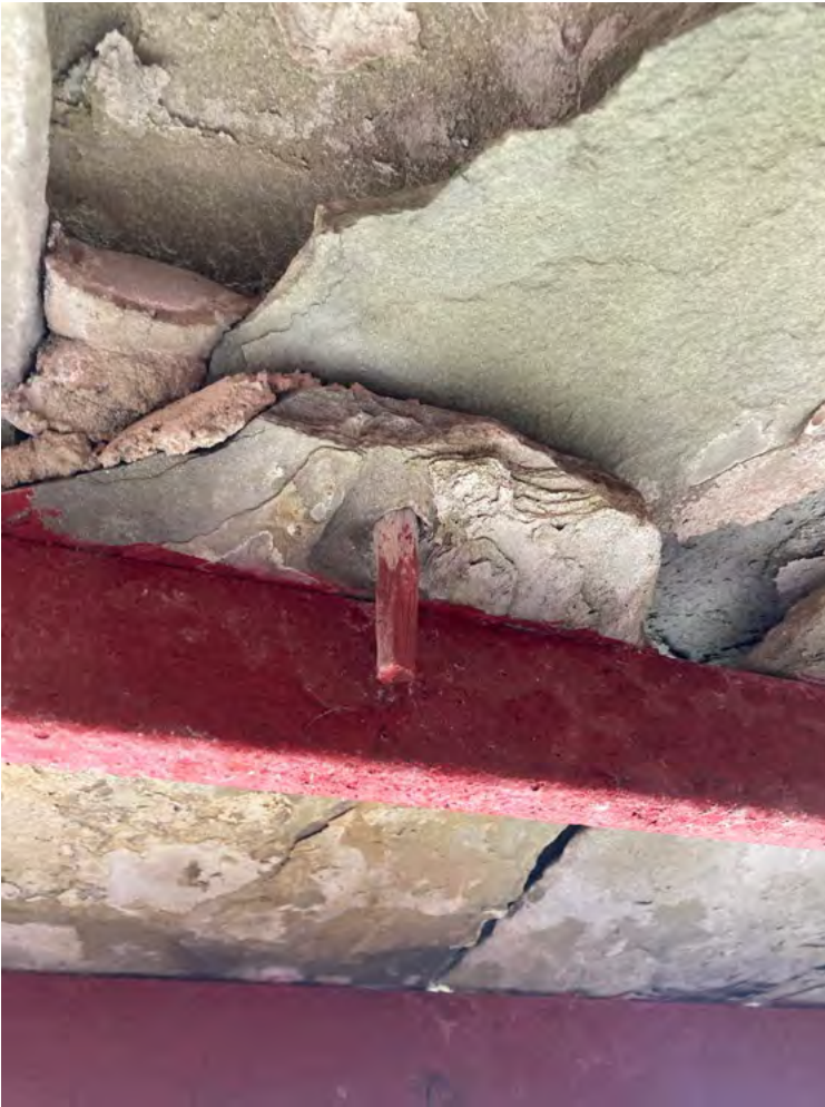
Figure 20: Batten and peg method of laying flagstone on a shelter at Arbroath Signal Station. Lime mortar bedding is still visible. © Graham Briggs.
