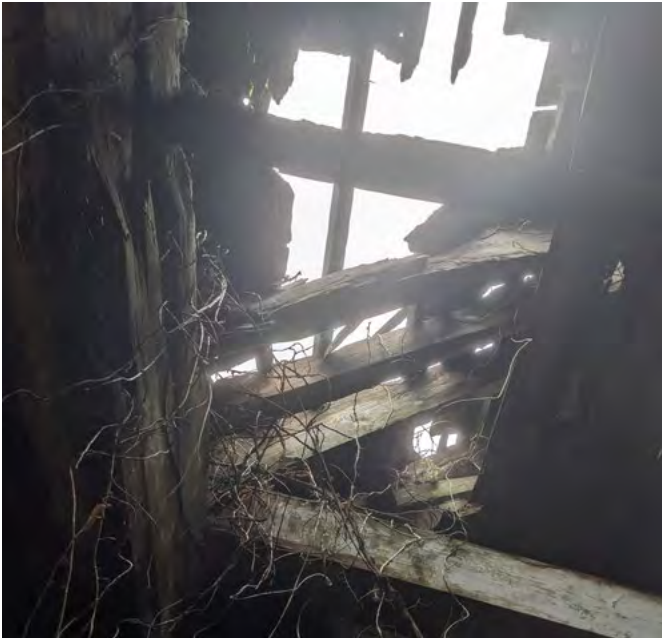
Figure 57: The roof structure of Monimail Morthouse, showing worked rafters and battens. © Sara Carruthers.
