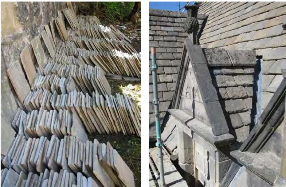
Figure 41a and b: Acheson House during re-roofing. © British Geological Survey.
