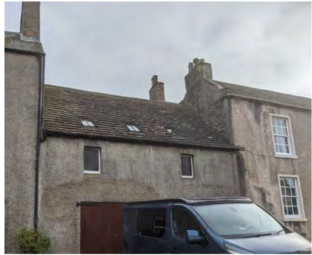
Figure 34: Rooflights in Little Causeway, Forfar. © Sara Carruthers.
