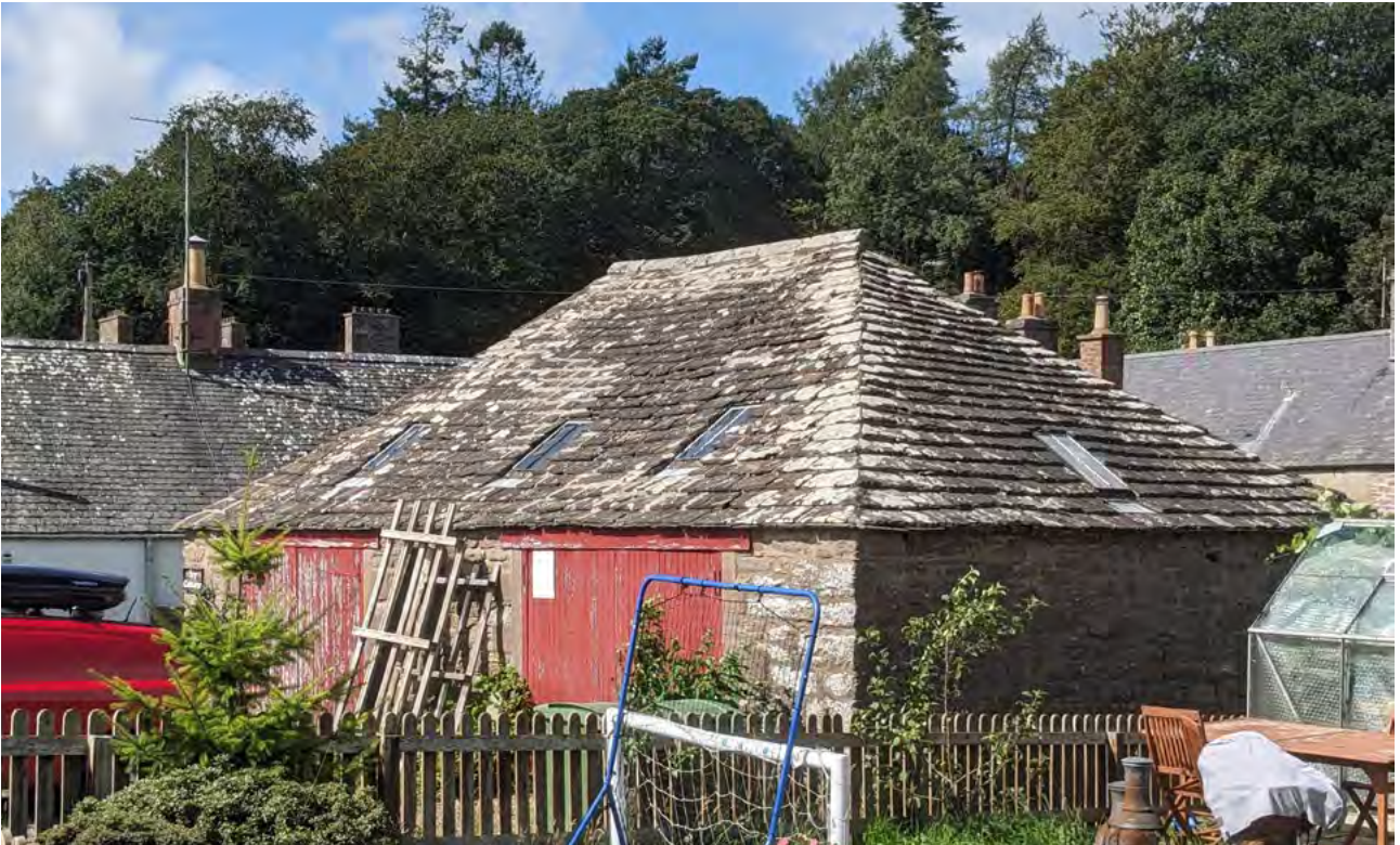
Figure 26: An example of mitred hips at Gig House, a workshop in Glamis. © Sara Carruthers.
