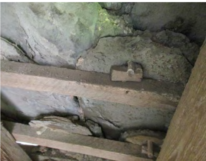
Figure 21: Historic pegs, packers and lime mortar bedding at Pittenweem Tolbooth, Fife. © Arc Architects.
