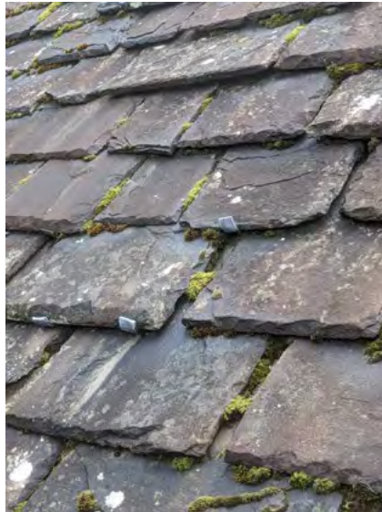
Figure 54: Replacement slates held in place with tingles, Falkland Palace. © Sara Carruthers.
