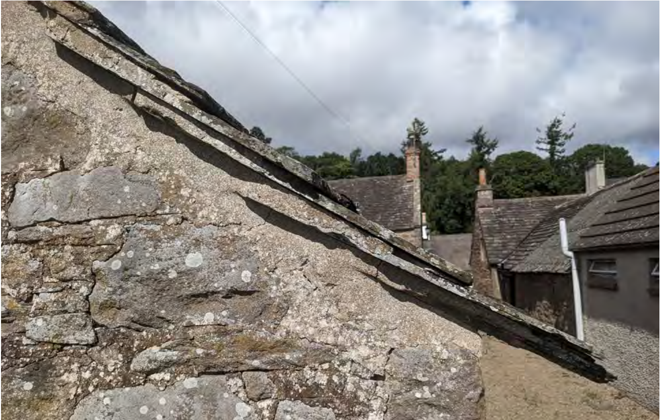
Figure 30: Detail of lapping and verge in Back Dykes, Glamis, Angus. © Sara Carruthers.
