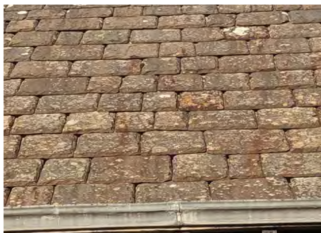
Figure 9: A detailed view of the flagstone slates on the roof of the north transept of St Clement's Chapel. © Sara Carruthers.
