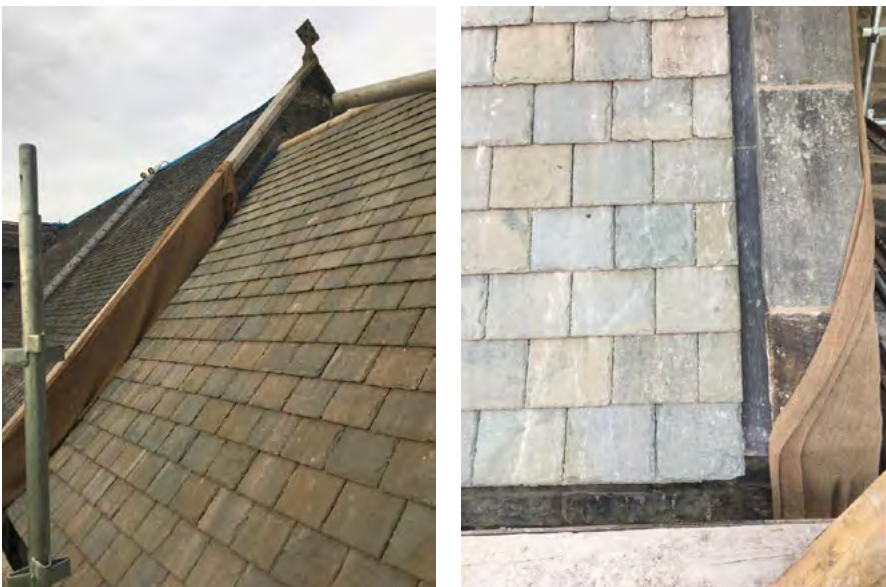
Figure 49a and b: The completed roof of St Athernase. © Douglas Binnie.
