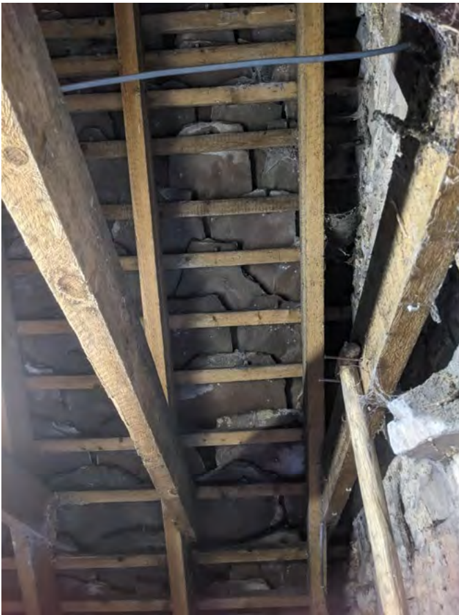
Figure 16: Batten and peg method of laying flagstone on an outbuilding at Templeton Farm, Angus. © Sara Carruthers.
