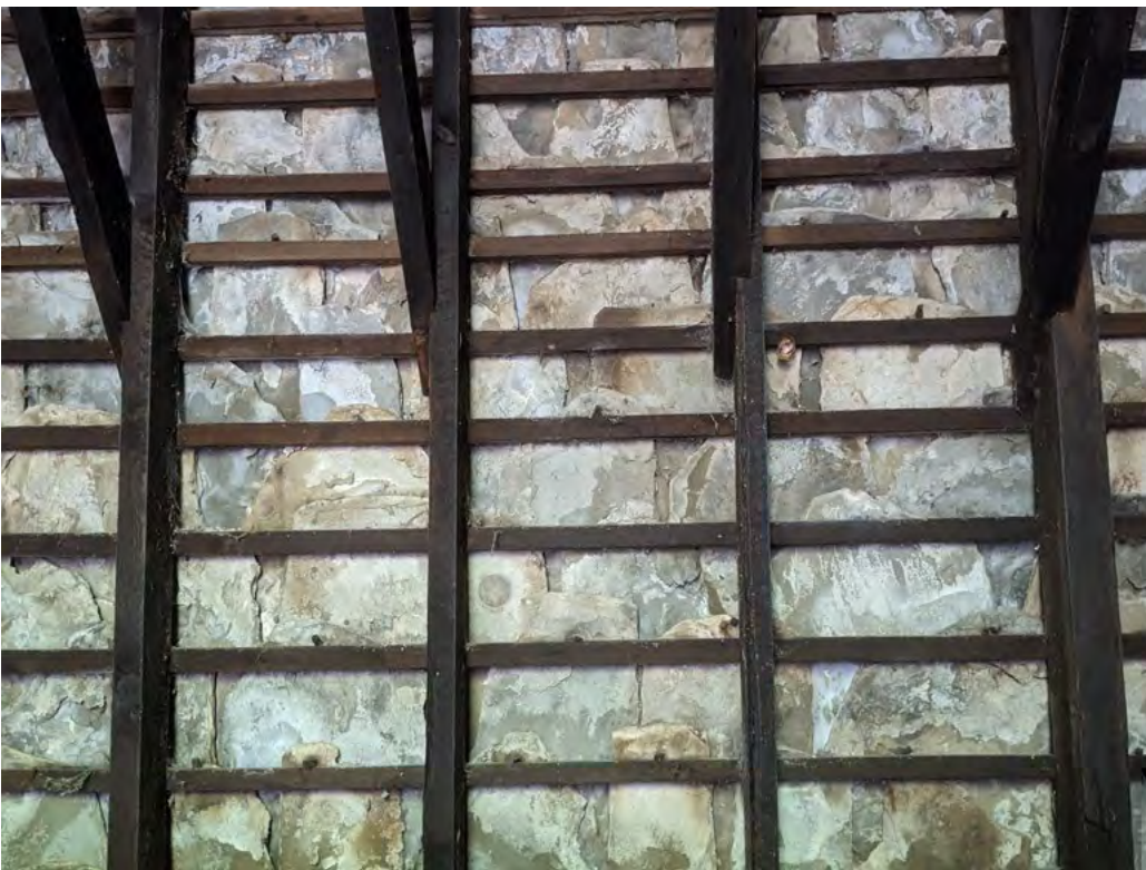
Figure 18: Interior showing the batten and peg method of laying flagstone at Tealing Doocot, Angus. © Sara Carruthers.
