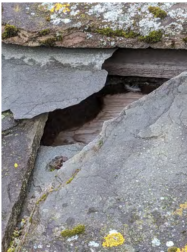
Figure 52: Close-up of a broken slate on the south elevation of the Abbot's House. © Sara Carruthers.
