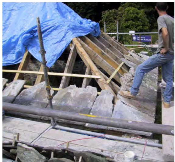
Figure 22: Roof repairs in progress at Pitmuies Estate, Angus, showing lime mortar bedding, pegged slates and battens. © Ian Cumming.
