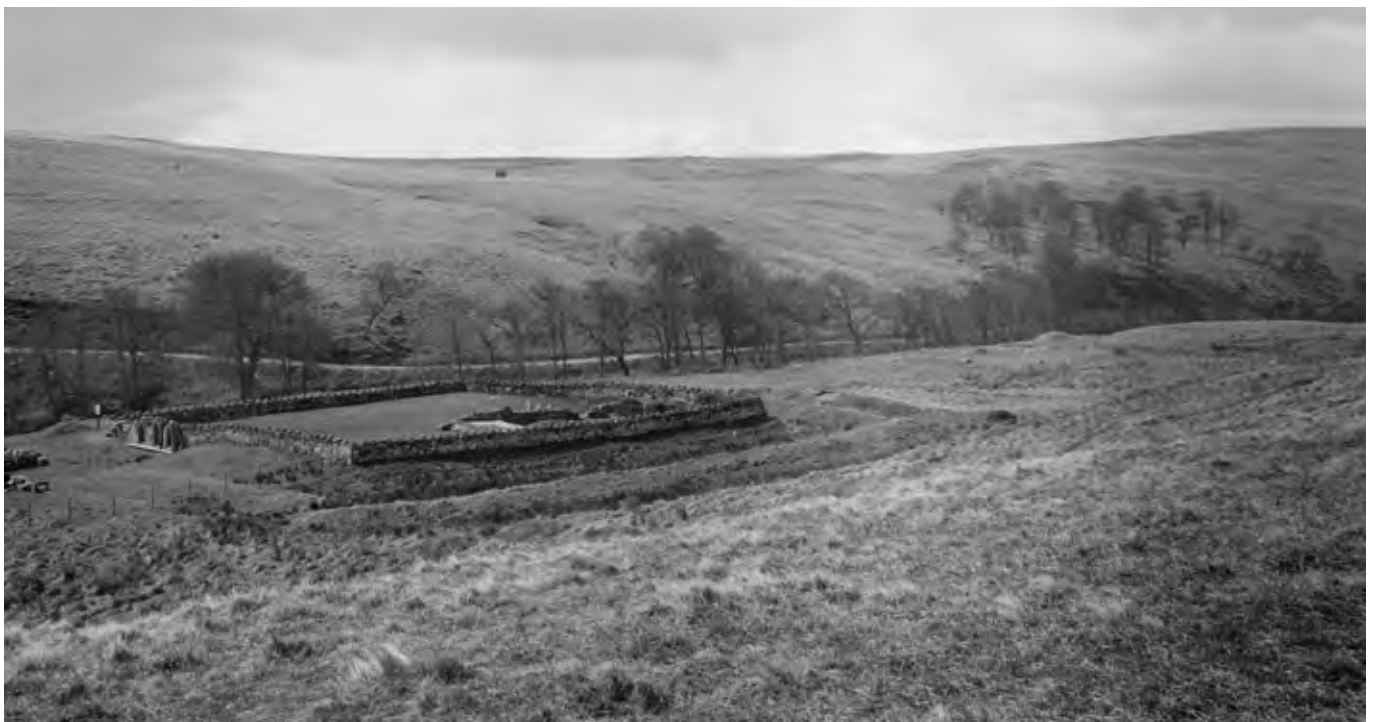
Fig 19 The moated enclosures at Hermitage, Scottish Borders are likely to be the predecessor of the nearby castle at Hermitage. SC1260663.
