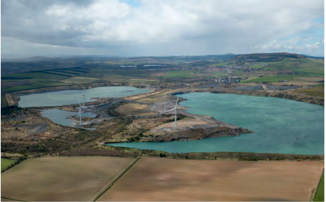
Fig 86 Westfield open castmine, Fife, now used as a wind farm. DP153383.
