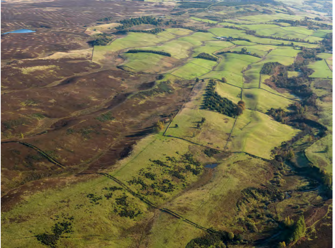
Fig 16 Buzzart Dikes deer park occupies the three ridges in the foreground, enclosed by a bank and internal ditch. The bank was surmounted by a wooden paling, evidence for which was revealed through excavations. DP056572.
