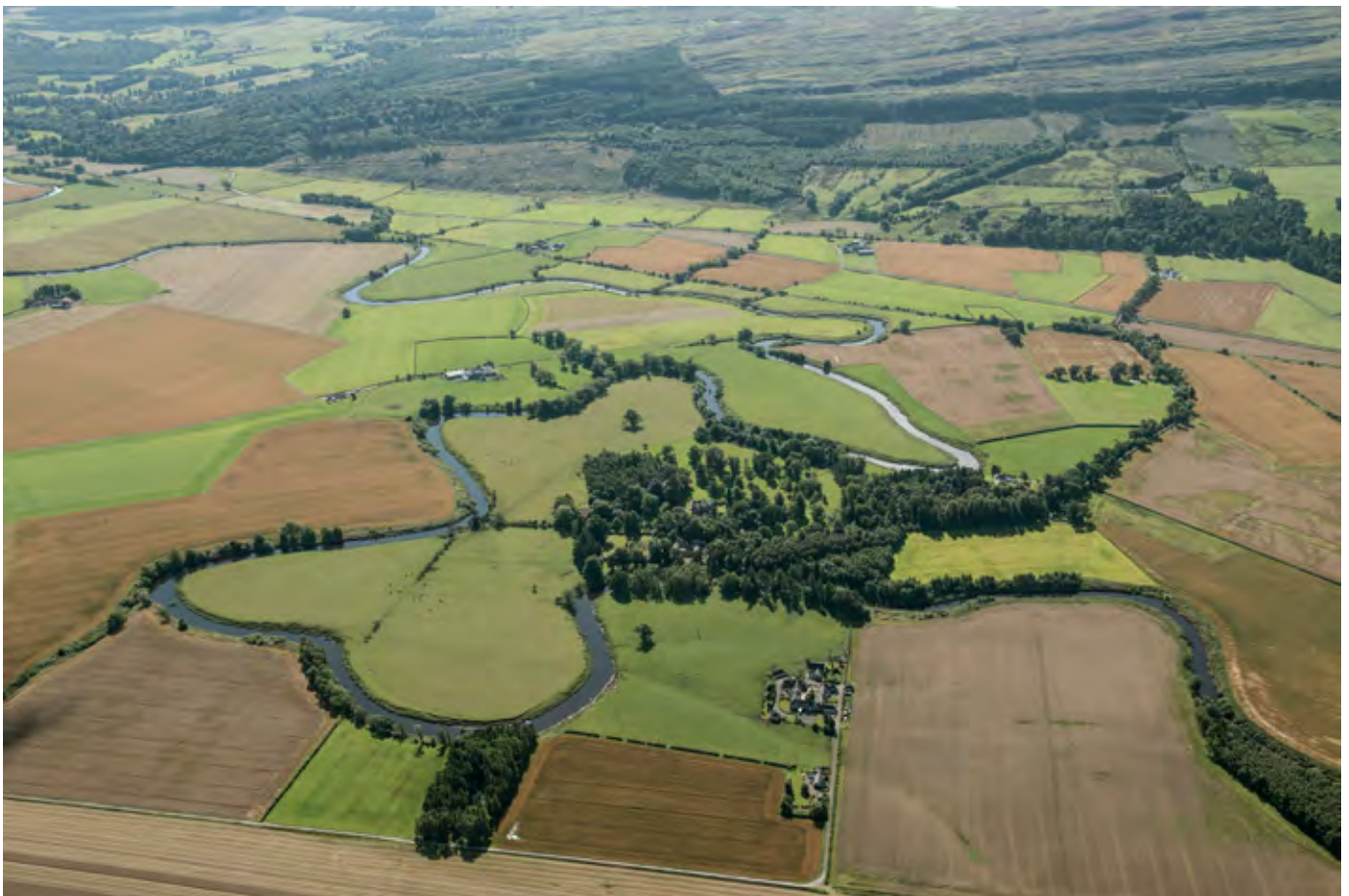
Fig 23 SEPA High-risk river-flood data indicates that Meiklewood House and its immediate policy woodland in a bend in the River Forth are not liable to flood, but much of the farmland along the river banks is. DP264767.
