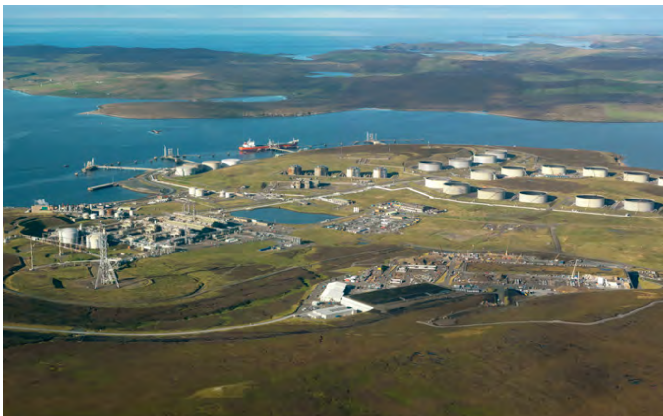
Fig 9 Sullom Voe Oil Terminal makes a significant impact on the landscape with its storage tanks. DP145855.
