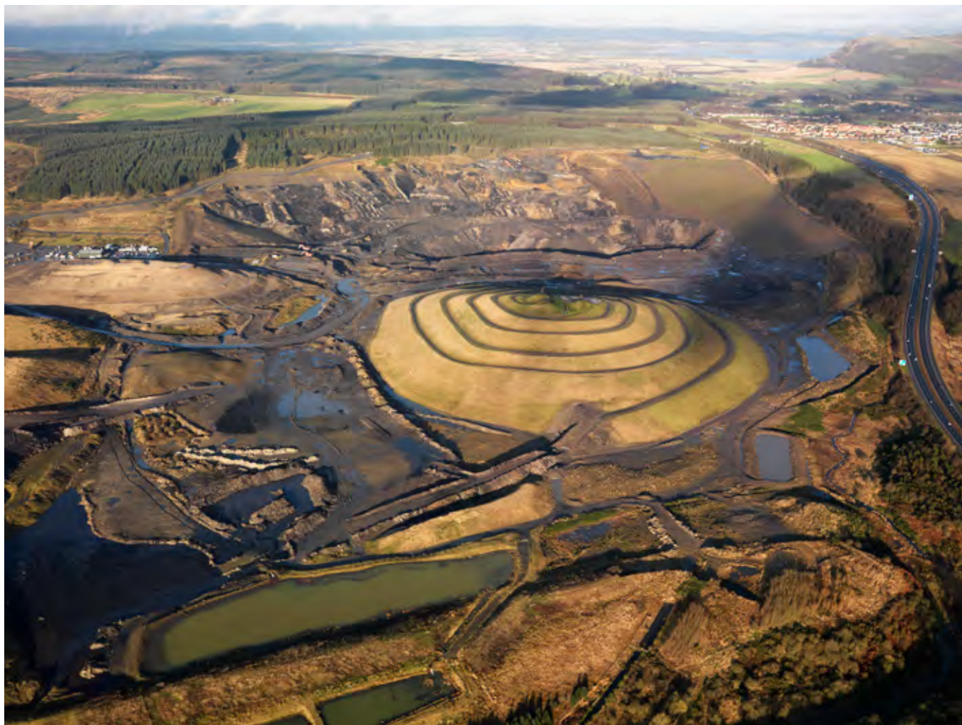
Fig 34 St Ninians opencast coal mine beside the M90 in Fife has been landscaped with an art installation by Charles Jencks but otherwise remains open, as do many others across the Central Belt. DP110945.
