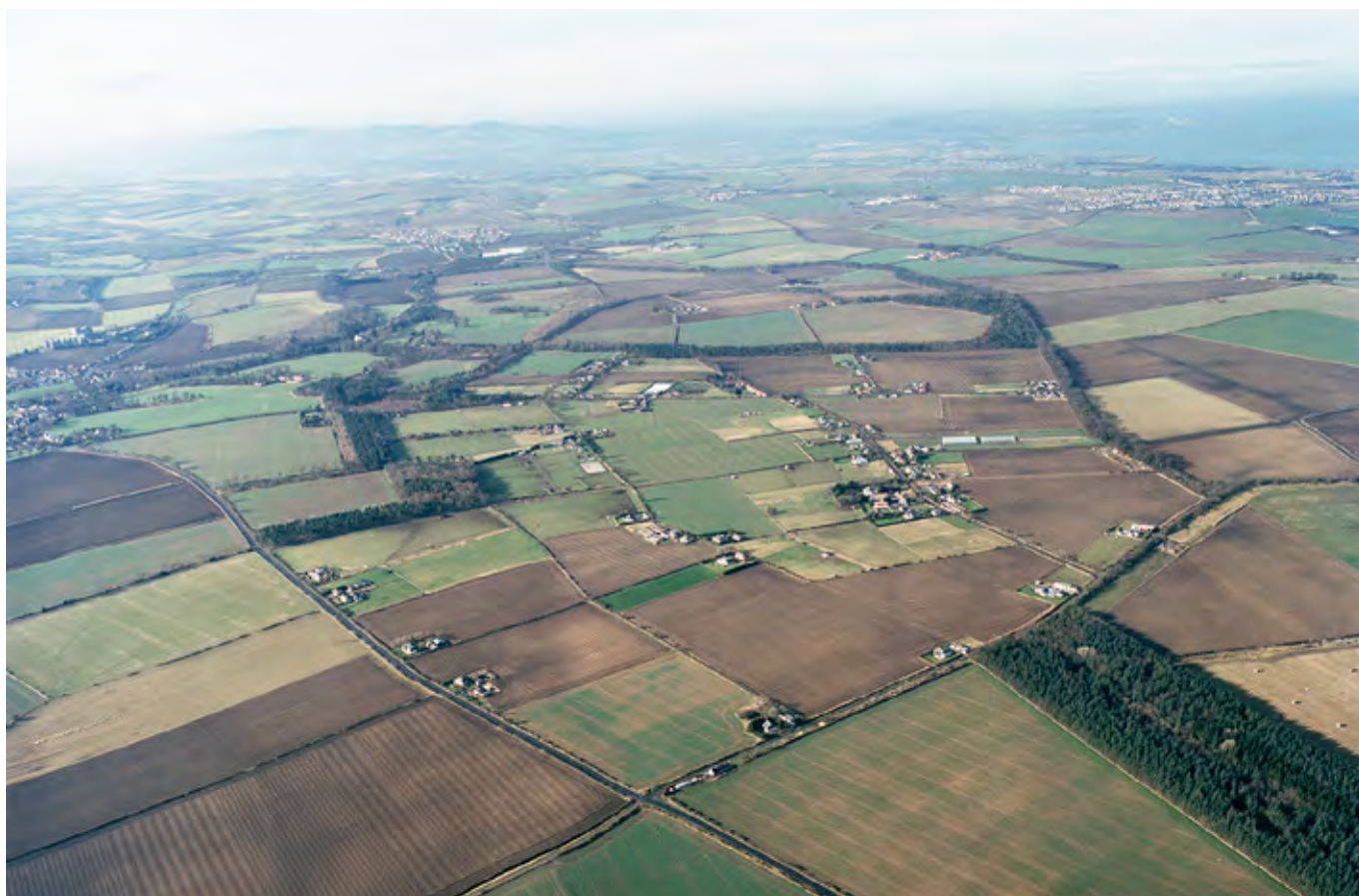
Fig 61 Homes fit for heroes, Boggs Holdings, East Lothian, carved out of an existing farm. SC968453.
