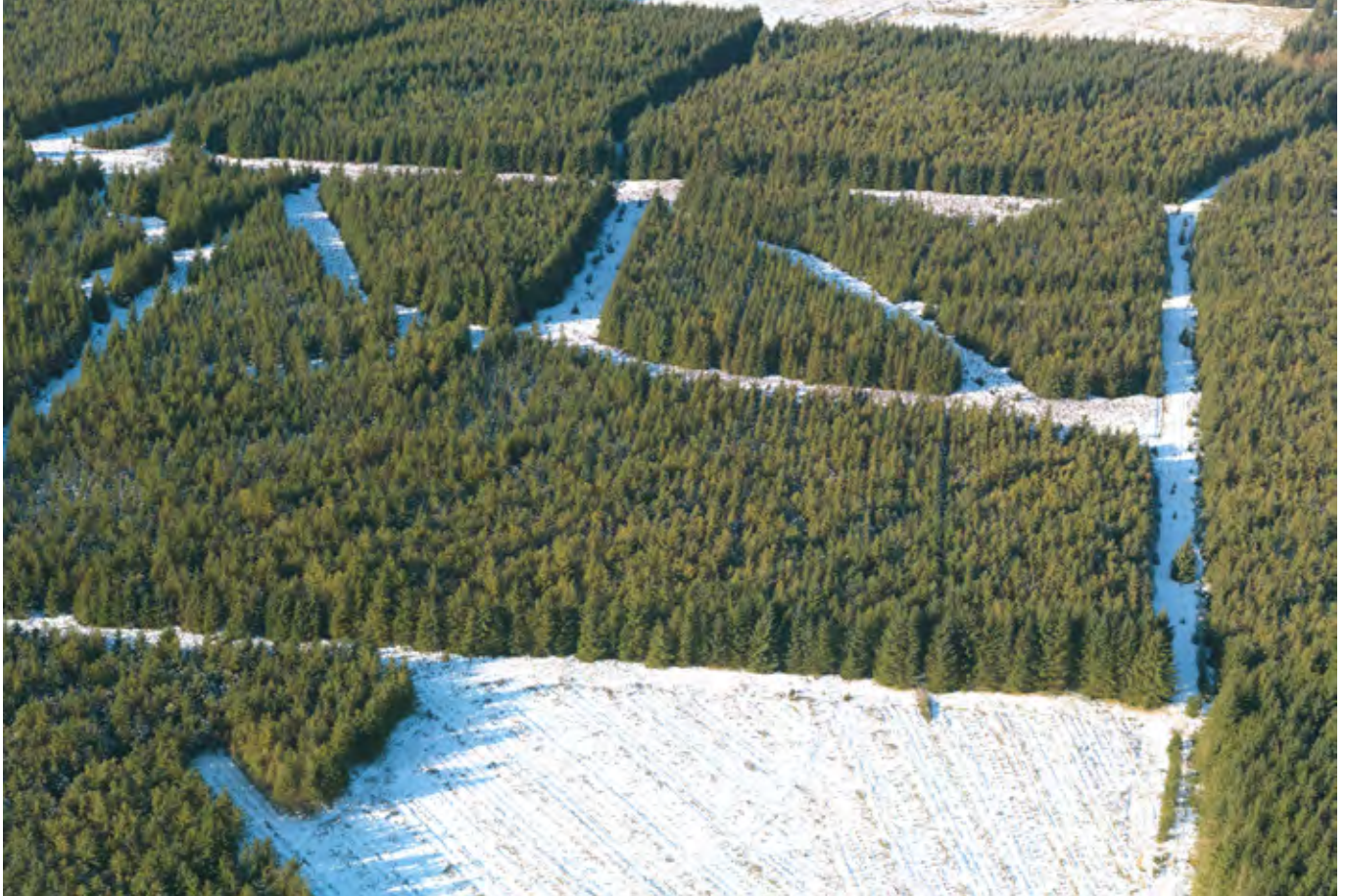
Fig 60 The straight edges of these conifer plantation at Harburnhead Hill, West Lothian typify pre-1989 plantings in which few concessions were made to amenity. DP055205.
