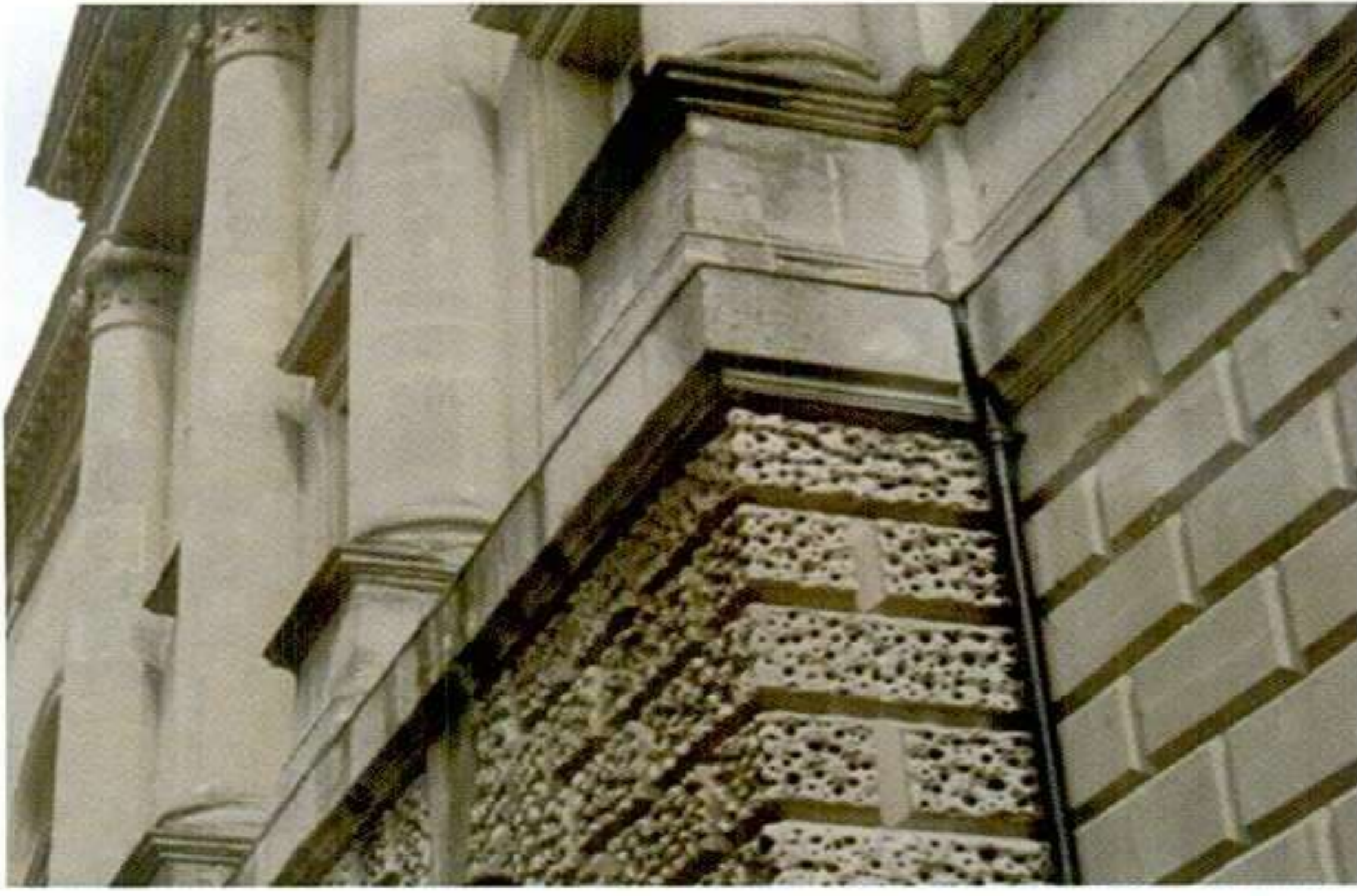
Varying degrees of soiling on Bath limestone surfaces and a similar variety of types of surface. Each type of limestone has its own properties and susceptibilities which need to be recognised when devising a cleaning regime.
