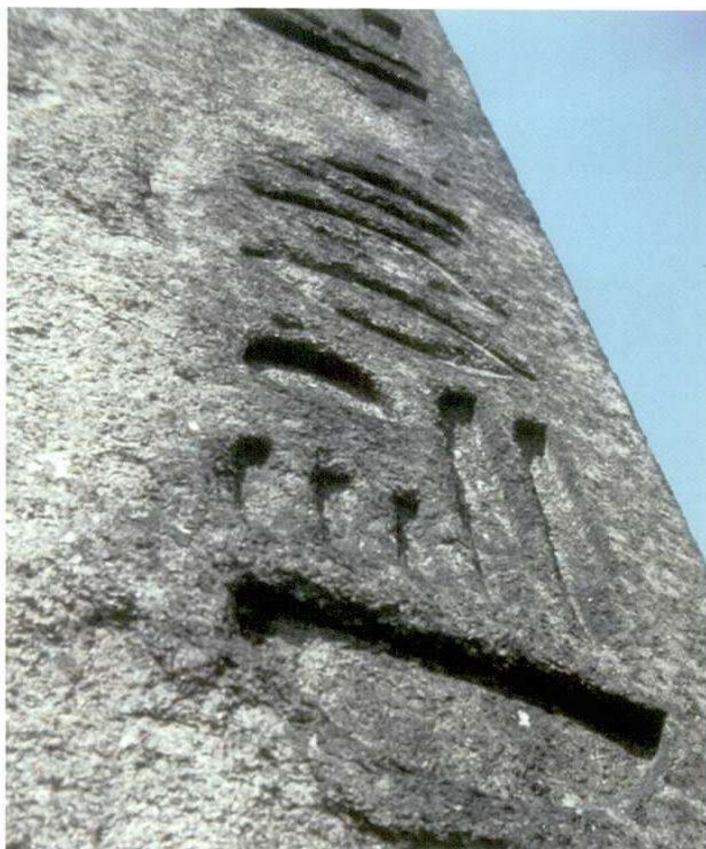
The granite of Cleopatra's Needle. London. The surface soiling is thin and superficial. This is confirmed in the petrographic thin section (Lithan Ltd for Adriel Consultancy). The thin section also shows the widespread micro fracturing of the granite, possibly due to the fires the obelisk was subjected to whilst still in Egypt.
