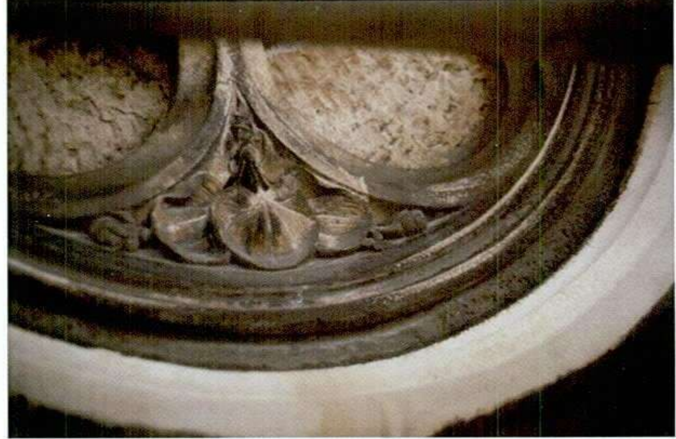
Varying degrees of soiling on Bath limestone surfaces and a similar variety of types of surface. Each type of limestone has its own properties and susceptibilities which need to be recognised when devising a cleaning regime.
