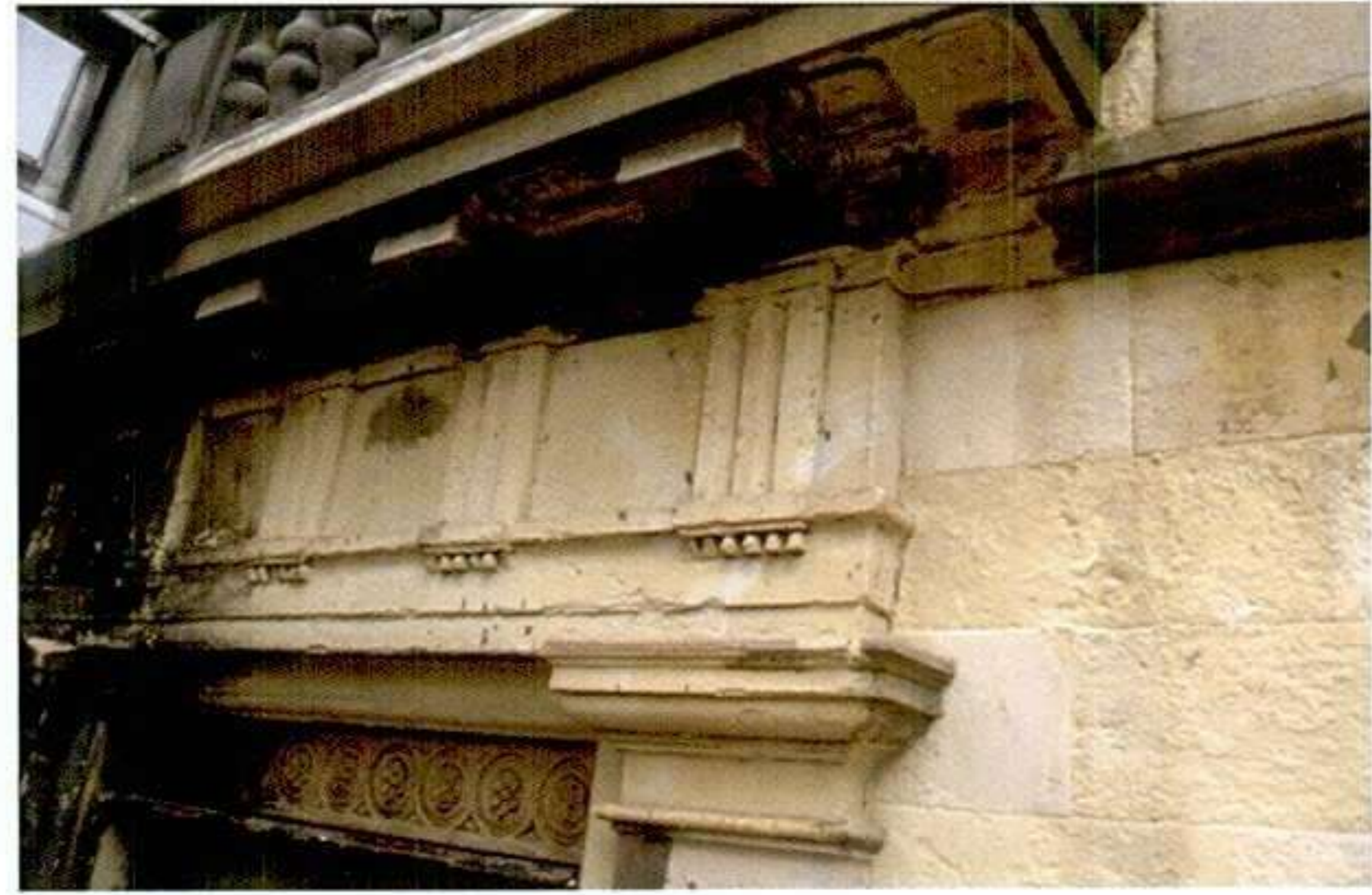
Caen limestone surfaces before and after trial cleaning. The soiling has been softened and removed by the water-based cleaning and the sulphated skin remains intact. Previous repairs in grey mortar have been uncovered.
