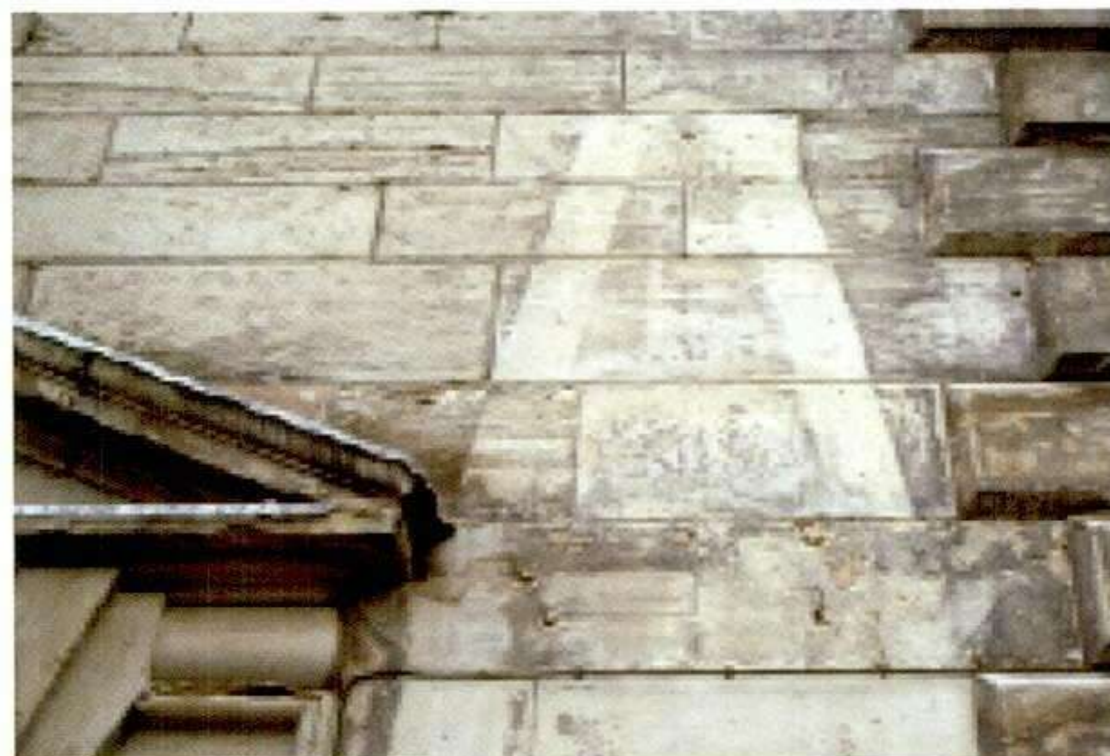
Above: A portion of this sandstone church in Birmingham has been protected by a family monument from decades of weathering and the subsurface changes that have developed elsewhere. The façade is “clean” despite its irregular appearance.
