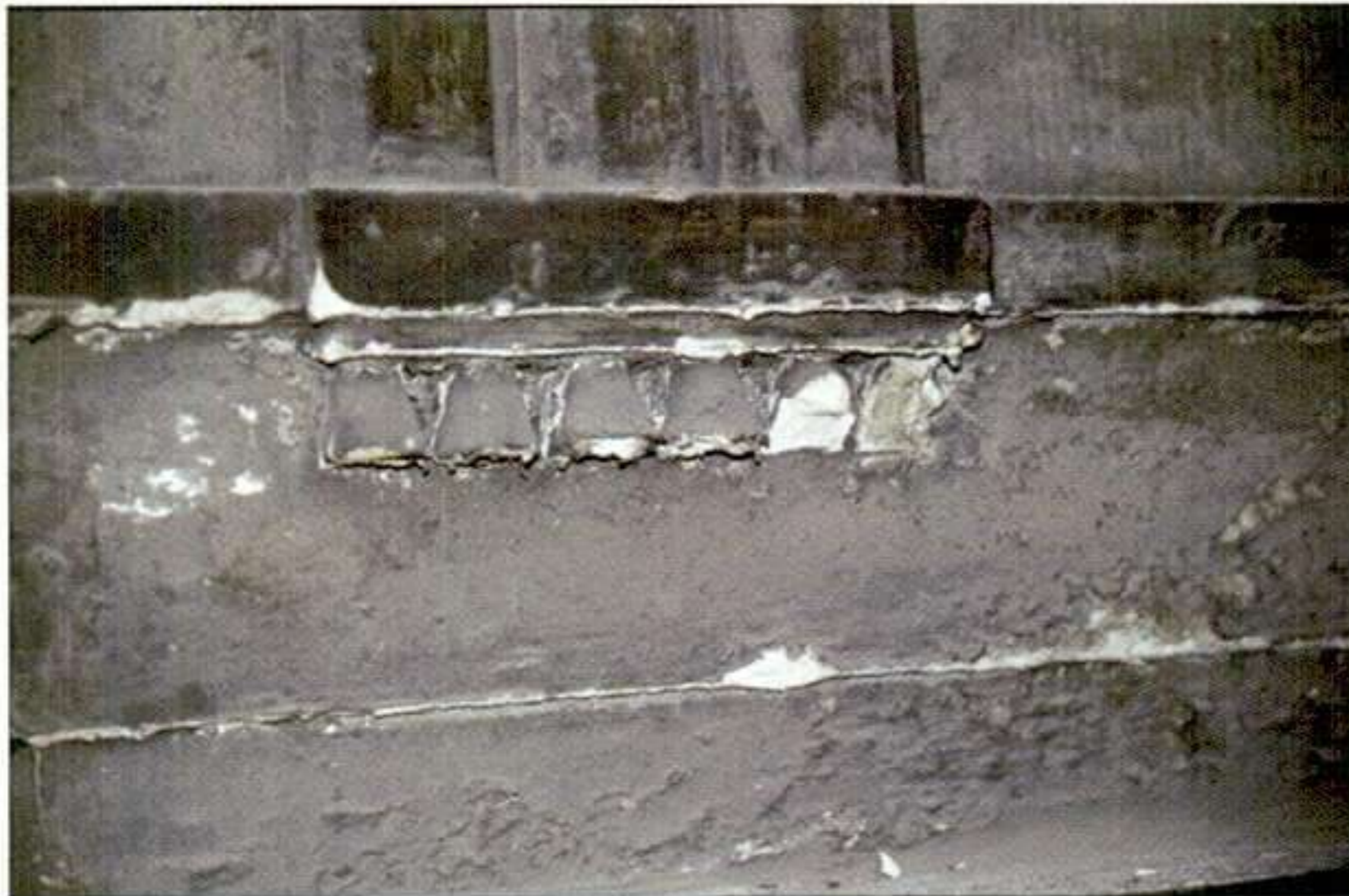
Caen limestone surfaces before and after trial cleaning. The soiling has been softened and removed by the water-based cleaning and the sulphated skin remains intact. Previous repairs in grey mortar have been uncovered.
