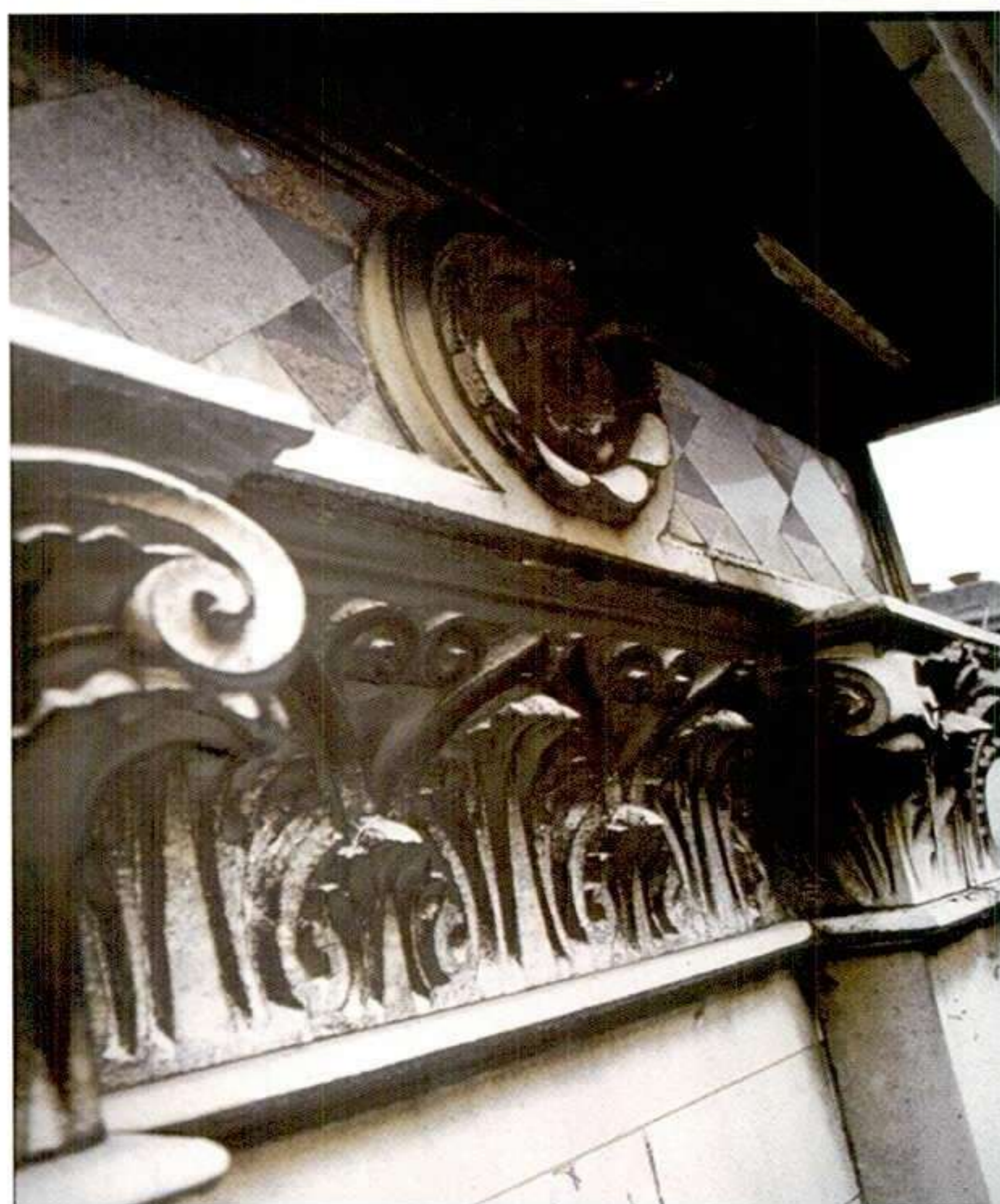
Above: A portion of this sandstone church in Birmingham has been protected by a family monument from decades of weathering and the subsurface changes that have developed elsewhere. The façade is “clean” despite its irregular appearance.
