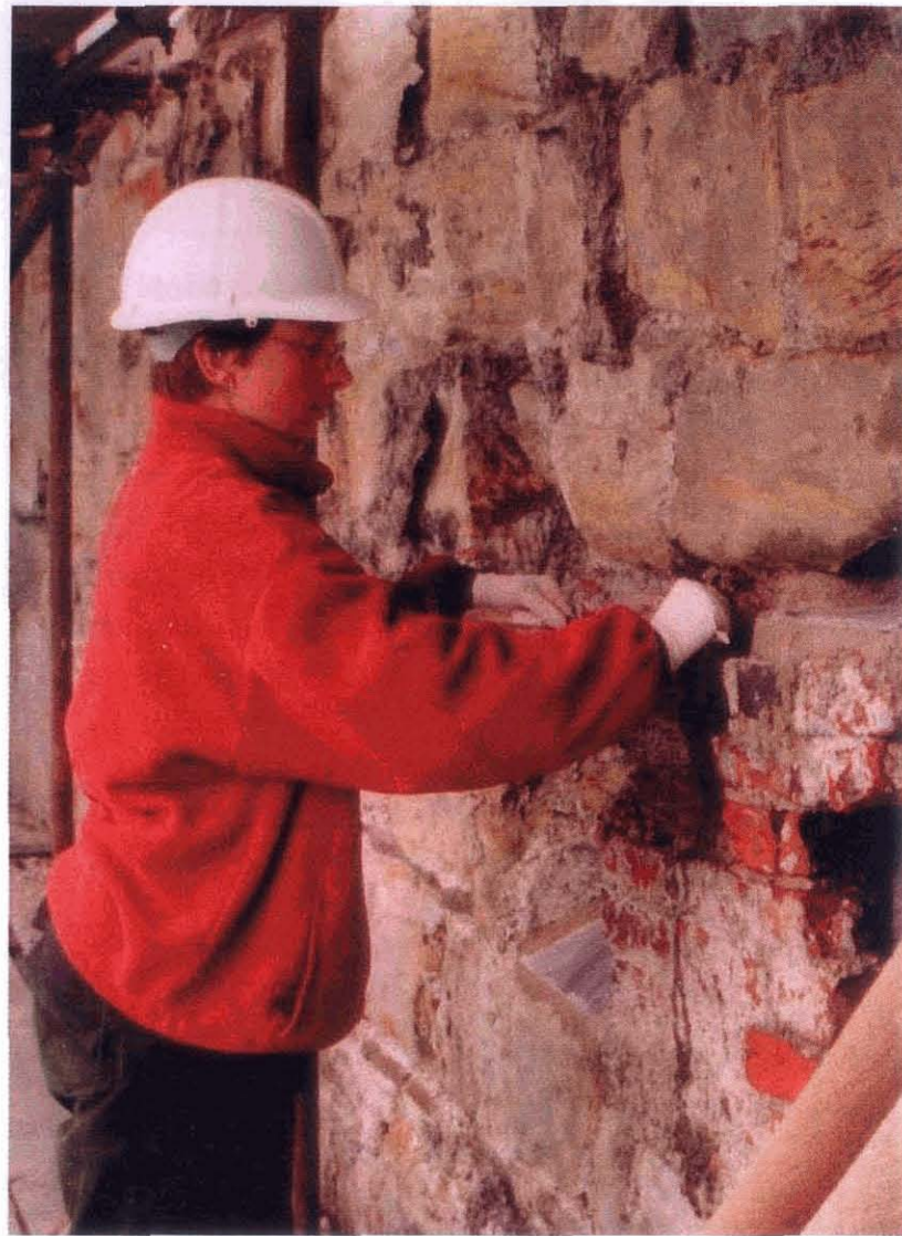
Figure 11.1 Conservation work on Kilns in progress (Copyright Scottish Lime Centre)
