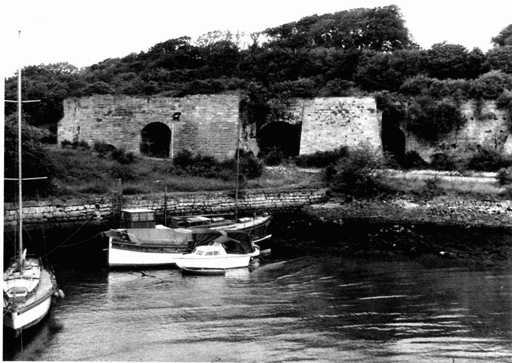
Figure 2 Kilns 11 & 12 from the harbour (Copyright Scottish Lime Centre)
