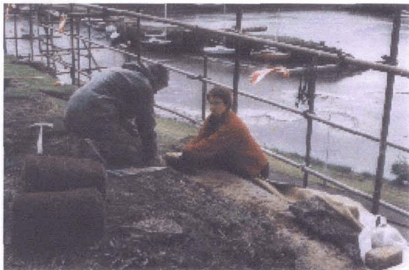
Figure 11.2 Conservation work on Kilns in progress (Copyright Scottish Lime Centre)
