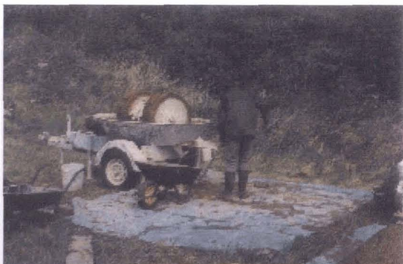
Figure 11.3 Conservation work on Kilns in progress (Copyright Scottish Lime Centre)
