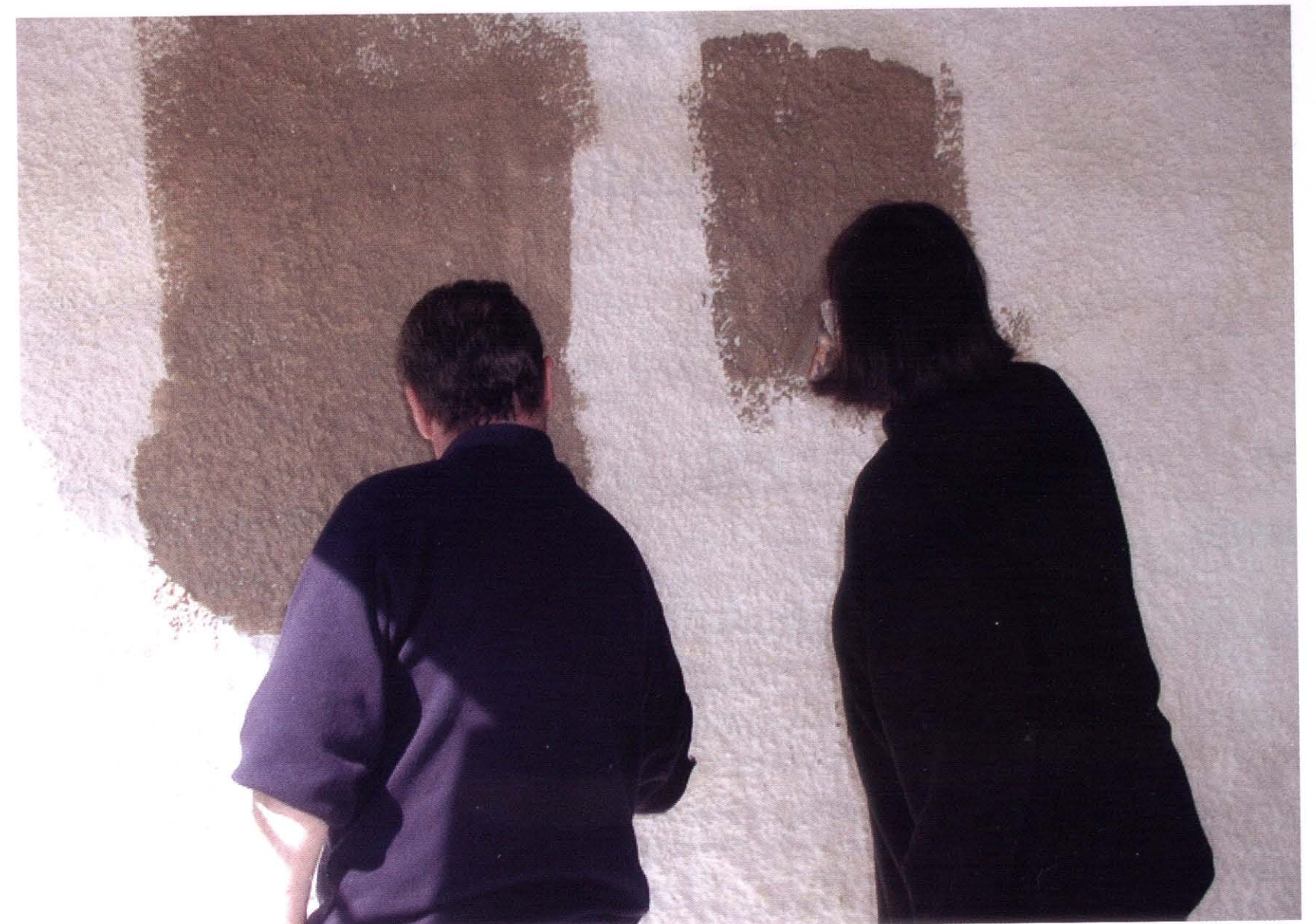
15.3 Applying limewash (Copyright Scottish Lime Centre)
