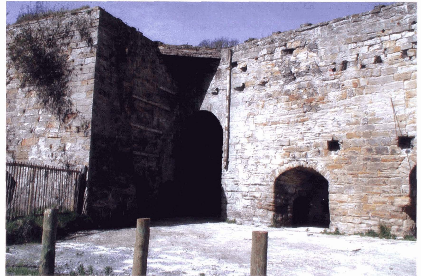
Figure 12 Kiln 11 after conservation (Copyright Scottish Lime Centre)
