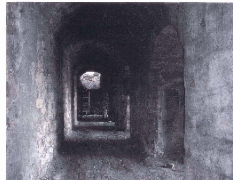
Figure 13 Vaulted passageway at rear of kilns (Copyright Scottish Lime Centre)
