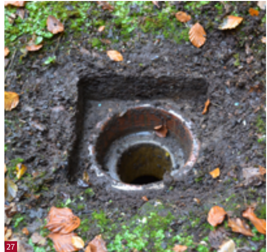
Fig. 26 Testing a gully and below ground drainage with a bucket of water.
