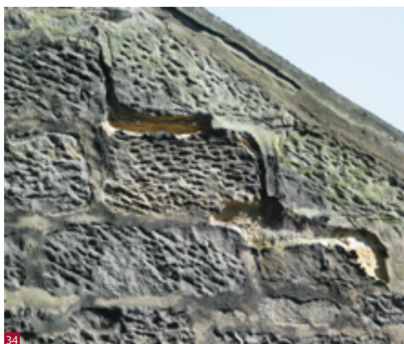
Fig. 34 Accelerated decay of masonry due to the use of the wrong mortar.
