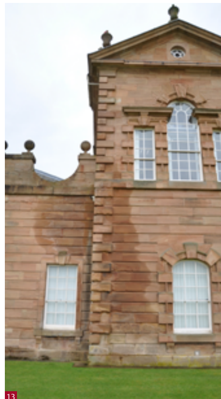
Fig. 13 Saturation of a wall due to a blockage in a parapet gutter.
