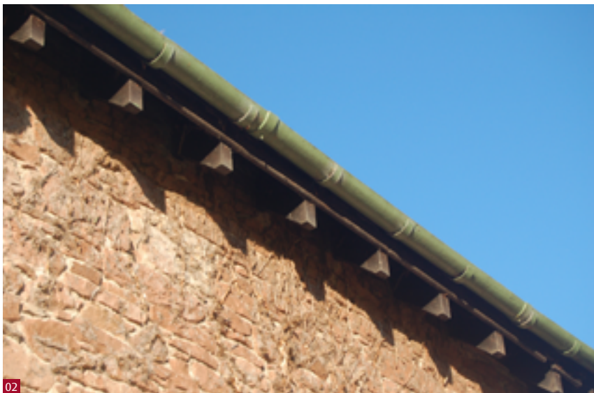
Fig. 2 Overhanging eaves on a 19th century building.
