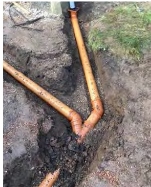
Figure 22. The new drain route from the southwest corner of the nave.
