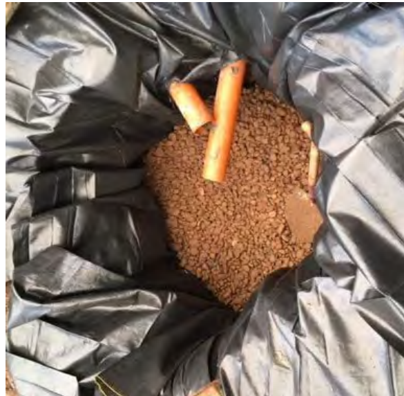
Figure 24. The soakaway pit lined and filled with gravel.
