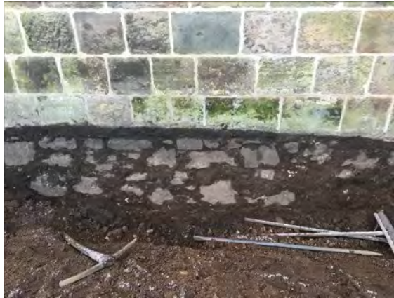
Figure 29. Newly exposed rubble on the north side of the nave.
