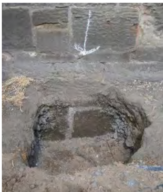
Figure 8. One of the investigation pits dug on the south wall of the nave.
