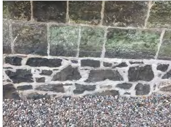
Figure 30. The masonry re-pointed using a quicklime based mortar.
