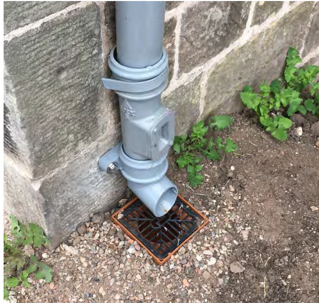
Figure 19. The new angled shoe directs water into the gully trap.
