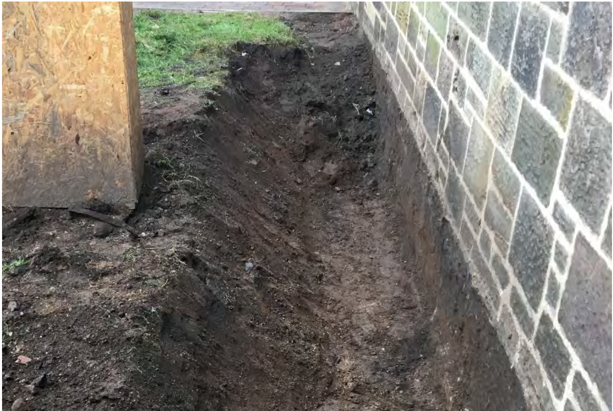
Figure 17. The newly dug trench along the south wall of the nave, where the base of an earlier wall can be seen. This restricted the depth of the excavation.
