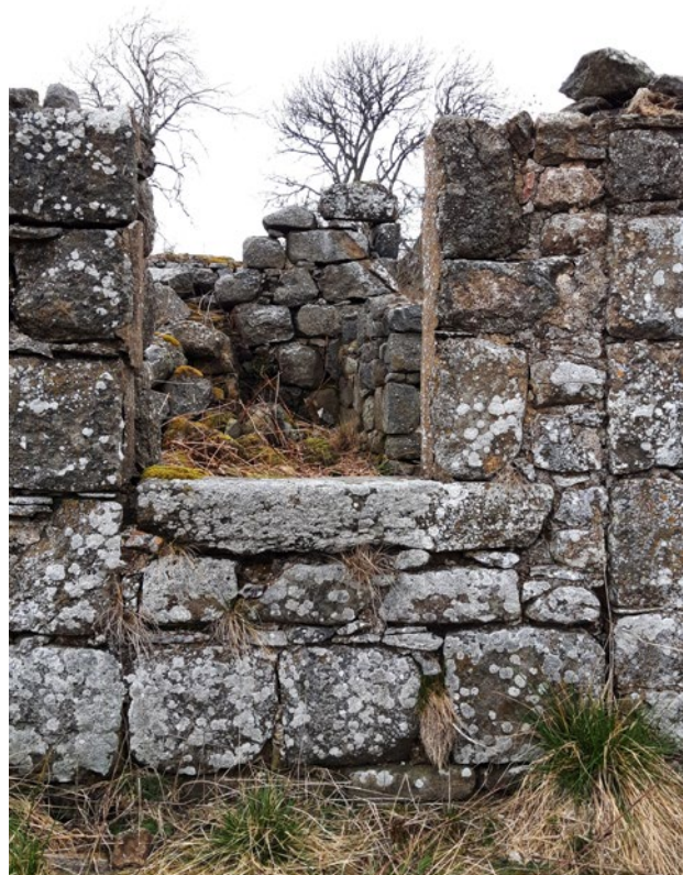
Remodelled entrance to the south-west end of Blackmiddens farmhouse. DP298673
