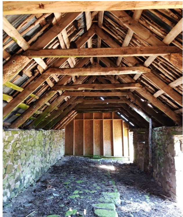
The roof of the byre at Blackmiddens exhibits the remains of a turf or peat sod covering, a rare surviving example in western Aberdeenshire of this alternative to thatch or slate. DP298625
