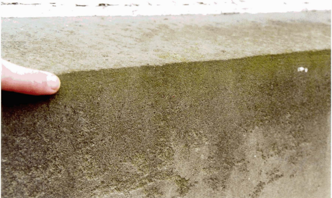
Plate 6 Preferential colonisation of roughened surface of sandstone.
