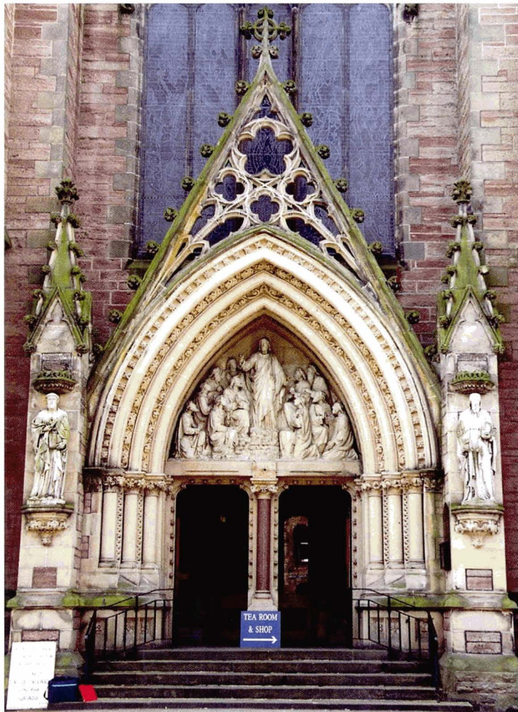
Plate 11 Heavy biological growth on run-off zone and on carved detail. Black soiling at edge of the zone is typical of gypsum crust formation on calcareous sandstone.
