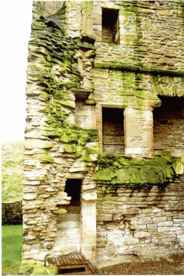
Plate 1 Typical example of algal colonisation of sandstone wallheads, ledges and splash zones at Crossraguel Abbey.
