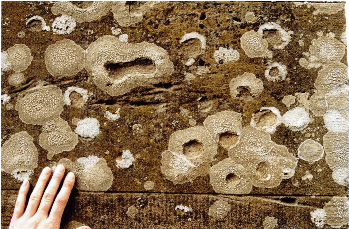
Plate 3 Example of lichen damage to sandstone. Note the formation of erosion pits at the centre of the growths.
