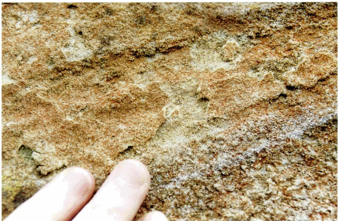
Plate 2 Example of decay of sandstone by the alga Trentepohlia. Note the orange coloration of the growths.
