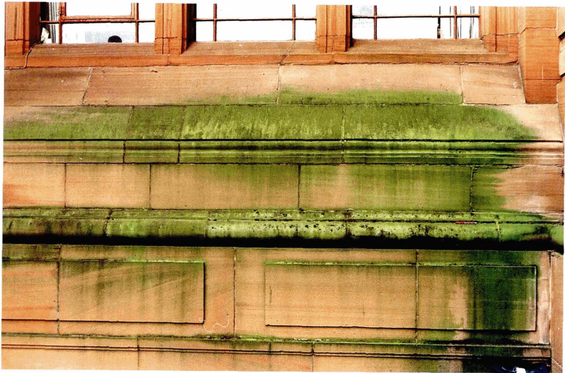
Plates 7 & 8 Rapid colonisation of red sandstone after chemical cleaning. Note preferential soiling of sills and run-off zones.
