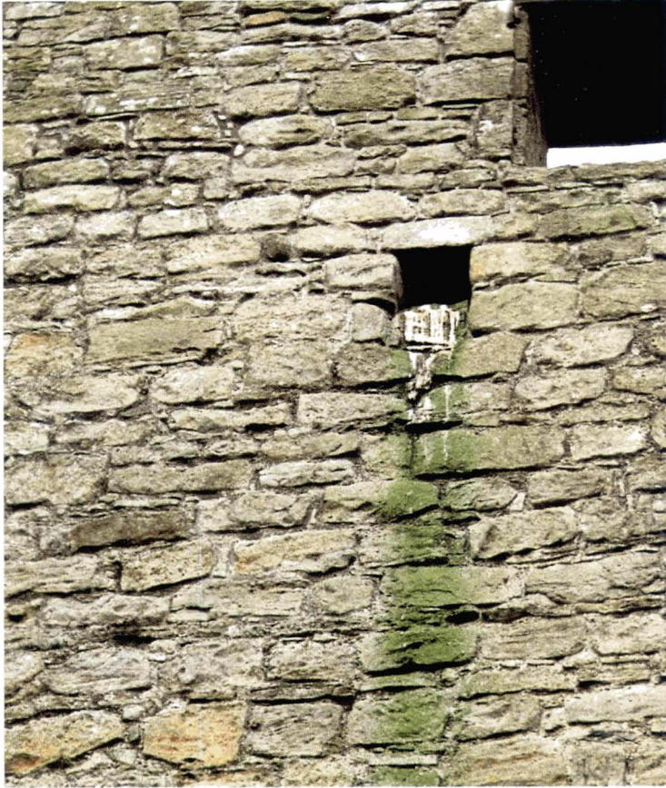
Plate 9 Preferential biological colonisation below opening used as an owl's nest site at Hermitage Castle.
