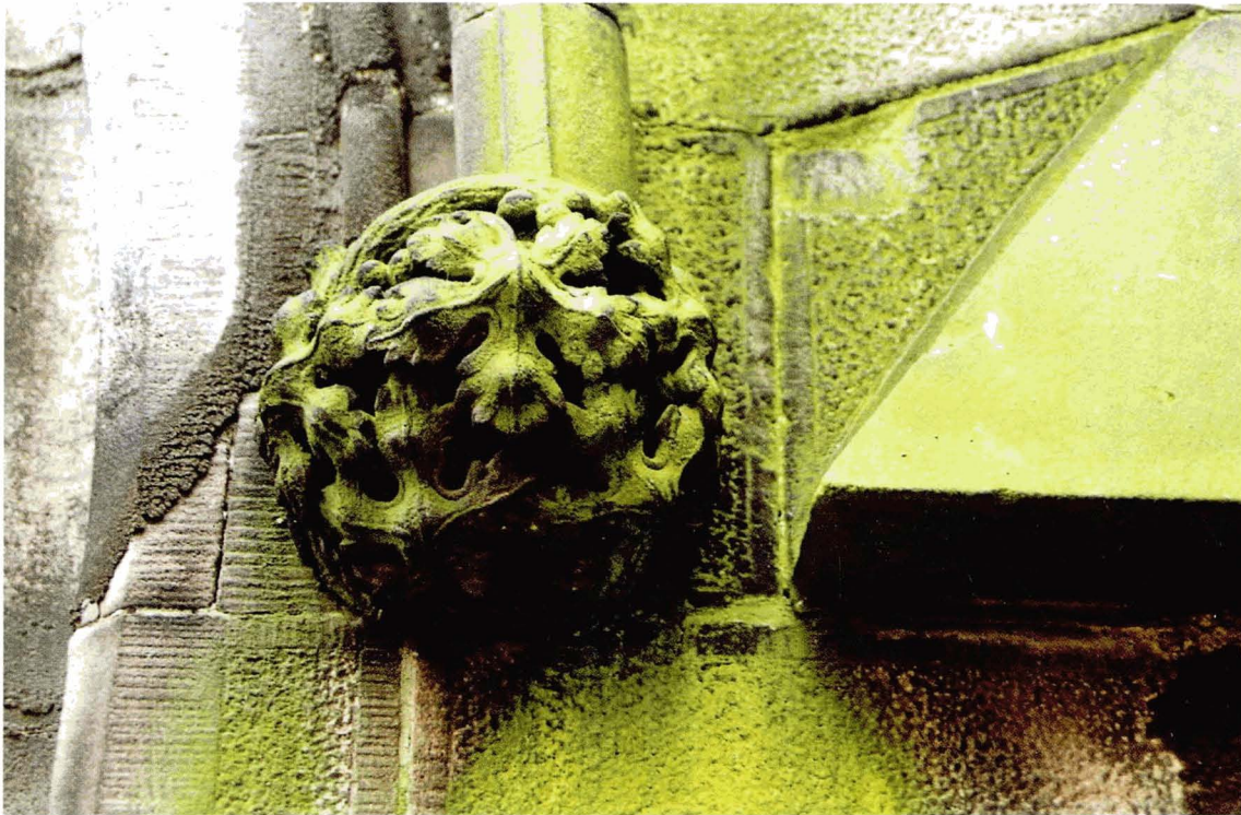
Plate 11 Heavy biological growth on run-off zone and on carved detail. Black soiling at edge of the zone is typical of gypsum crust formation on calcareous sandstone.
