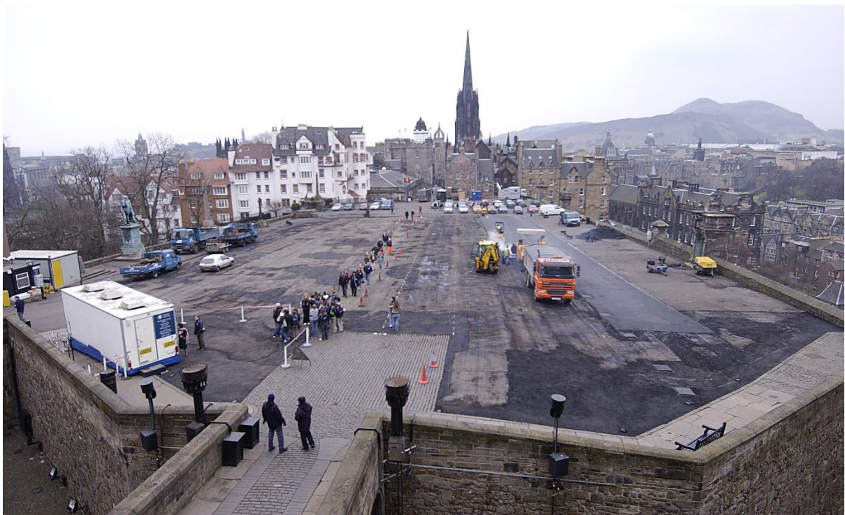
Figure 7: Resurfacing works being undertaken on the Esplanade. © Crown Copyright HES.
