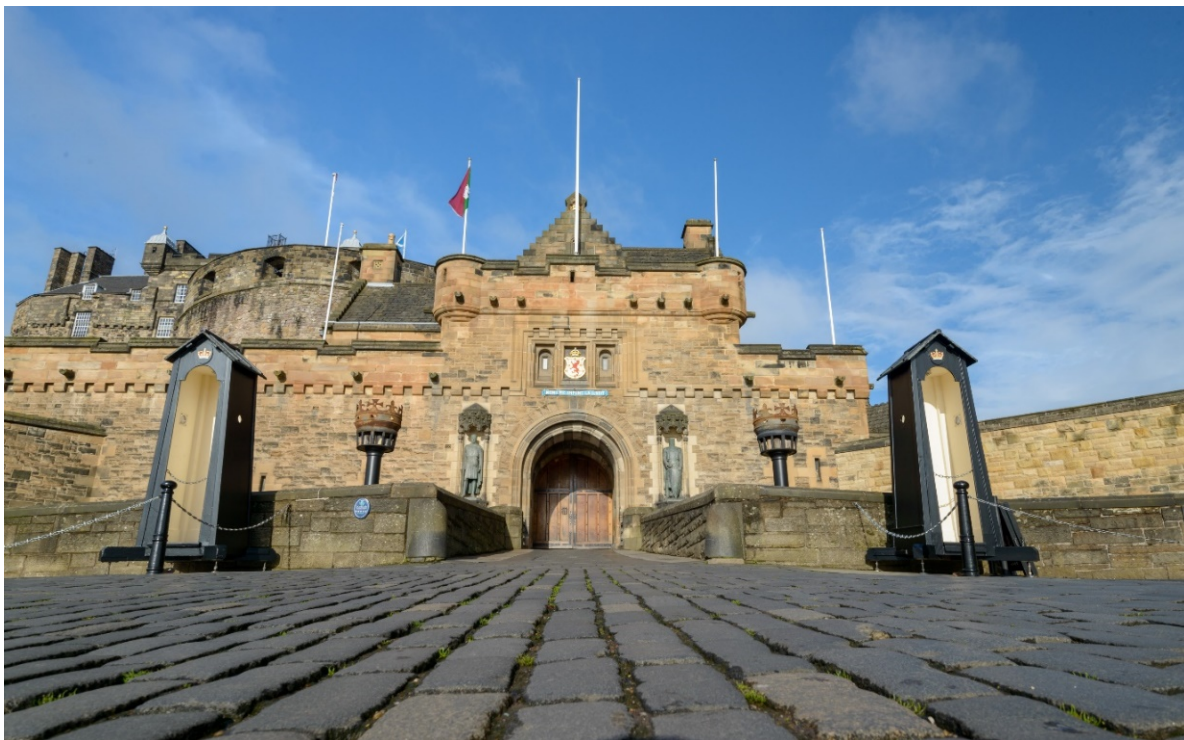
Figure 10: View of approach to gatehouse, from Esplanade. Note setts on ground, and sentry boxes either side of the narrow walkway (a fixed bridge leading over the dry ditch) © Crown Copyright HES.
