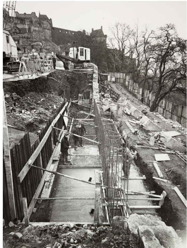
Figures 5 & 6: North wall of Edinburgh Castle Esplanade, before and during reinforcement works. (left) 1966, looking east (right) 1967, looking west. Both images © Crown Copyright: HES.
