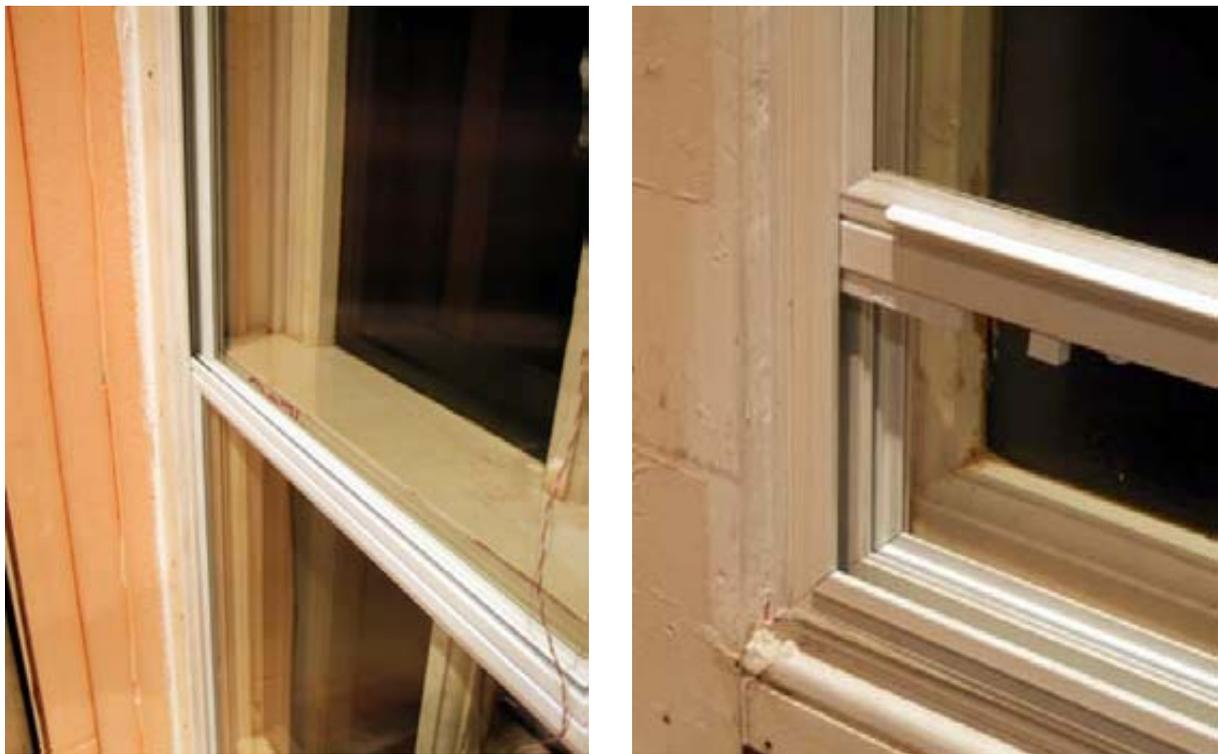
Figure 2 Secondary glazing installed to single-glazed sash & case window on the room side: the left photo shows the meeting rails, the right photo the bottom of the window.
