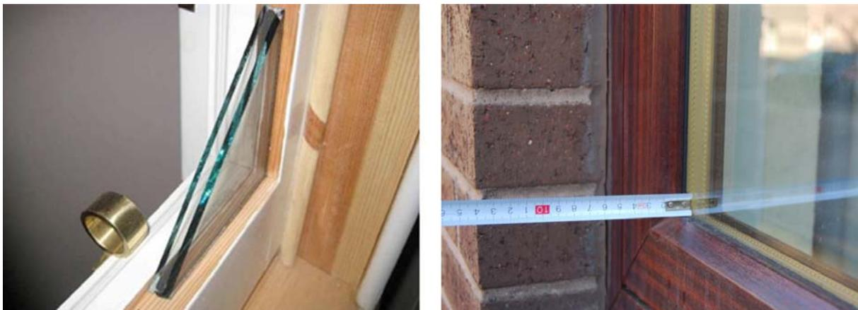
Figure 1 Slim-profile double glazing (left photo) has a slimmer cavity, and therefore overall thickness, than conventional double glazing (right photo).
