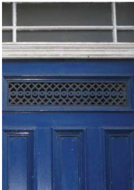
Ventilation grille in a late 19th C tenement door.
