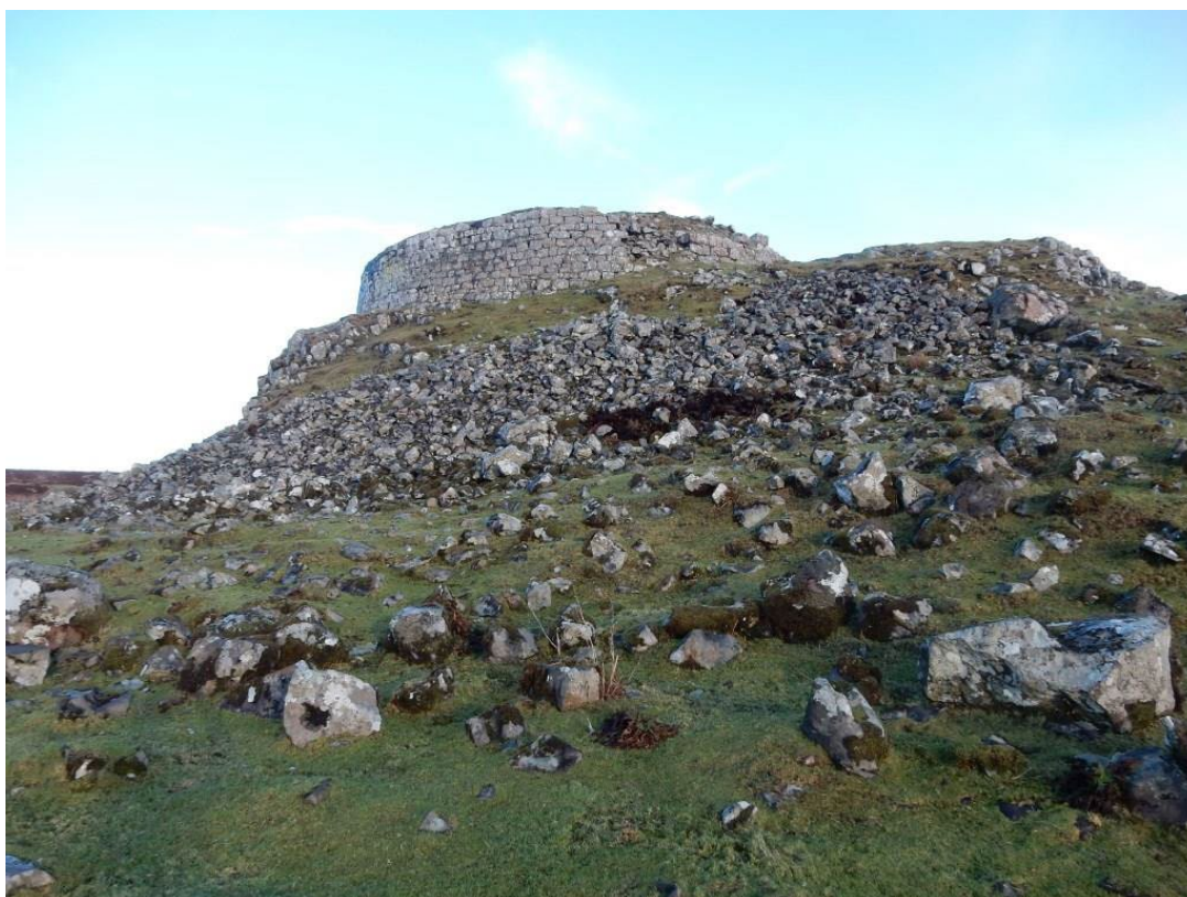
Figure 17: Dun Beag, south-west sector, showing collapsed masonry ©Ann MacSween
