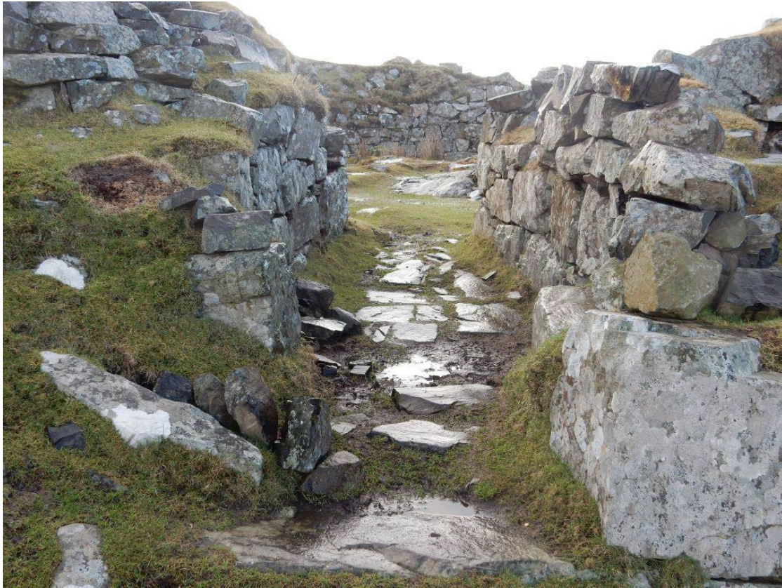
Figure 8: Dun Beag, looking along entrance into courtyard ©Ann MacSween
