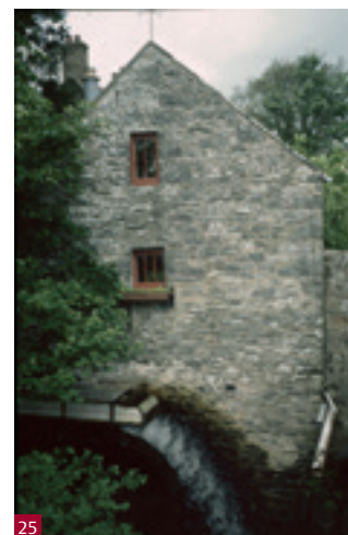
Fig. 25 A former corn mill in the Scottish Borders where a waterwheel was re-introduced to power a pump for a ground source heat system. The historic mill pond, weir (caul), lade and wooden launder (trough) were all reused to drive the new wheel.
