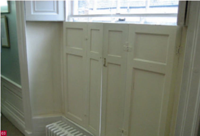
Fig. 3 Keeping shutters closed is a simple, inexpensive way to retain heat in older properties.
