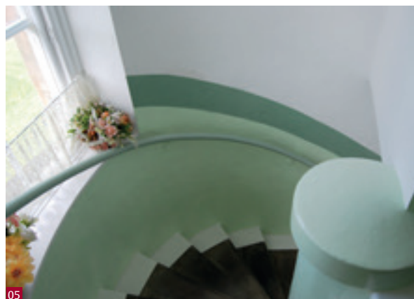
Fig. 5 A blanket of aerogel insulation was applied to the internal face of the stone wall of this stairwell, and plastered over.
