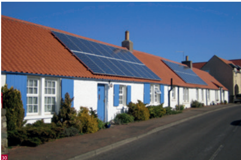
Fig. 30 Solar panels initially installed on one cottage affect this entire streetscape in East Lothian as the installation has encouraged other residents to make similar installations.
