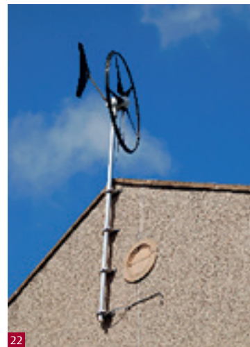
Fig. 21 Westray Parish Church, Orkney (Category C-listed). The 6kW turbine is far from the building, thus in an exposed position and reducing the visual intrusion to the setting.
