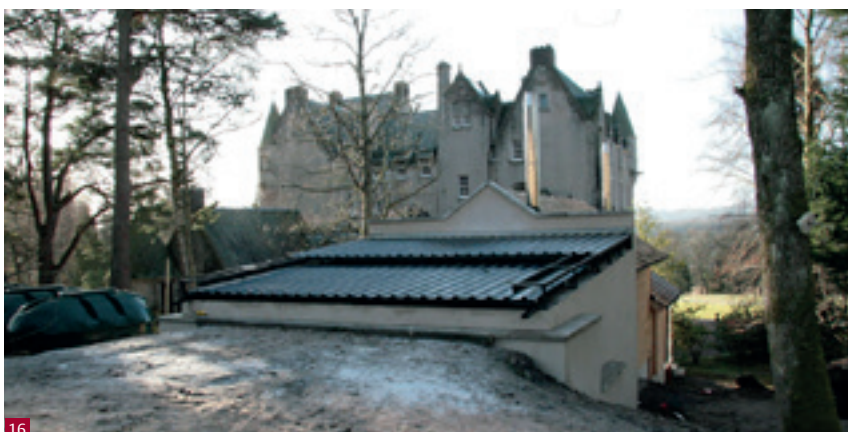
Fig. 16 Fuel store for a biomass boiler serving Kincardine Castle, Aberdeenshire. This small storage facility is refilled from a larger shed located further away. This storage shed has been built behind a timber dog kennel, and is hardly visible from the castle.
