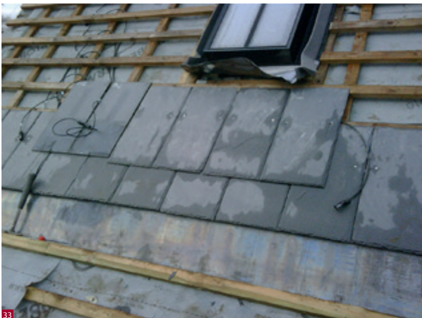
Fig. 33 Solar PV tiles designed to look like slate are integrated into a slate roof during refurbishment works (© Solar Slate www.solarslate-ltd.com ).
