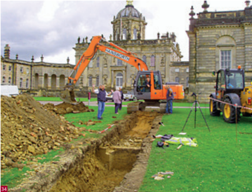
Fig. 34 Installation of Ground Source Heat Pump (GSHP) at Castle Howard. An archaeologist supervised all necessary ground disturbance during the work, during which a revetment wall was uncovered (© Hon. Sir Simon Howard/Castle Howard Estate Ltd).
