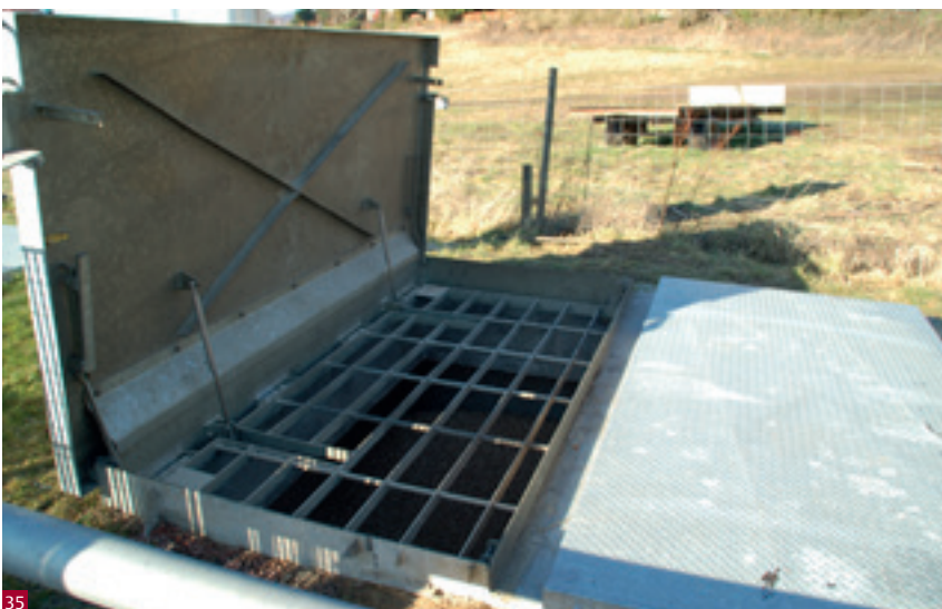
Fig. 35 Biomass fuel storage silo, Rosslyn Chapel. The large underground pellet silo allows for easy deliveries from the supplier.
