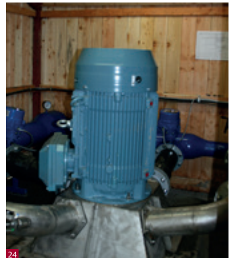
Fig. 24 Electricity being generated at the turbine house at Balbeg Country Holidays' self-catering cottages, Ayrshire. Excess is exported to the National Grid (© Energy Saving Trust).
