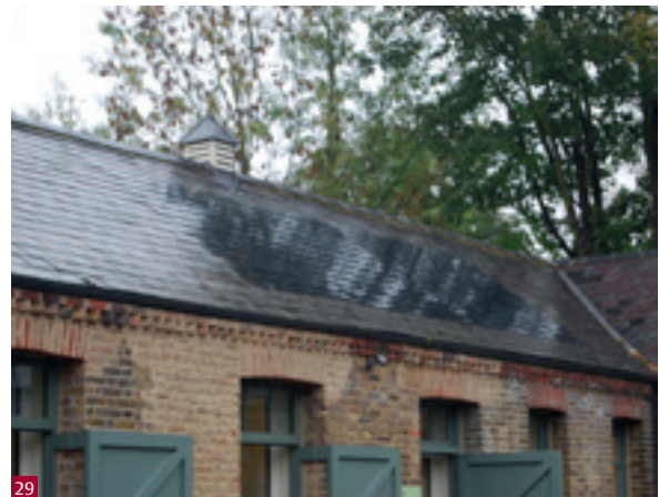
Fig. 29 Solar tiles at Morden Hall Park, London, attempt to mimic the appearance of slates.
