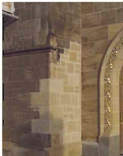
Different stone types can be successfully combined where there are no incompatibilities in their composition with respect to stone performance
