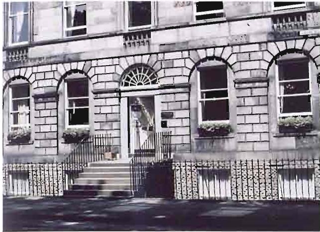
Above Typical arrangement of rock-faced, rusticated and polished ashlar in pale-coloured Craigeith sandstone, the New Town of Edinburgh. (A A M'Millan)
