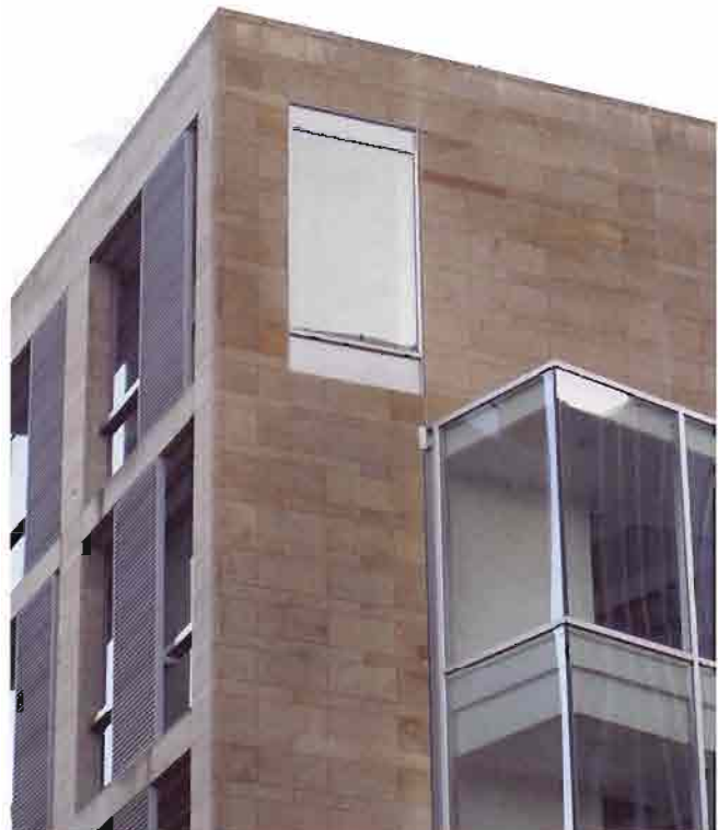
Joints are filled between the carefully proportioned courses of Blaxter's stone cladding on Evolution House by Reich and Hall Architects in Edinburgh's Westport.
