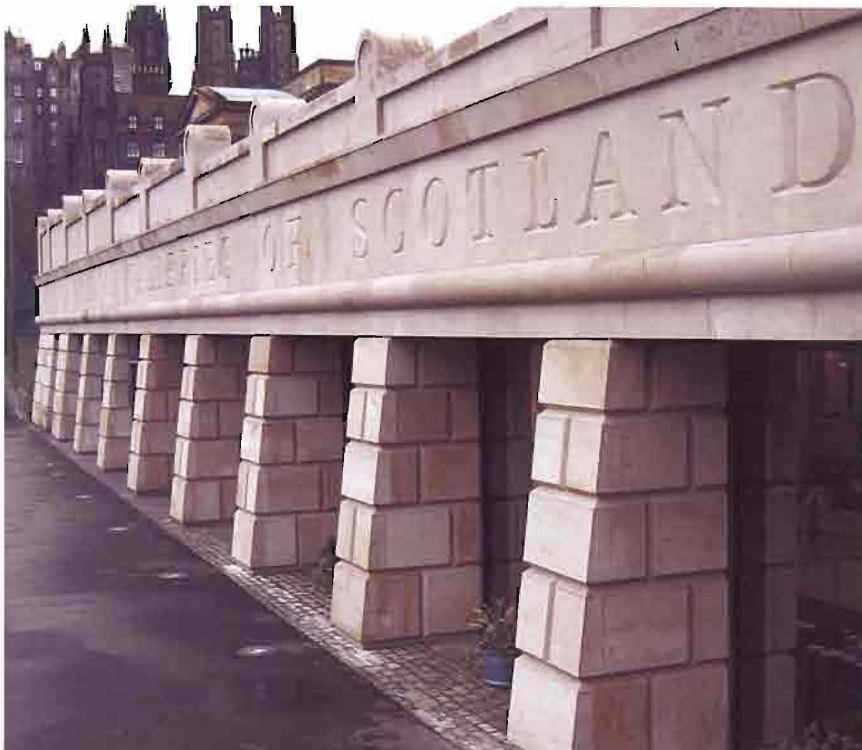
Weston Link by John Miller & Partners uses Light Clashach Sandstone to form a battered, rusticated entrance wall.
