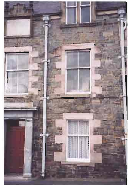
A 19th century greywacke constructed building in Earlston. Note pink sandstone quoins and lintels. (A A McMillan)
