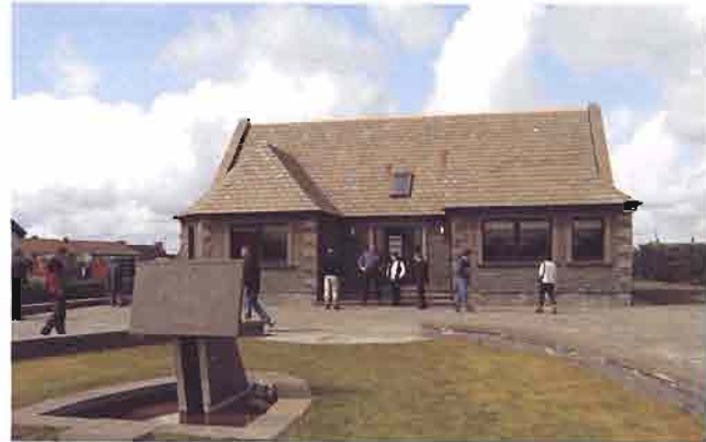
Devonian house, Halkirk, Caithness. A new property built entirely out of local Caithness flagstone. (A A McMillan)
