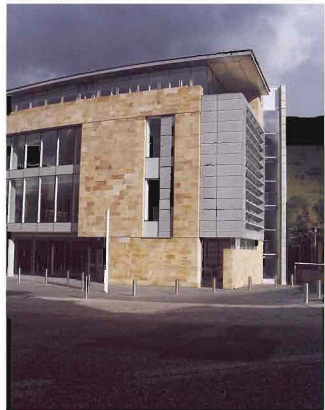
Holyrood Park House by architects CDA uses Clashach sandstone to good effect on its principle façade and demonstrates the suitability of this stone type to high quality commercial buildings.
