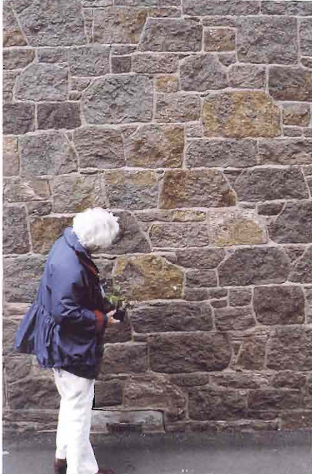
Warm weathering colours in trachyte, a locally quarried igneous rock, used here in a 19 th century building in Haddington, East Lothian. (A A McMillan)
