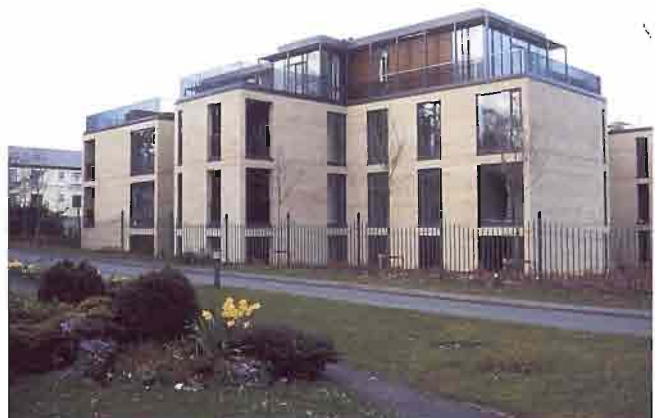
Hand-set cladding on a luxury apartment building in Edinburgh's Murrayfield area. Reiach and Hall Architects used Peakmoor ashlar on the exterior of Succoth Heights.
