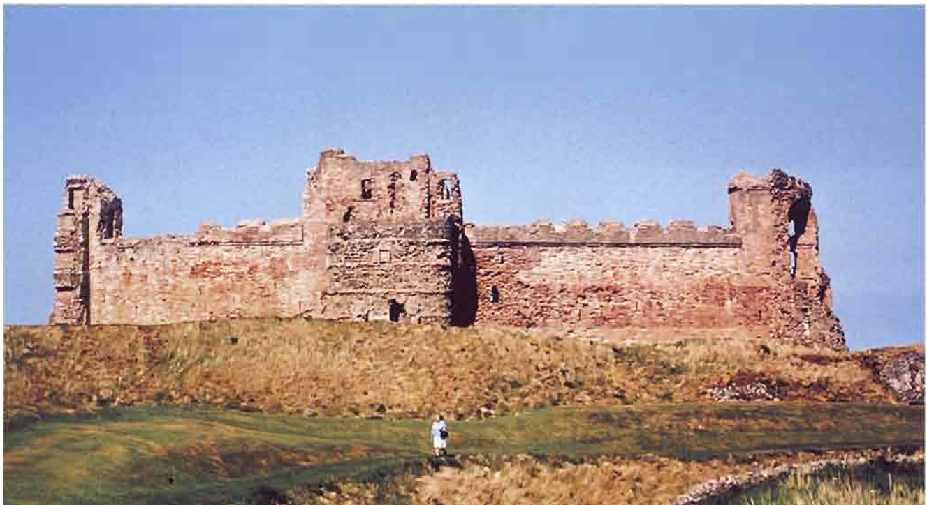
Below Tantallon Castle. Defensive curtain forewall viewed across outer ditch
