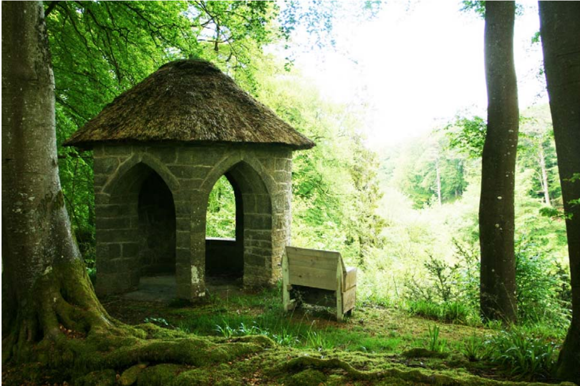
Rustick Hut (above Habbie's Howe), Newhall House, Penicuik, late 18 th century (LB14647)
