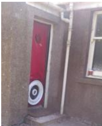
Fig. 4 Blower door fitted to test for air-tightness
