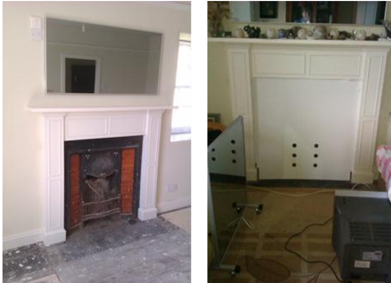
Fig. 27 Living room fireplace showing temporary board fixed into place.
