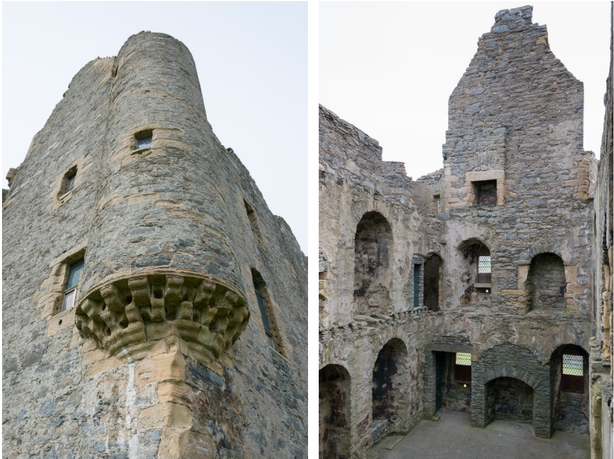
Figure 9 (Left): North-east turret rising from first floor to upper floors. Chequer-set corbels with shotholes between, resembling those of Munness Castle, Unst. The glazing is modern, installed in the 1980s. Figure 10 (Right): Interior of the main block of Scalloway Castle: the hall fills the whole of the first floor. This view shows the fireplace and two windows on the east end. The flooring of the upper storeys has not survived. Large patches of plaster are visible on the walls on the left-hand side of the image. Both © Crown Copyright HES.
