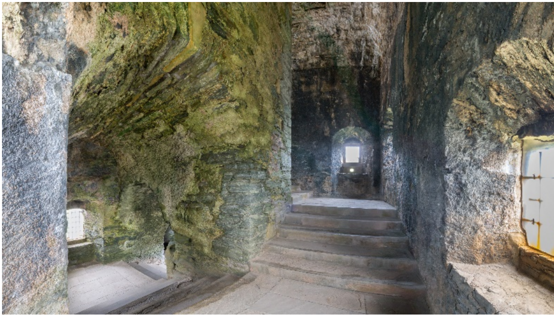
Figure 8: The scale-and-platt stair rises to the first floor. © Crown Copyright HES.
