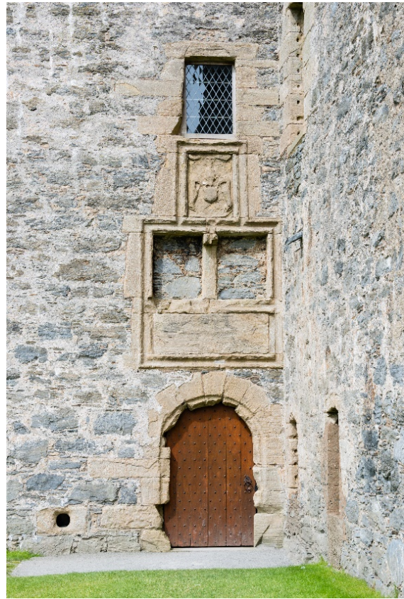
Figure 4 (Left): Detail of circular gunloop, identical to those on Muness Castle, Unst. Image taken prior to the installation of modern glazing.
