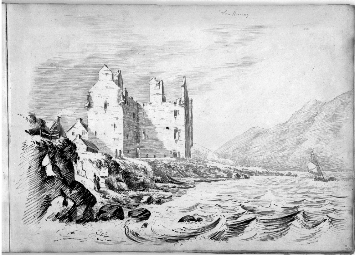
Figure 13: 1801 drawing of Scalloway Castle; by this stage ruinous. Walter Scott would later describe the 'rifted walls and dismantled battlements giving unrestrained access to the roaring seablast'. © Courtesy of HES.
