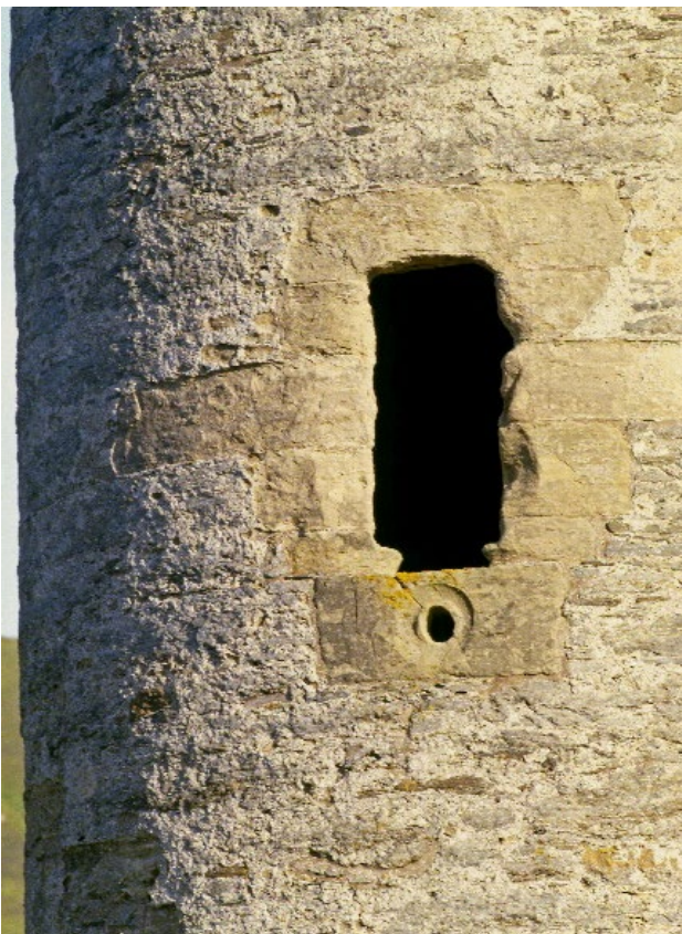
Figure 4 (Left): Detail of circular gunloop, identical to those on Muness Castle, Unst. Image taken prior to the installation of modern glazing.
