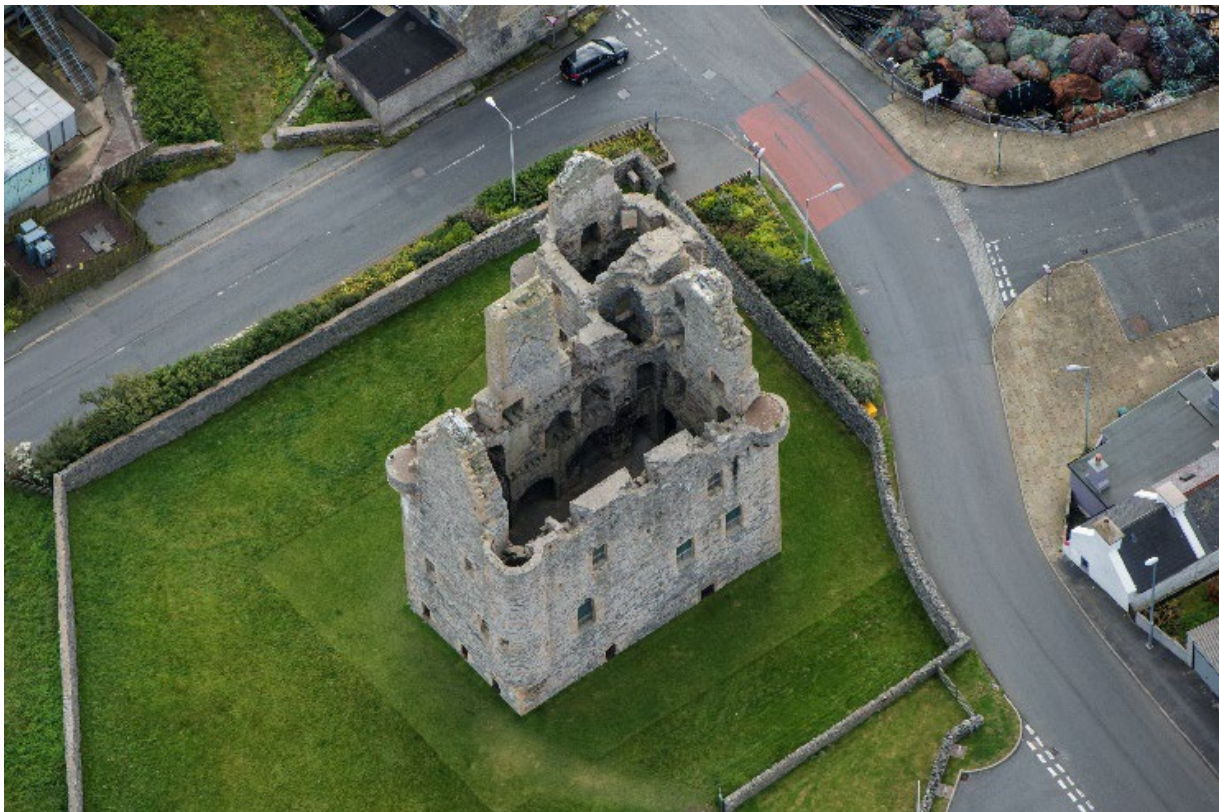
Figure 15: oblique aerial view of Scalloway Castle. The presence of the stair turret in the north-east corner (bottom centre of image) may suggest that a second jamb was intended at this point to create a Z-plan form. © Historic Environment Scotland.
