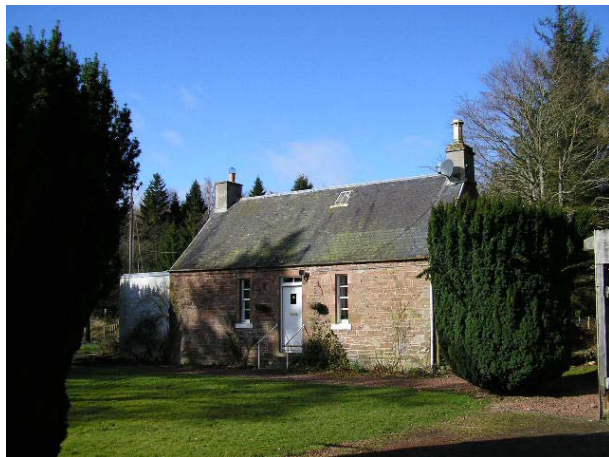
Figure 14: Weens Cottage, Borders Red sandstone & brick Four measurement locations Wall thickness: 400mm External face: rubble (x3) and cement (x1) Internal face: hard plastered
