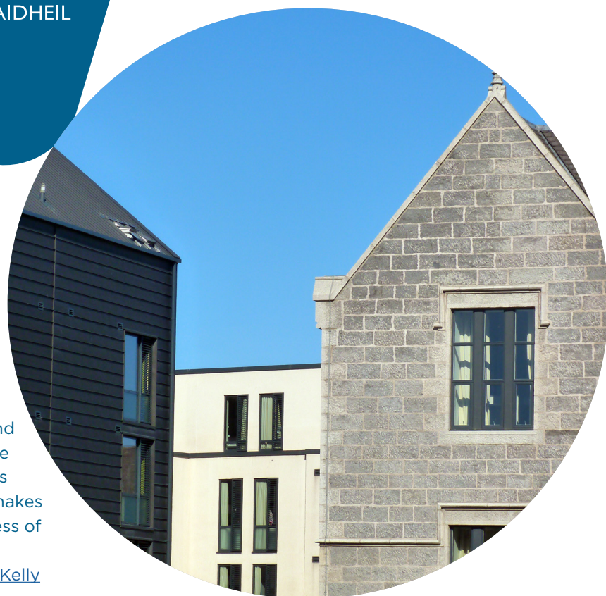
View of the converted school with the new additional elements © Aberdeen City Council
