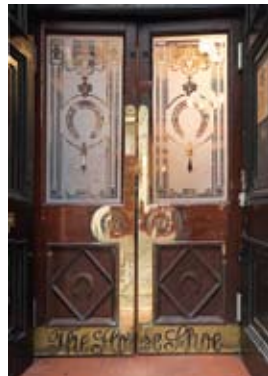
Lobby doors at, the Horseshoe
