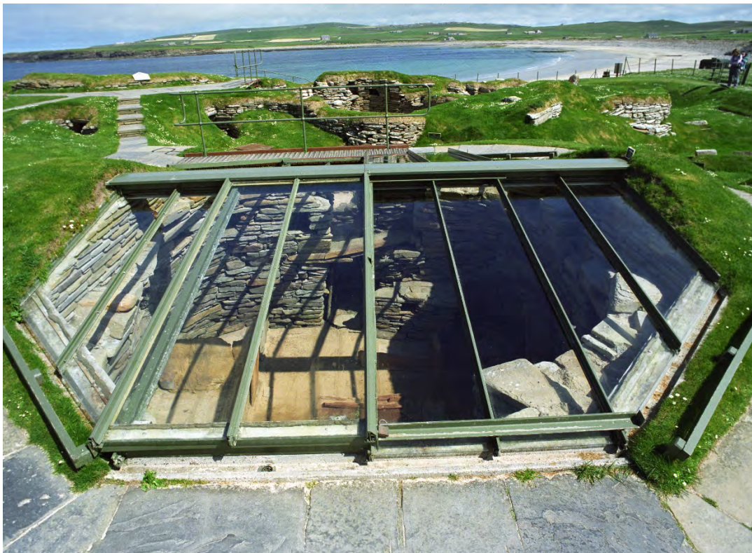
Figure 12: House 7 with its glass roof. In 2007 it was replaced with a turf roof which created a more benign environment. © Crown Copyright HES.
