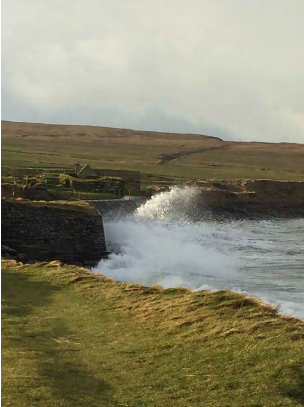
Figure 6: Waves crashing against the sea wall, showing the vulnerability of Skara Brae structures to storm damage. © Historic Environment Scotland.
